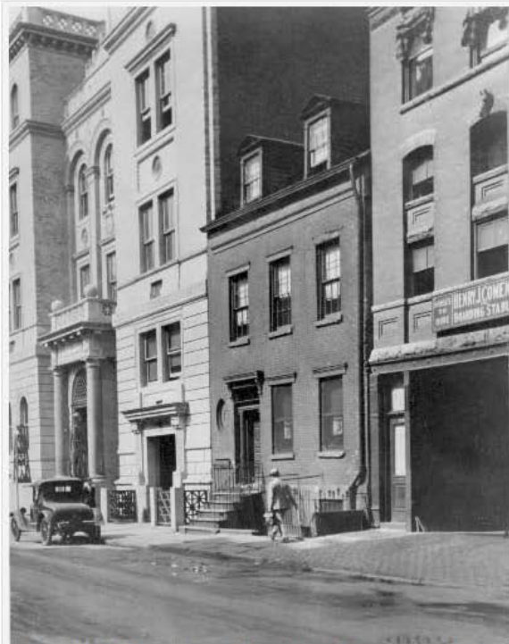
An old photograph can help you find out more about the history of your building.
