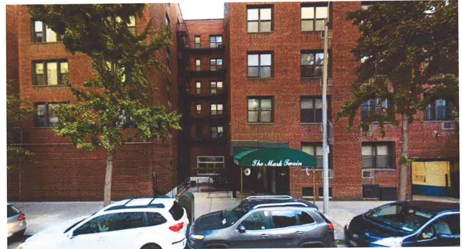
CURRENT PHOTO - FULL FAÇADE
