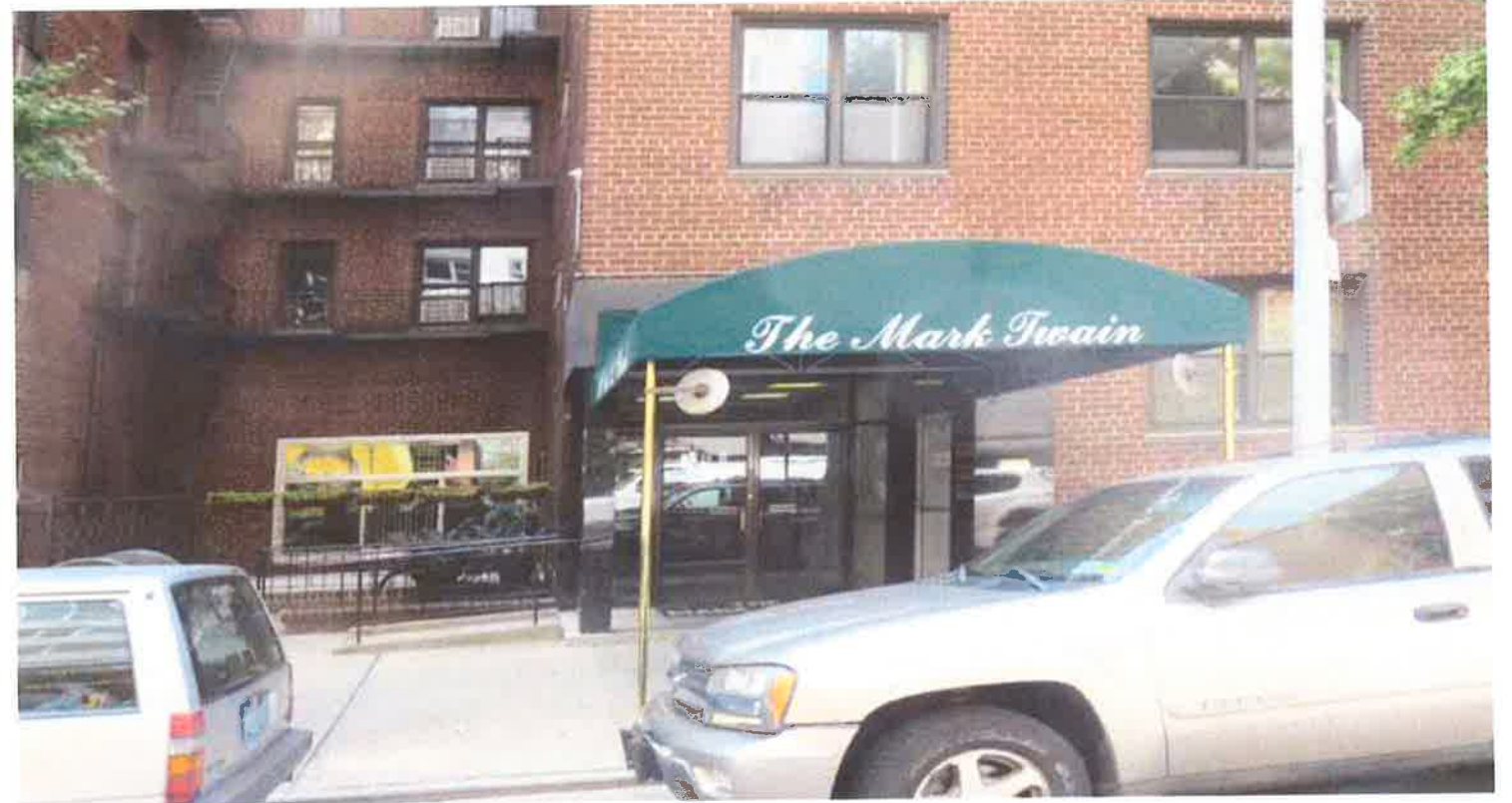
CURRENT PHOTO - AREA OF WORK
