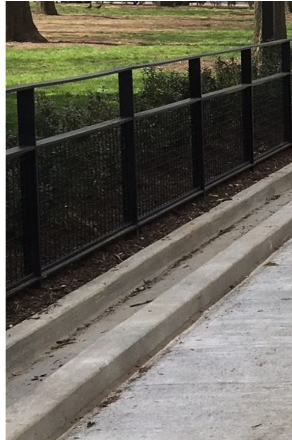
EXISTING FENCE AT BLEECKER STREET
