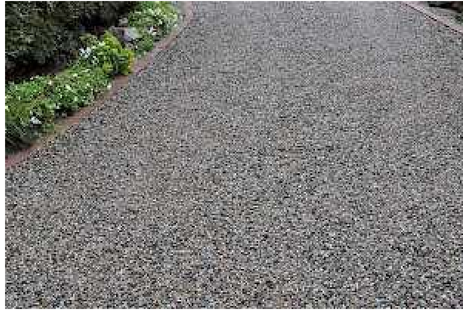
COMPACTED STONE DUST
