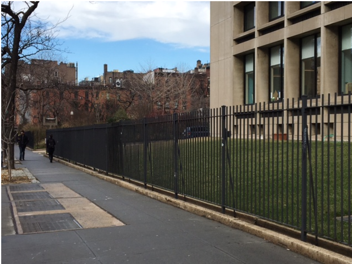
2. WEST VIEW OF SILVER TOWERS 1 FENCE ALONG HOUSTON STREET
