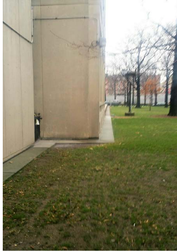
1. WEST VIEW OF OAK GROVE ALONG SILVER TOWERS
