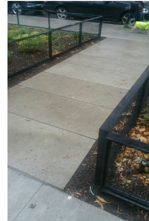
EXISTING CONCRETE PATH AT BLEECKER STREET
