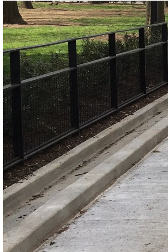
EXISTING FENCE AND GUTTER AT BLEECKER STREET
