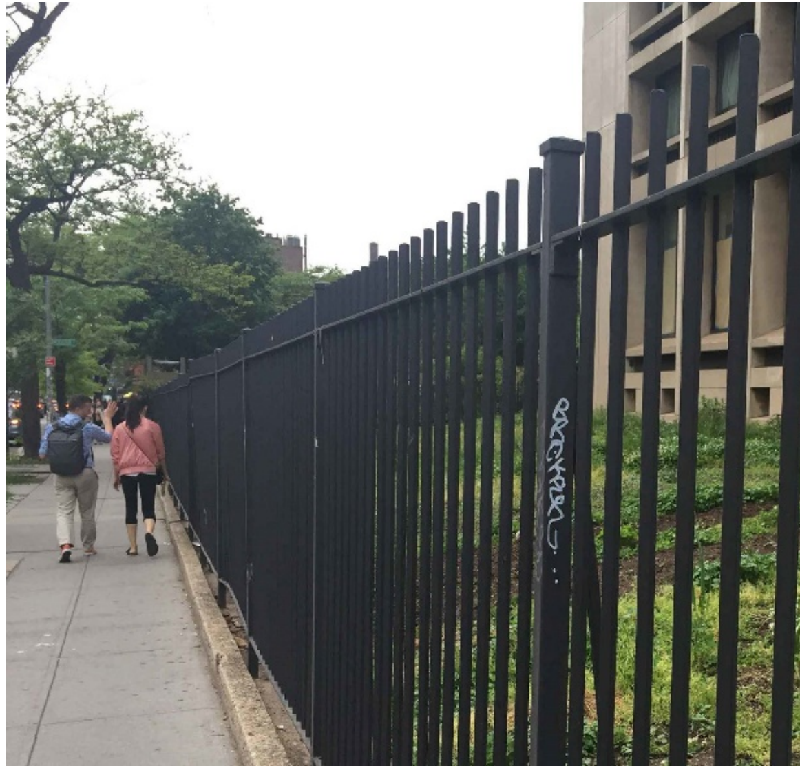
EXISTING WEST VIEW FENCE ON HOUSTON STREET
