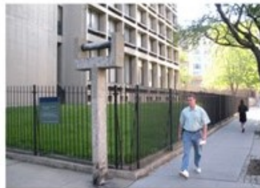
EXISTING SILVER TOWERS 1 FENCE AND GUTTER
