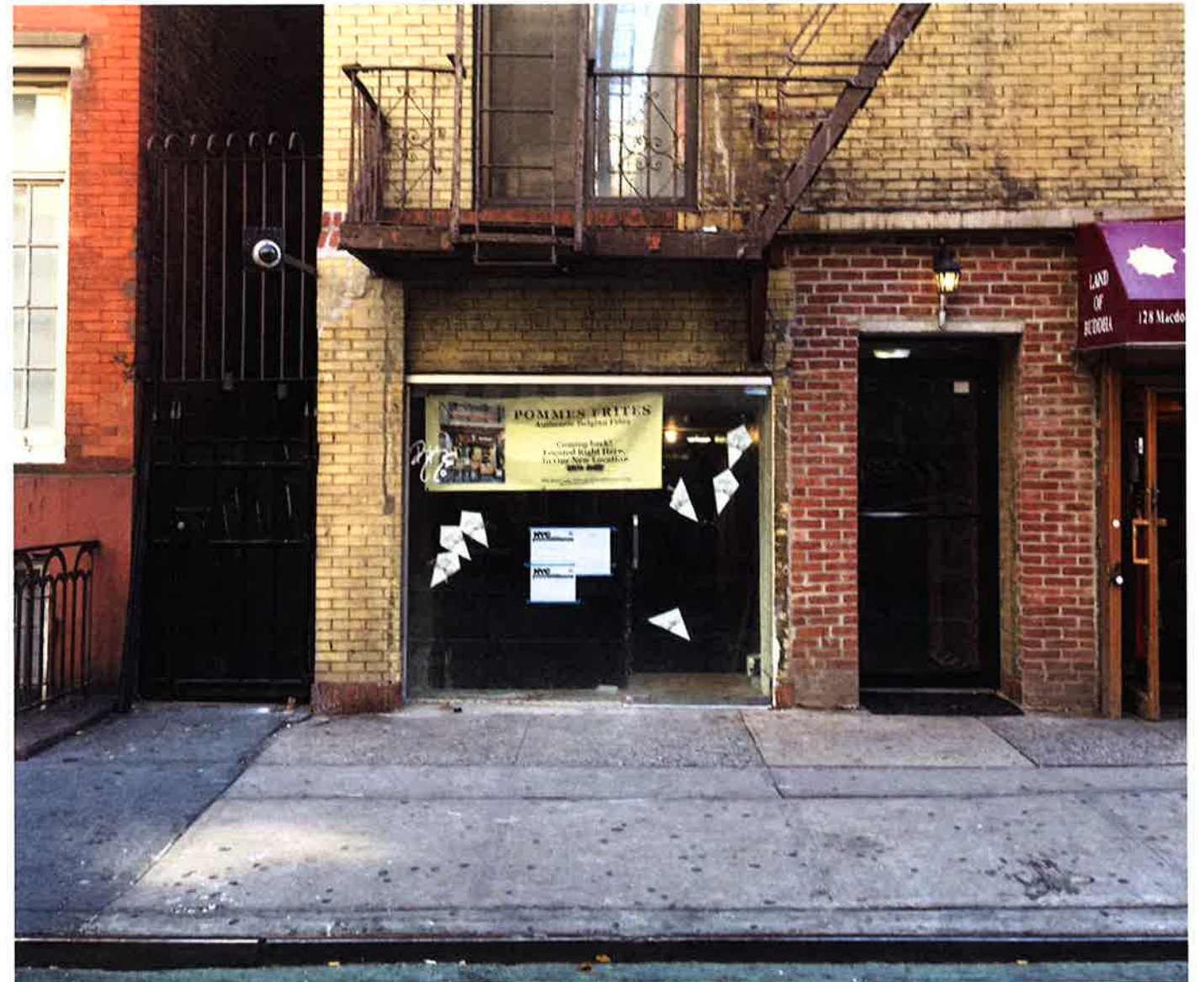
EXISTING STOREFRONT FACADE
