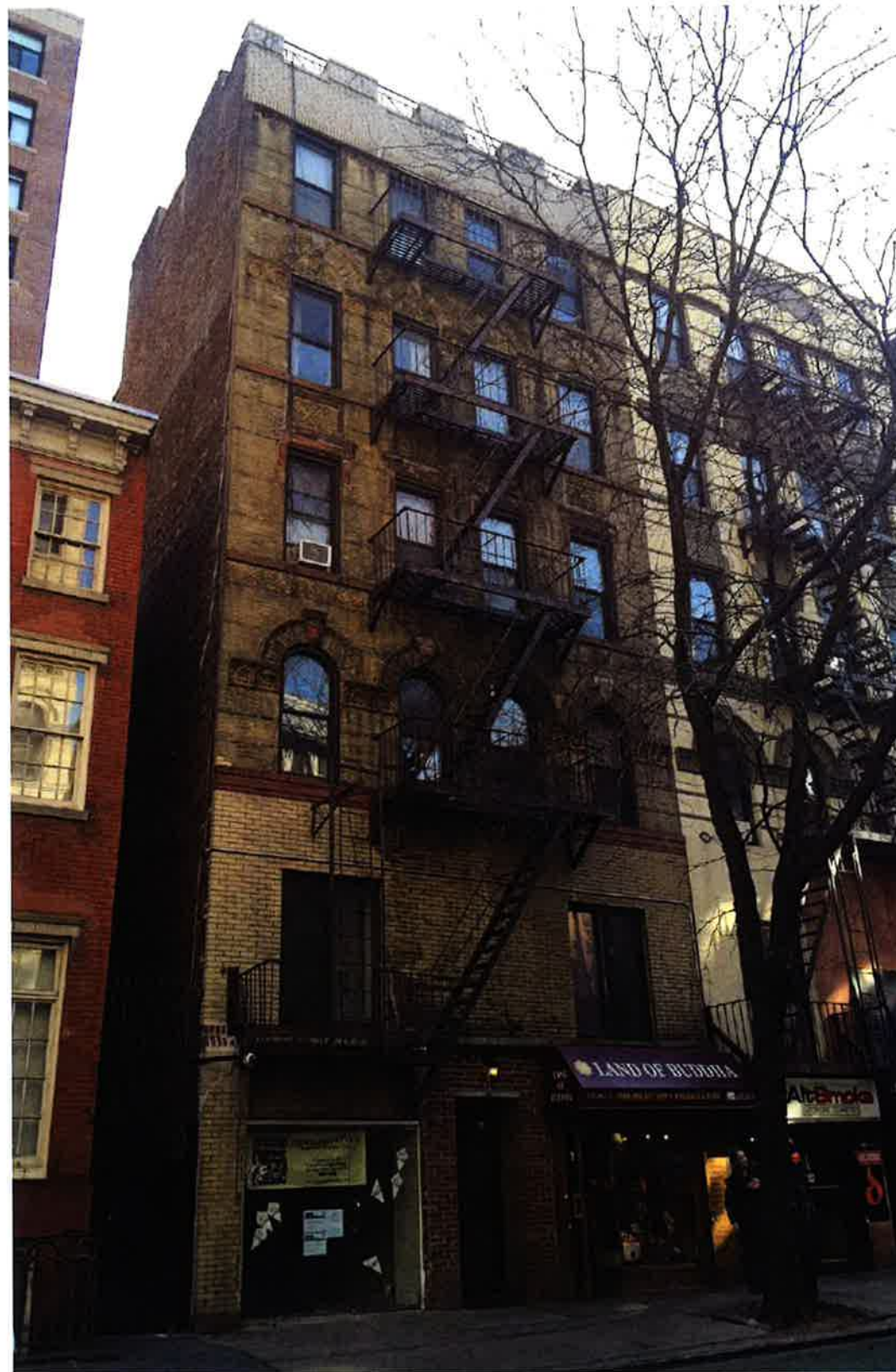
EXISTING FACADE - LOOKING SOUTH-EAST
