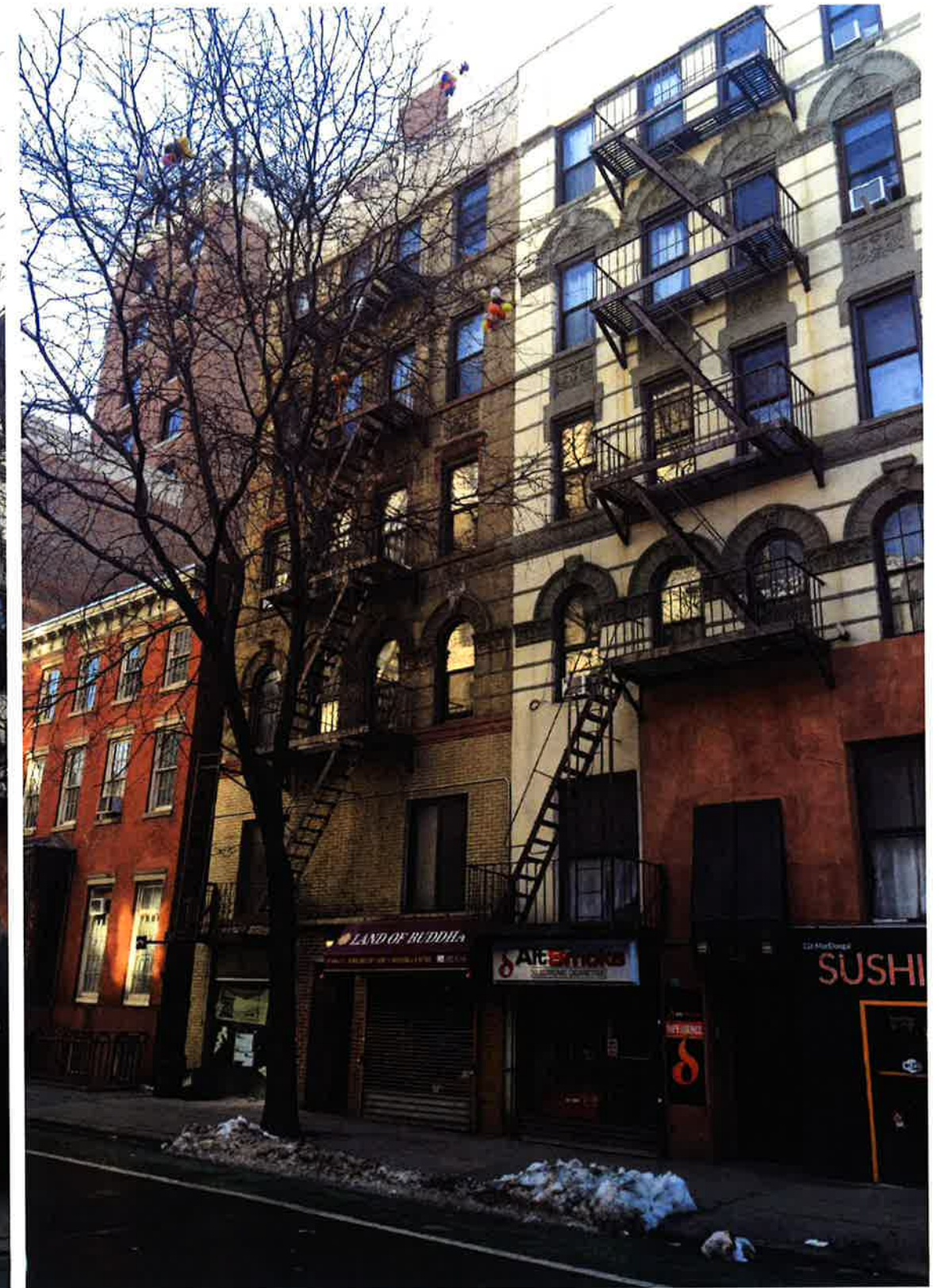
EXISTING FACADE - LOOKING NORTH-EAST
