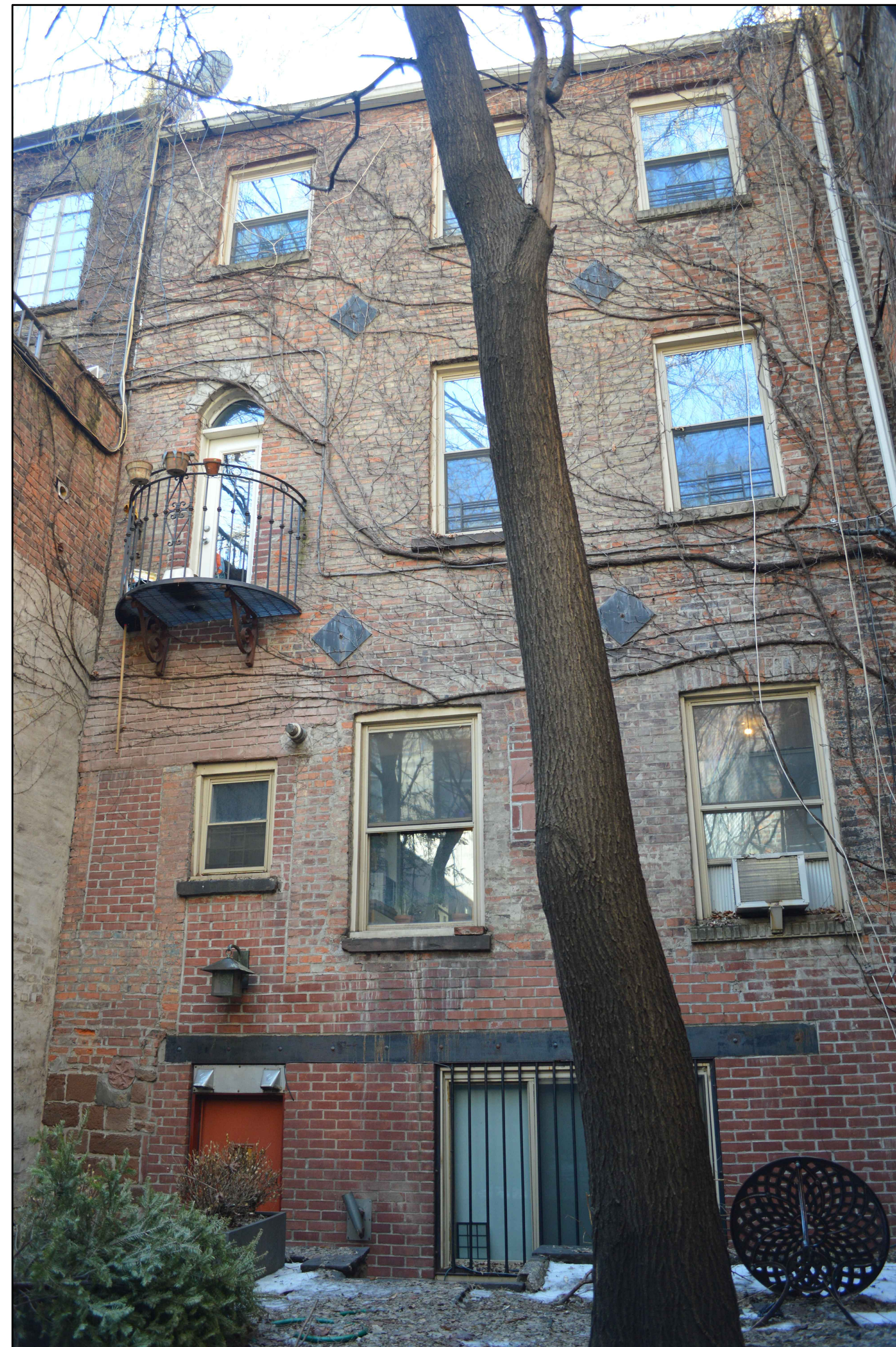
13 Bleecker Street - Rear Facade
