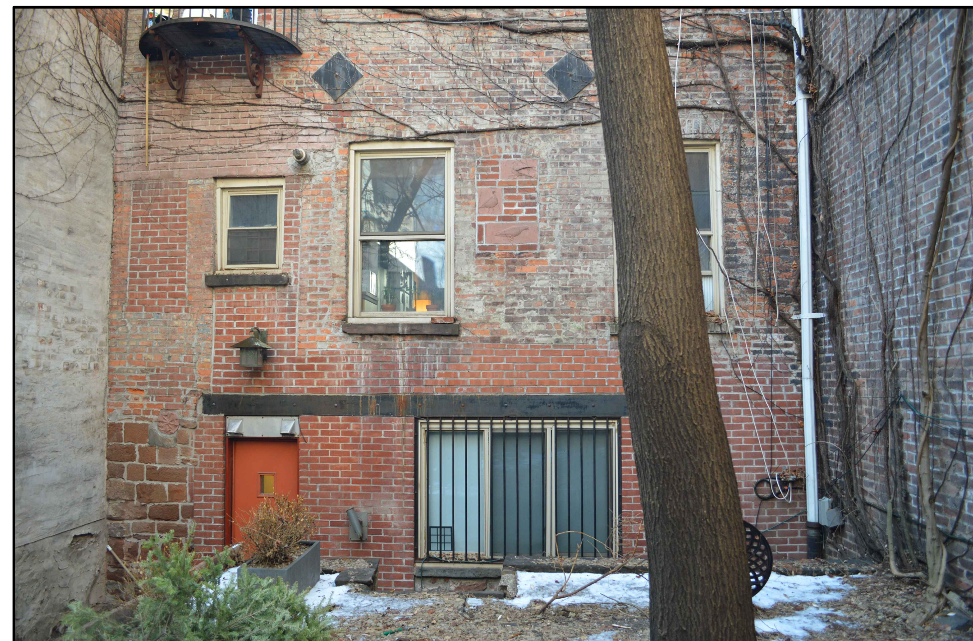
13 Bleecker Street - Rear Facade
