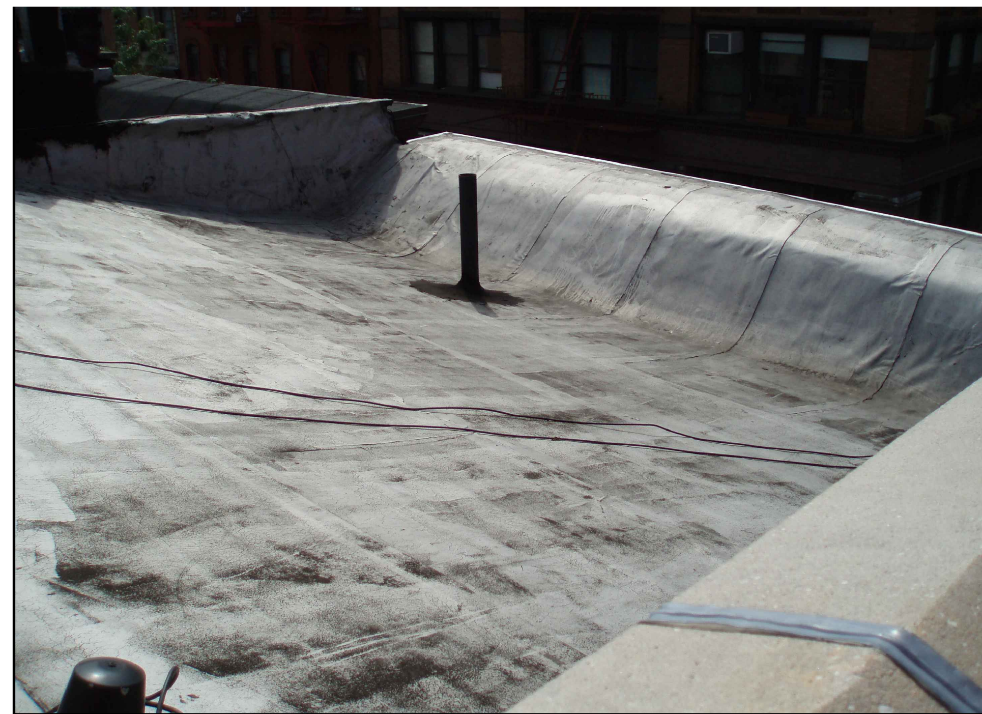
13 Bleecker Street - Roof Photograph
