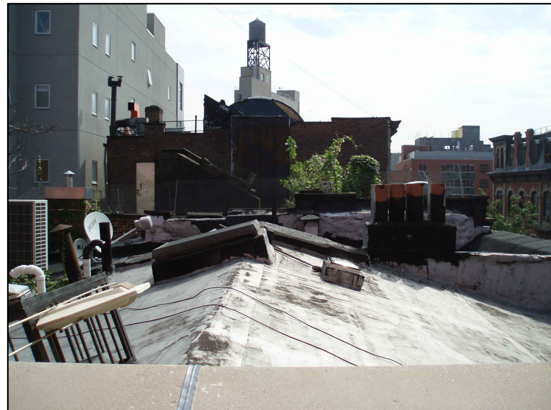
13 Bleecker Street - Roof Photograph
