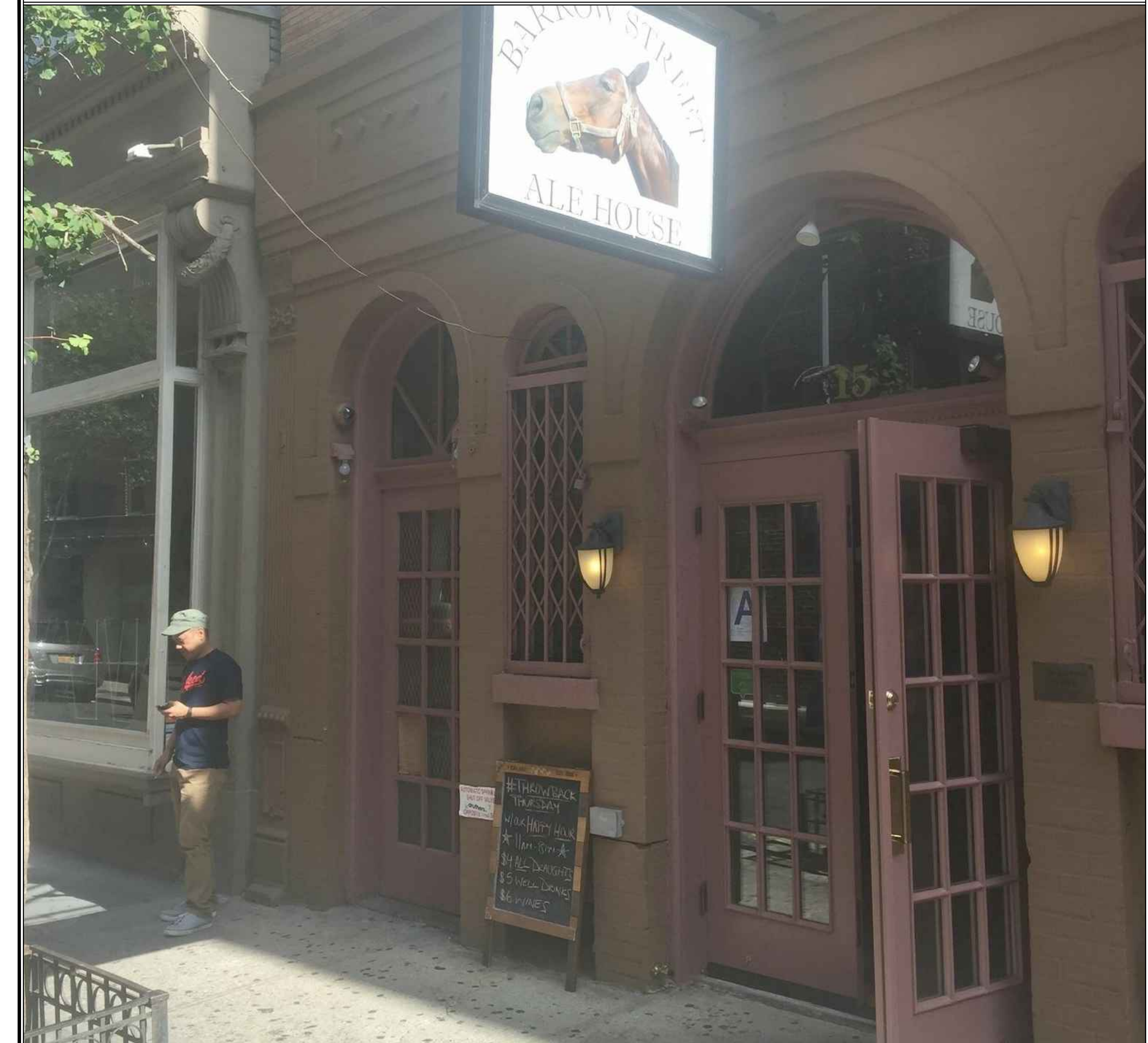
EXISTING FACADE CONDITIONS
