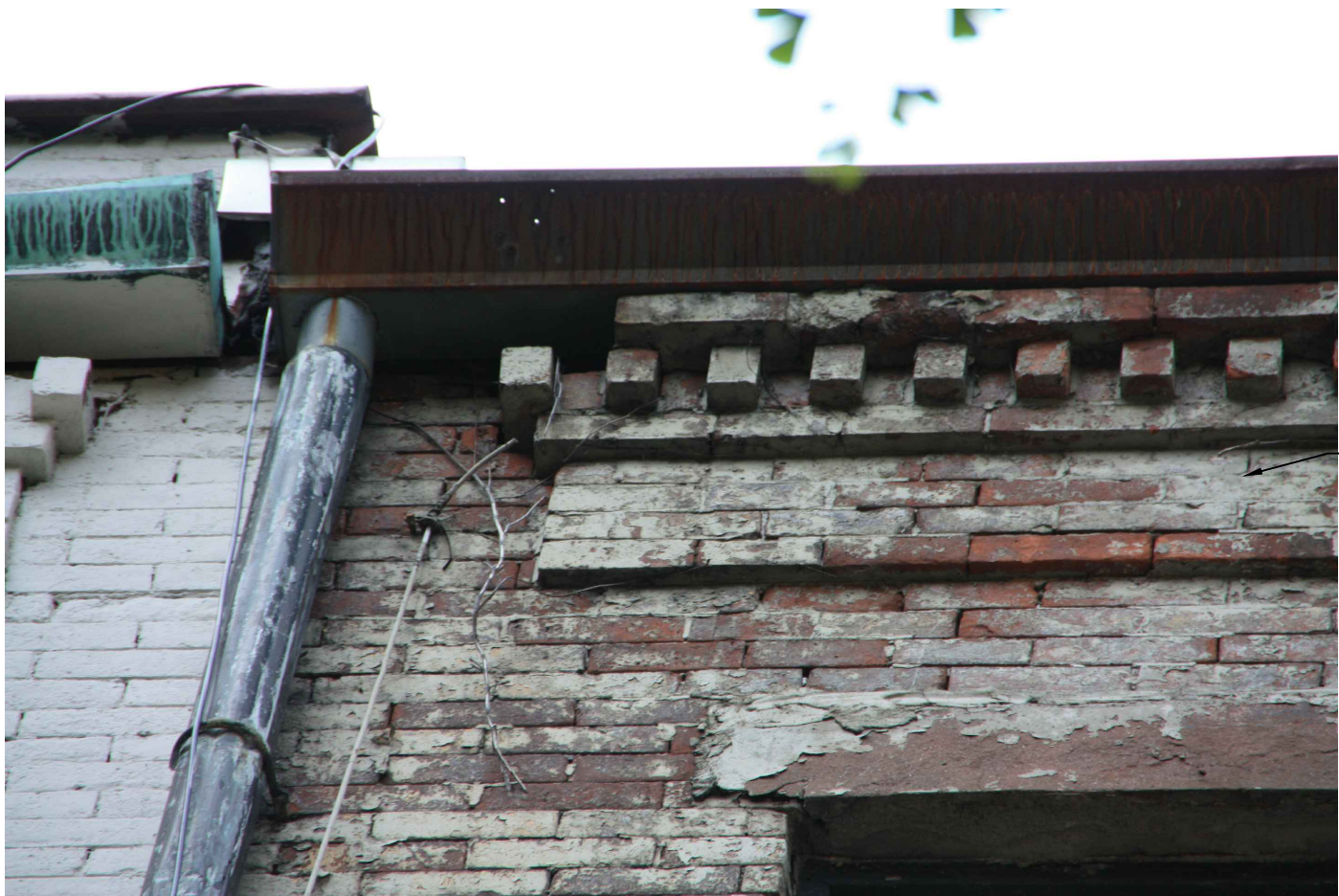
EXISTING BRICK CORNICE TO REMAIN. REPOINT AND PATCH TO MATCH W/ EXISTING IN BOND, TYPE AND COLOR.
