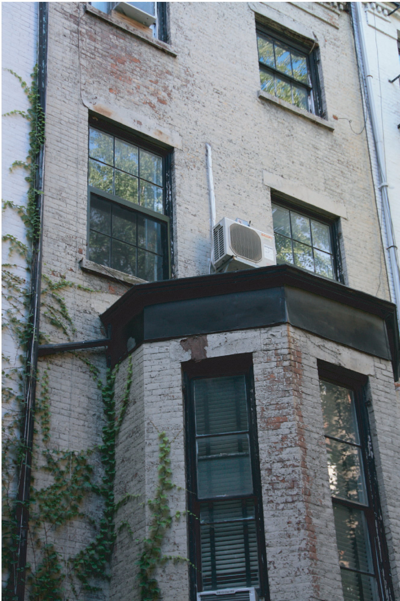
4. EXISTING MASONRY IN POOR CONDITION
