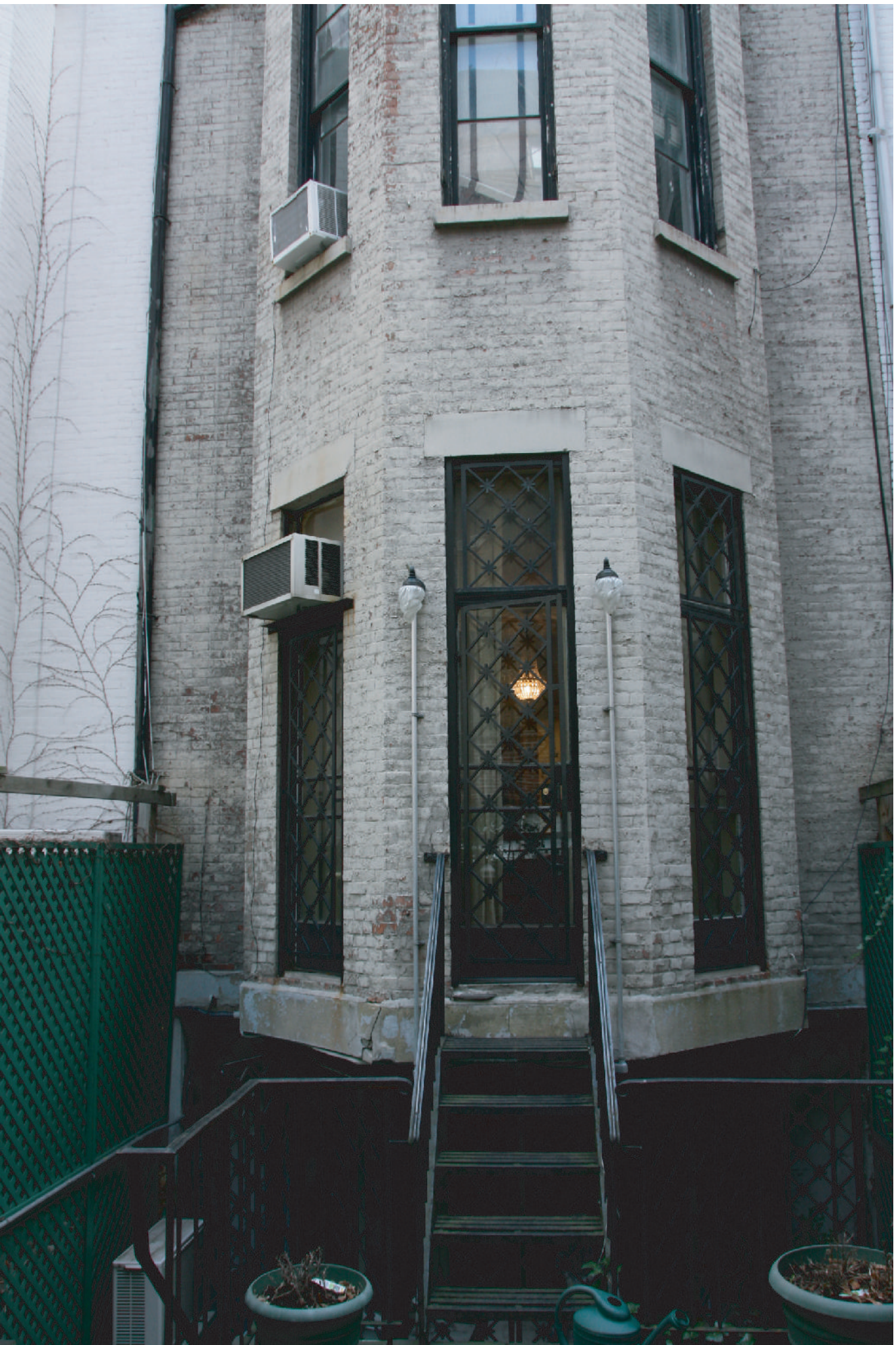
6. REAR EXTENSION- BRICK MASONRY IN POOR CONDITION
