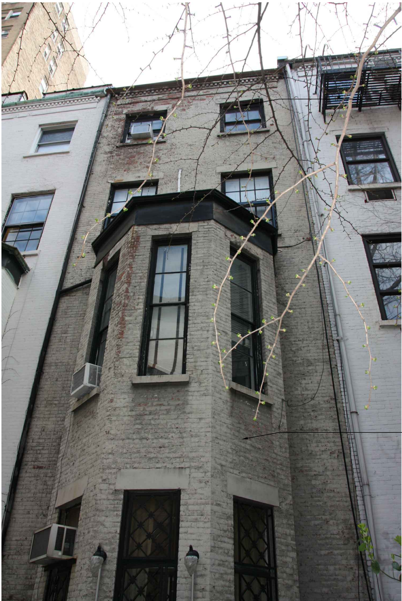
EXISTING WINDOWS AT 3RD AND 4TH FLRS TO BE REPLACED W/ NEW TO MATCH W/ EXISTING.
