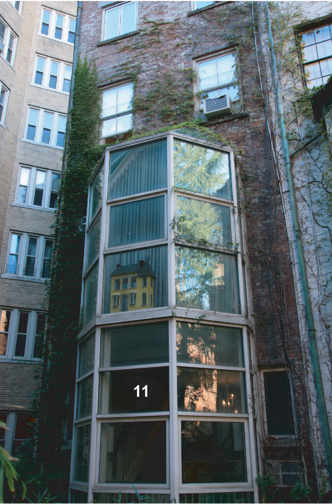
6. REAR EXTENSION- BRICK MASONRY IN POOR CONDITION
