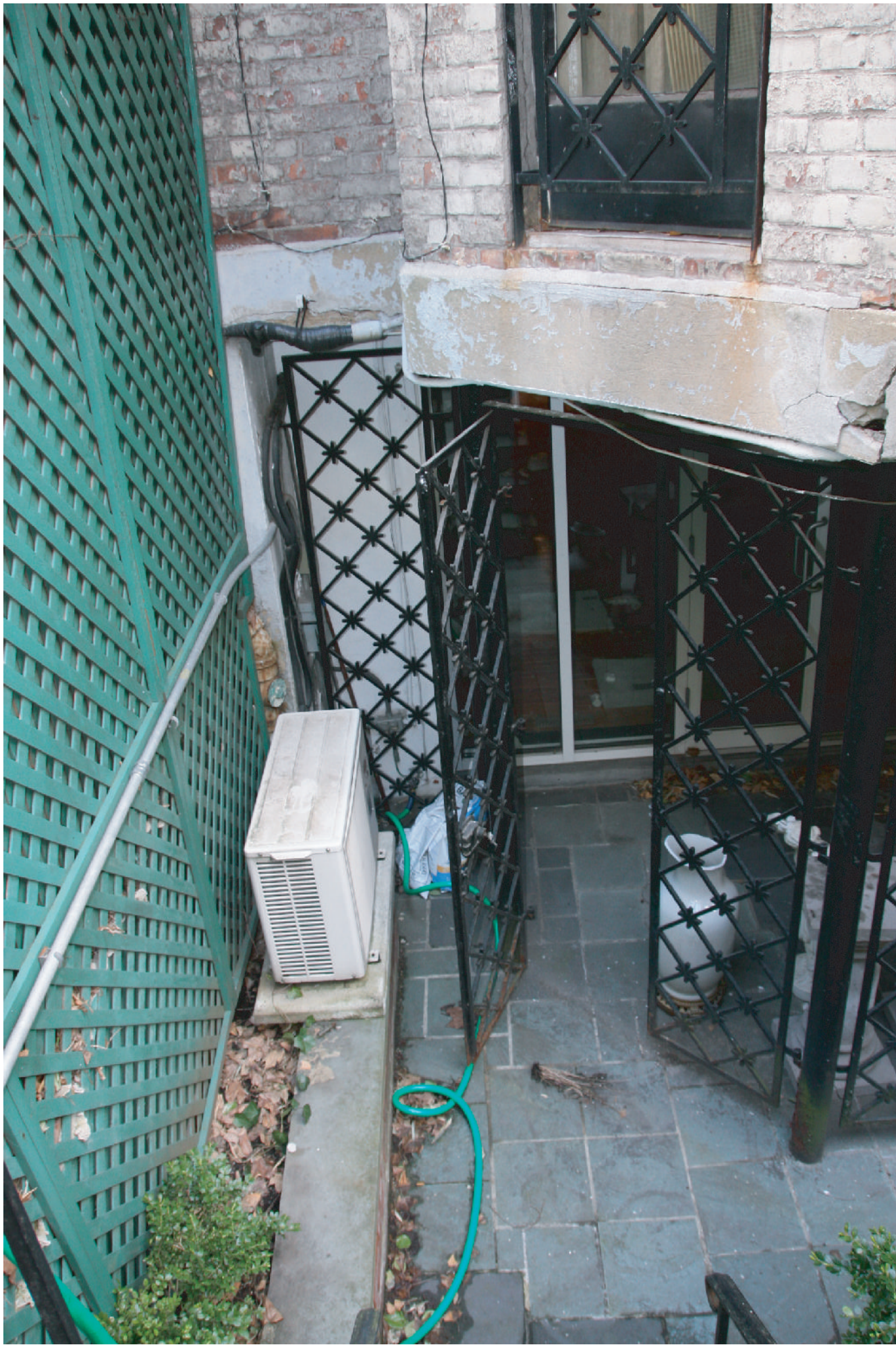
5. REAR YARD CELLAR LEVEL MASONRY DETIORATION AT LINTEL
