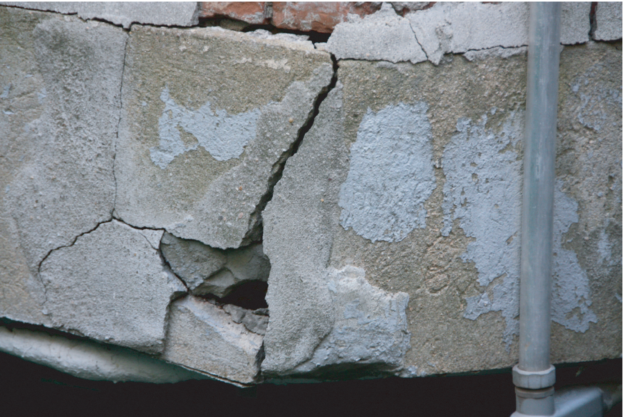
1. SPALLING AT IRON LINTEL AND COLUMN CONNECTION
