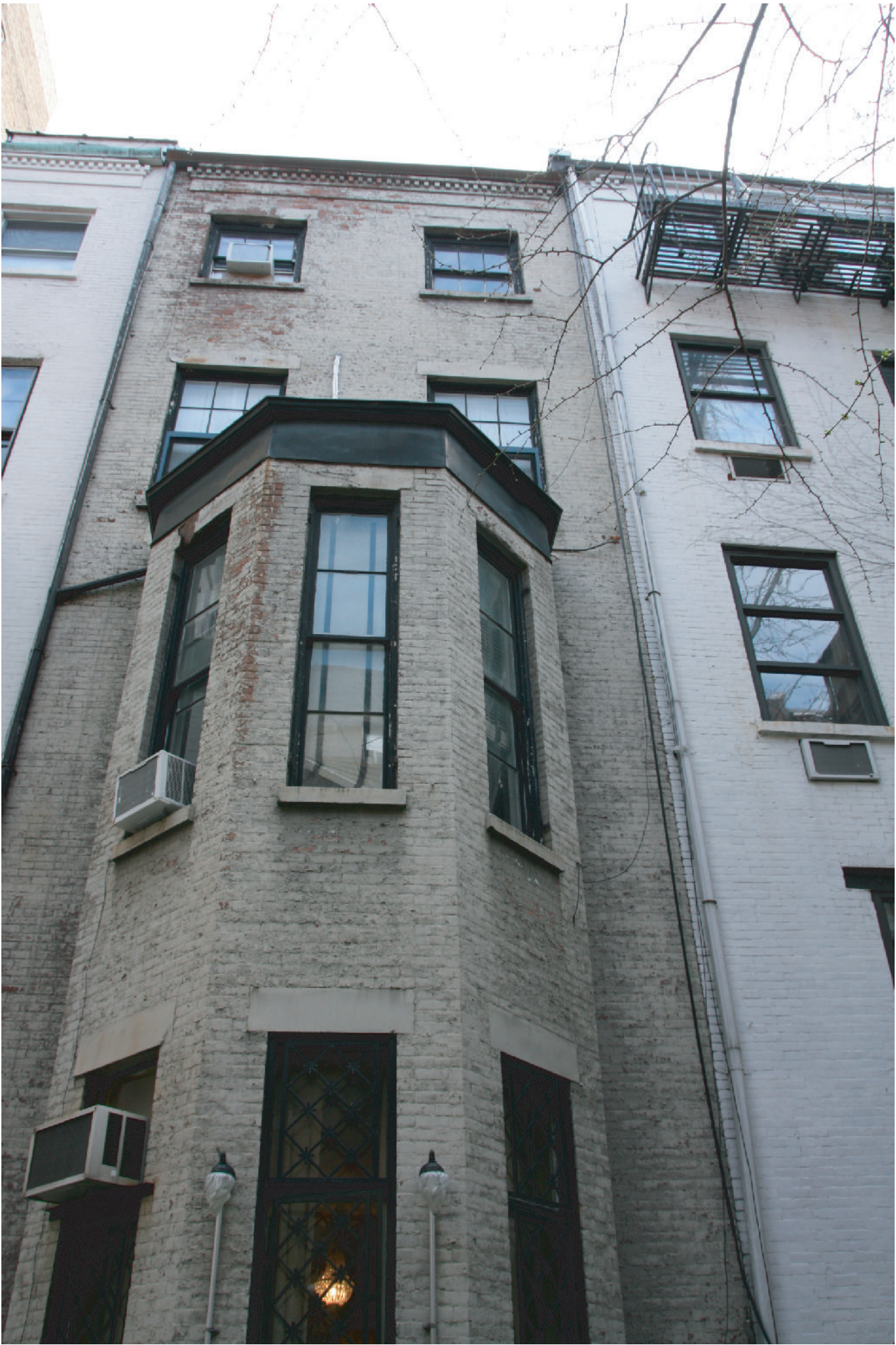
7. REAR EXTENSION- BRICK MASONRY IN POOR CONDITION
