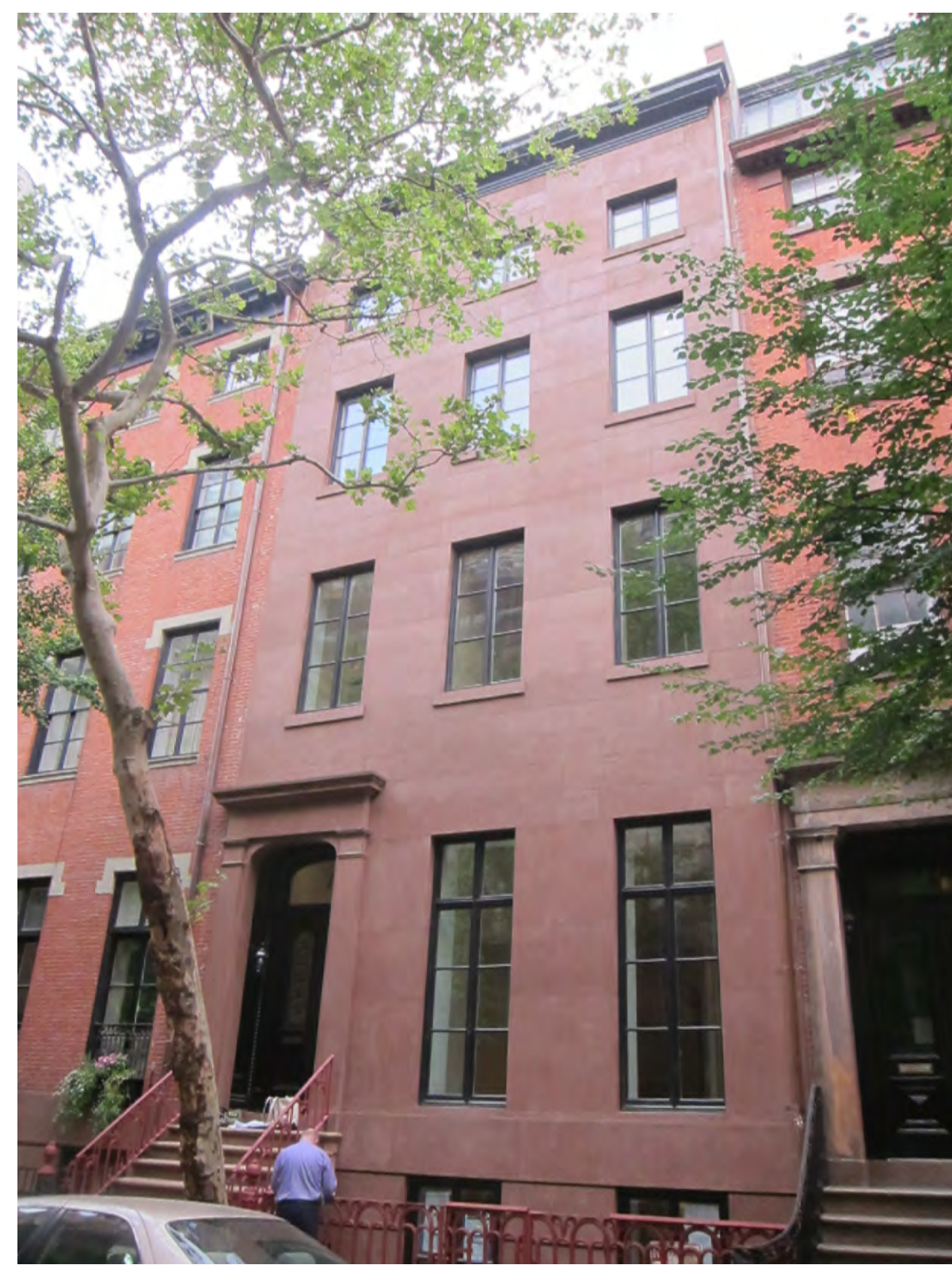
3 16 E. 10th ST - FRONT FACADE NTS
