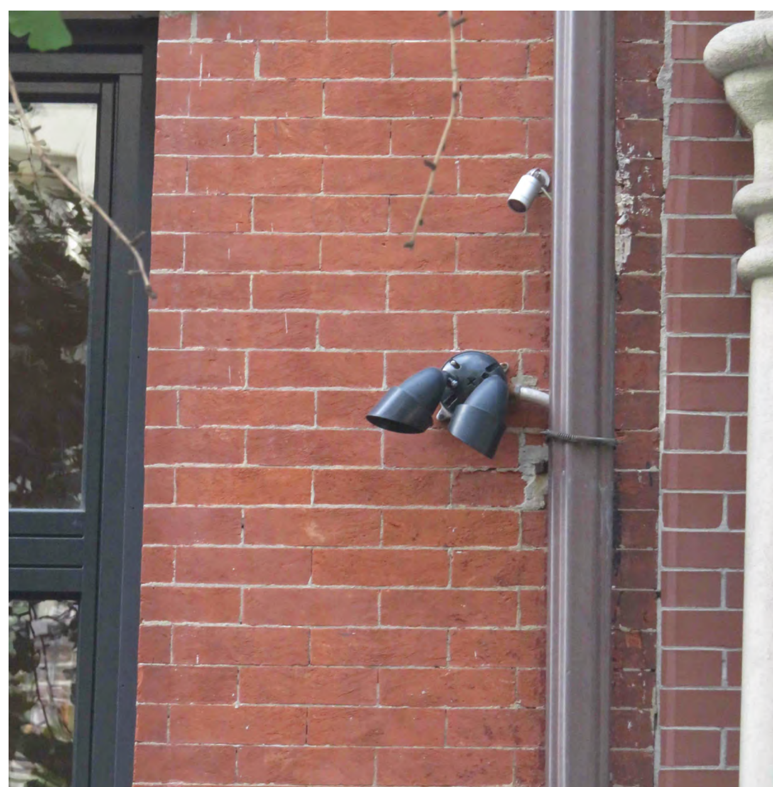
6 NEIGHBOR'S FACADE showing security cameras NTS
