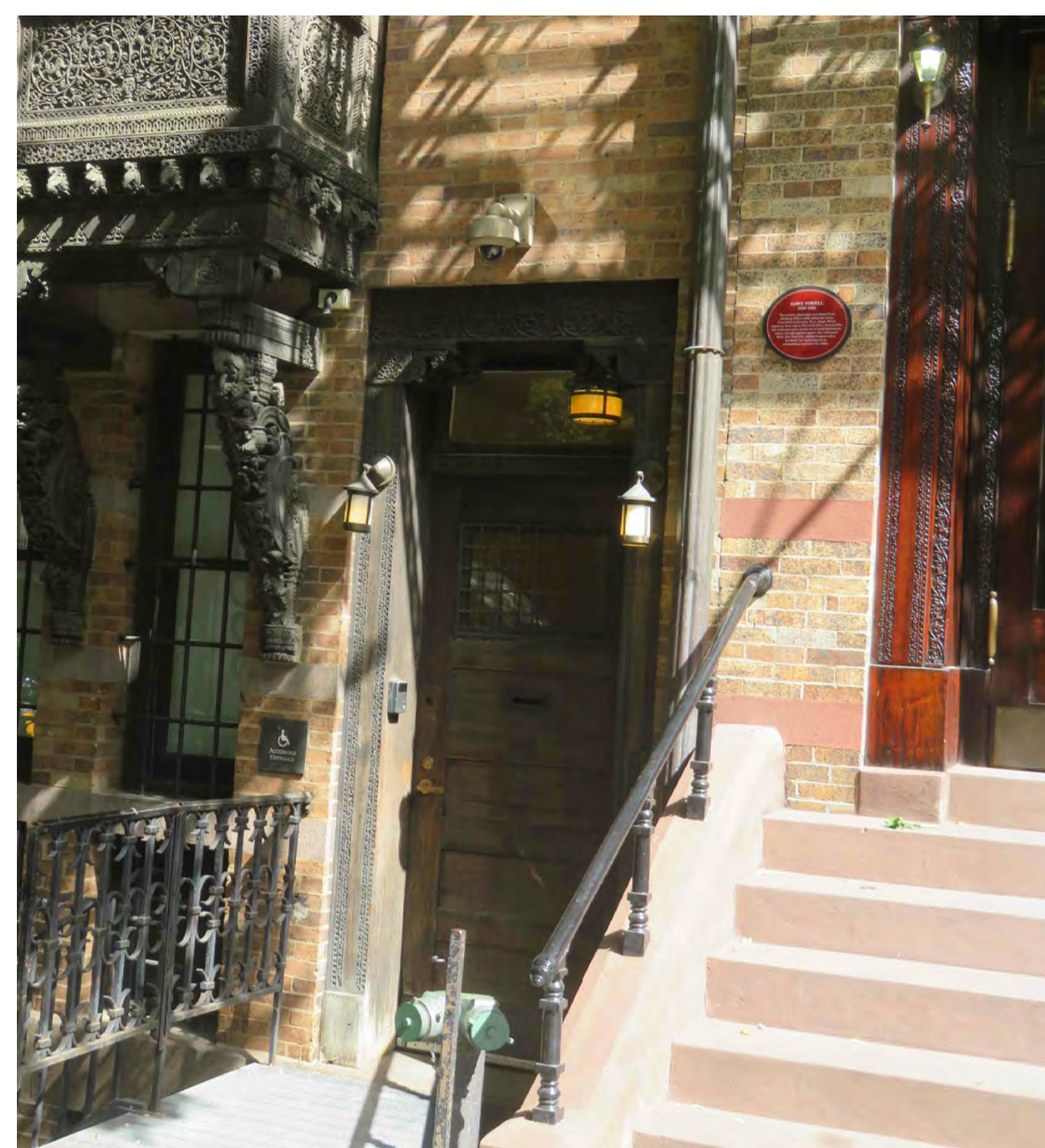
7 NEIGHBOR'S FACADE showing security cameras NTS
