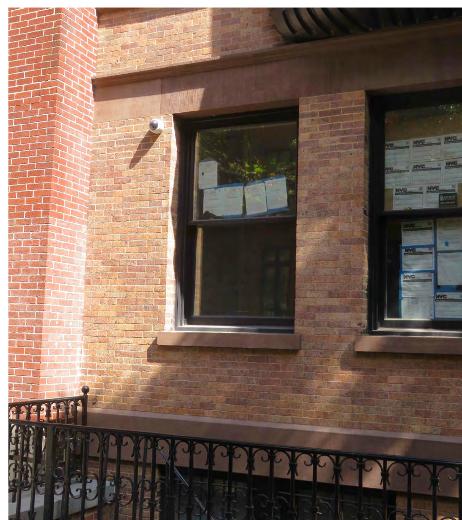
9 NEIGHBOR'S FACADE showing security cameras NTS
