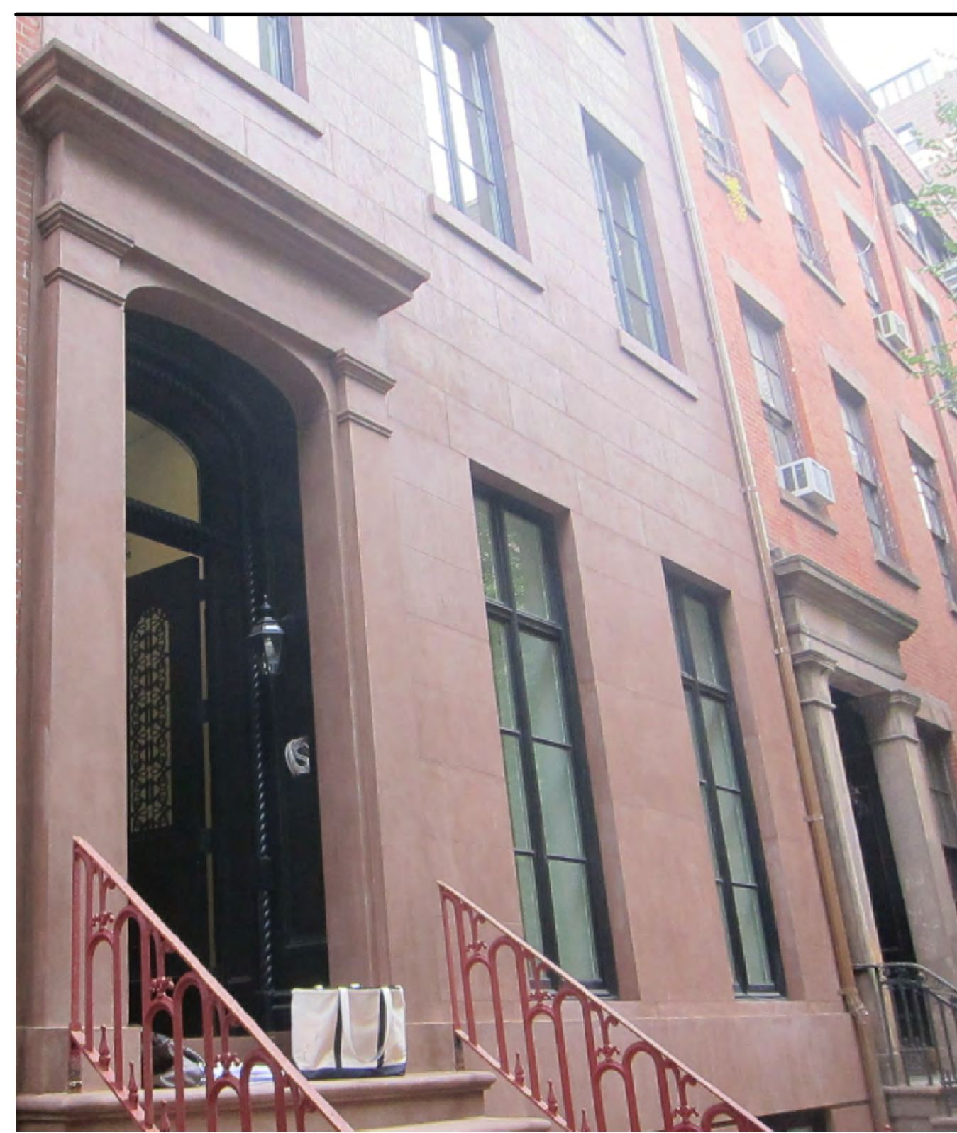
4 16 E. 10th ST - FRONT FACADE NTS
