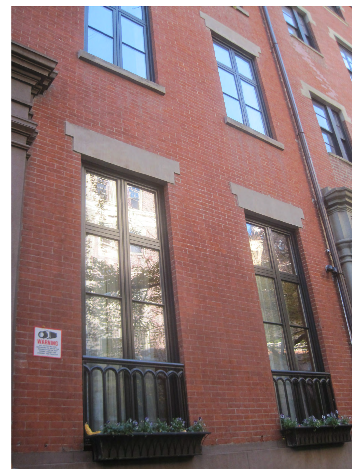
5 NEIGHBOR'S FACADE showing security cameras NTS
