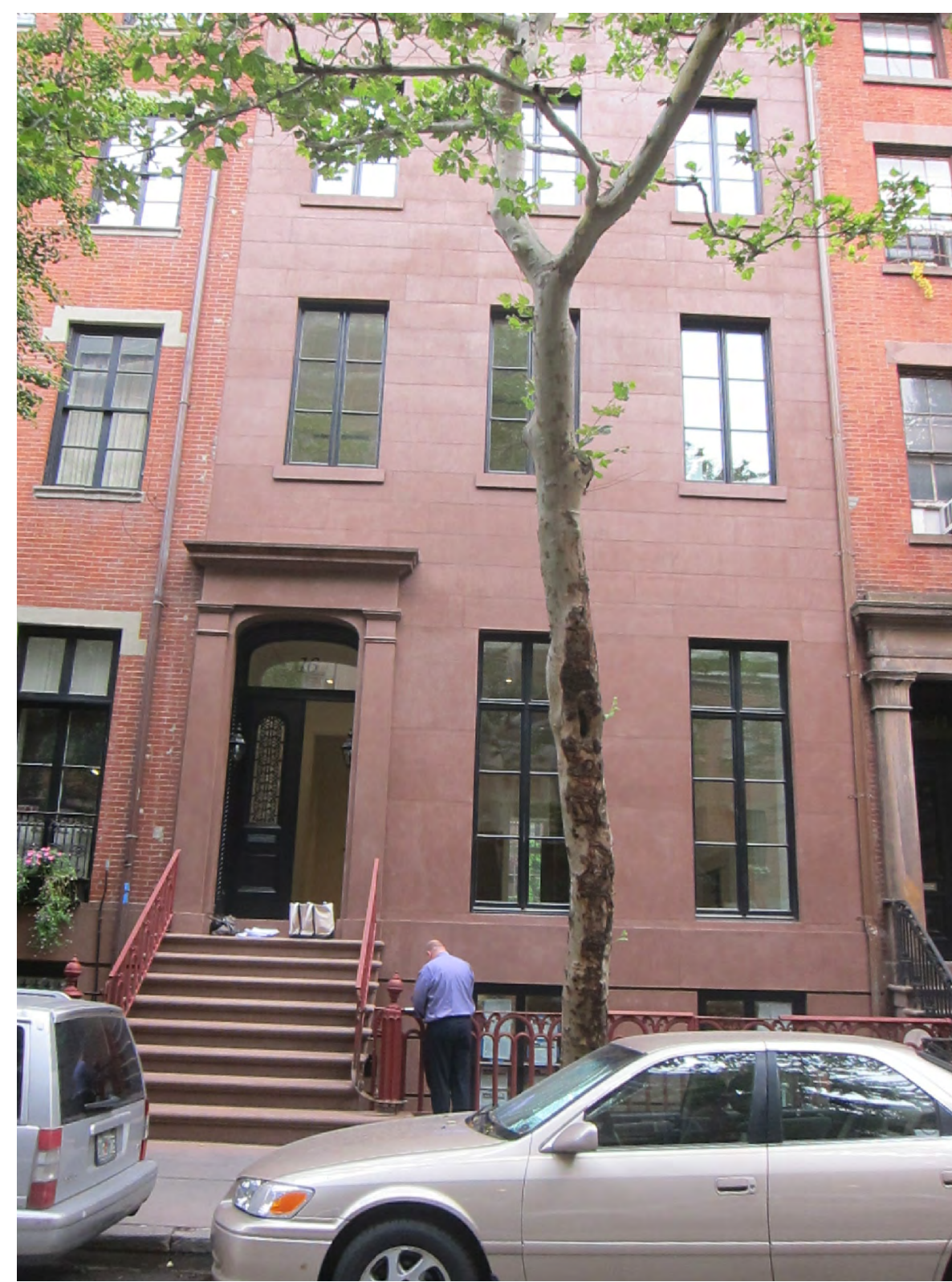
2 16 E. 10th ST - FRONT FACADE NTS
