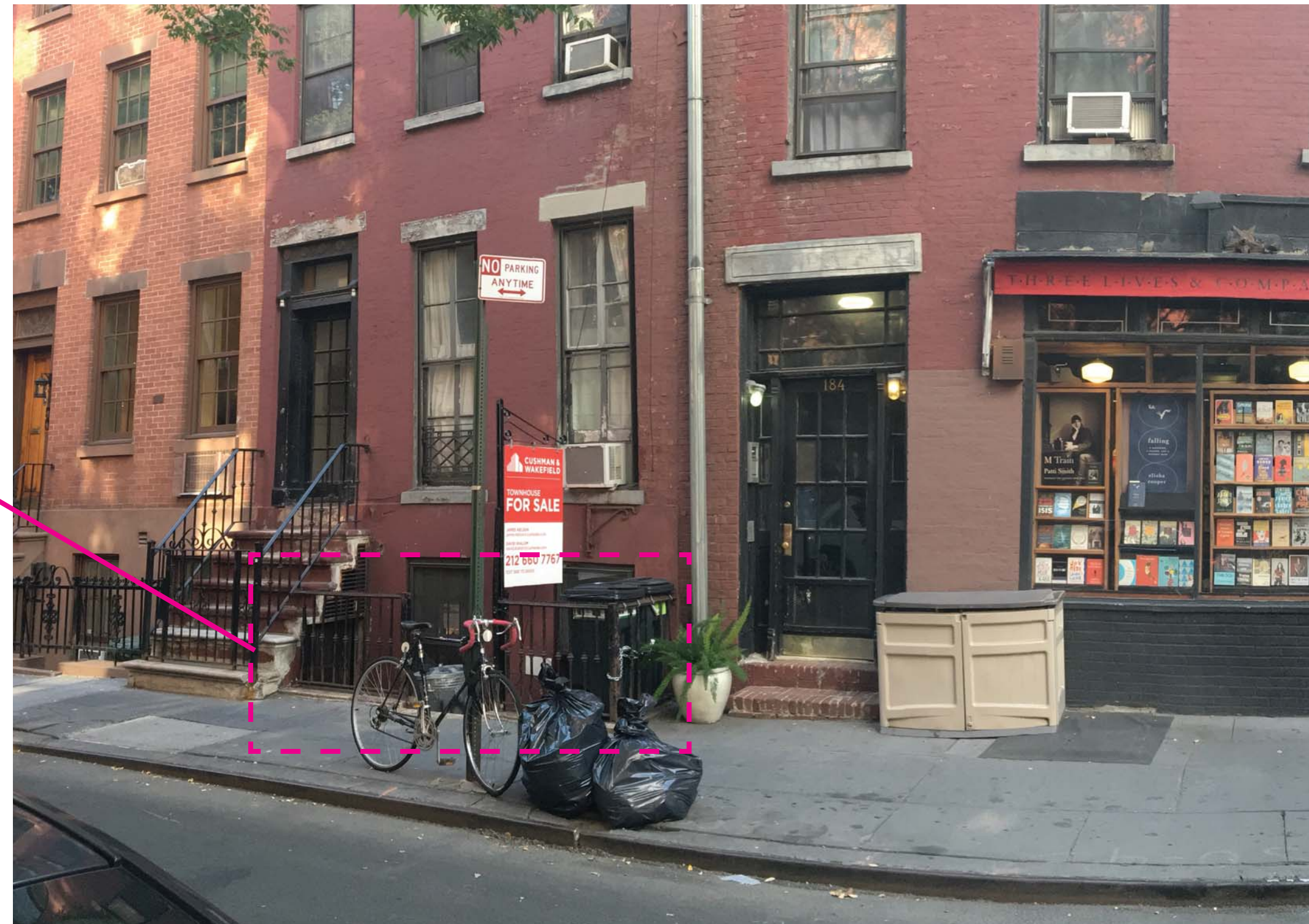
RAILING AT 182 WAVERLY PLACE (SQUARE COLLARS & RODS)
