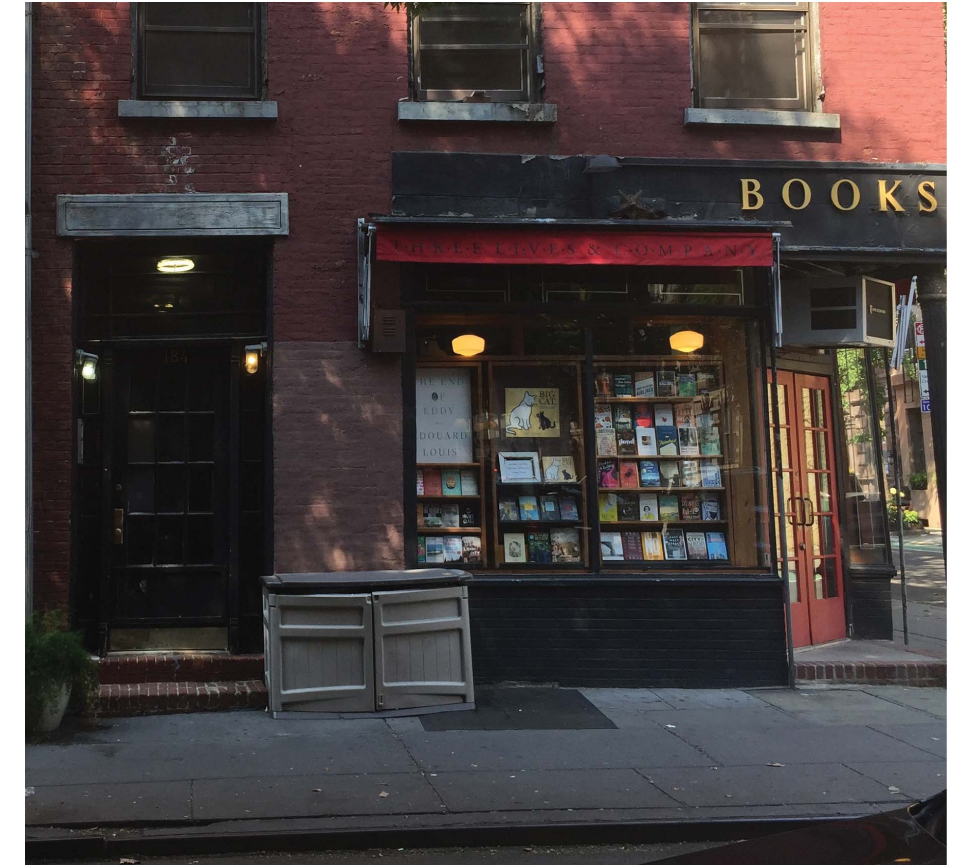
3. PHOTO OF EXISTING CONDITION
