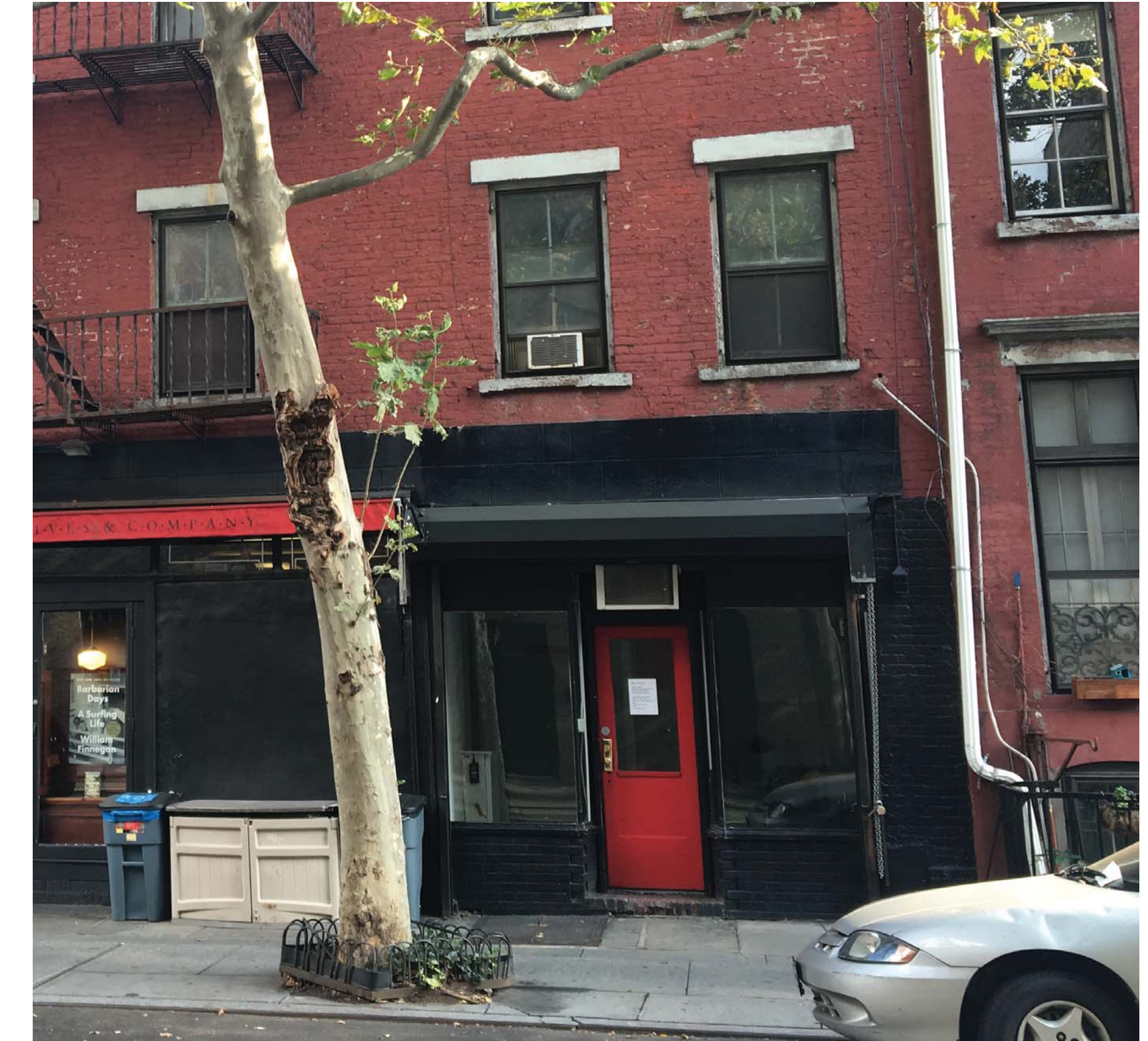
3. PHOTO OF EXISTING CONDITION
