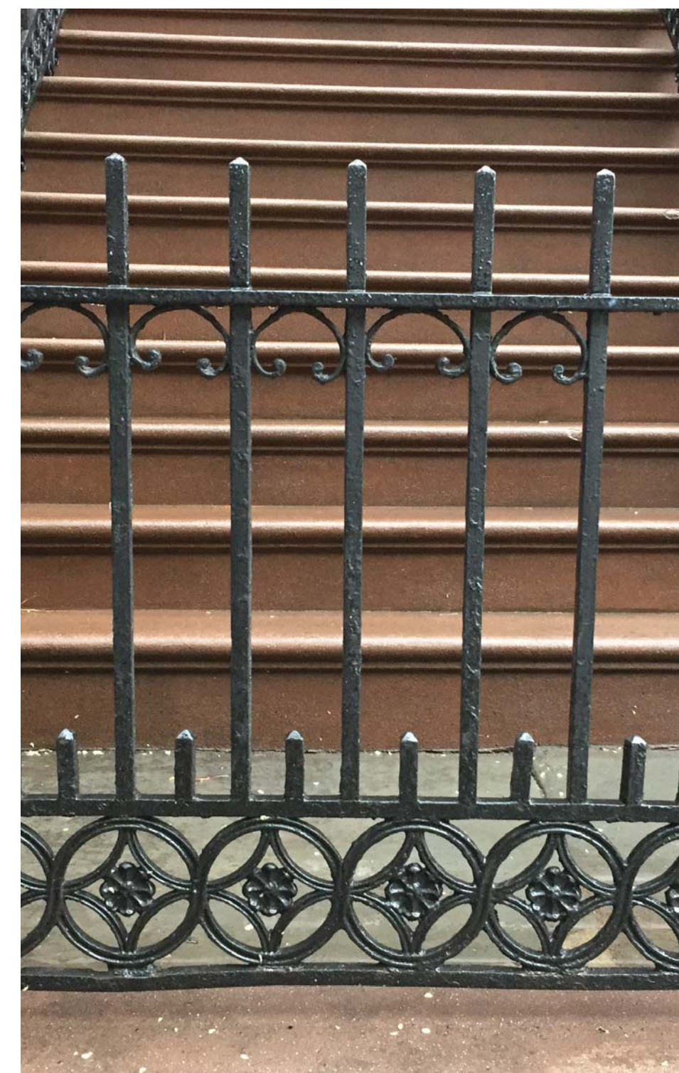
PRECEDENT RAILING AT W.12 ST.
