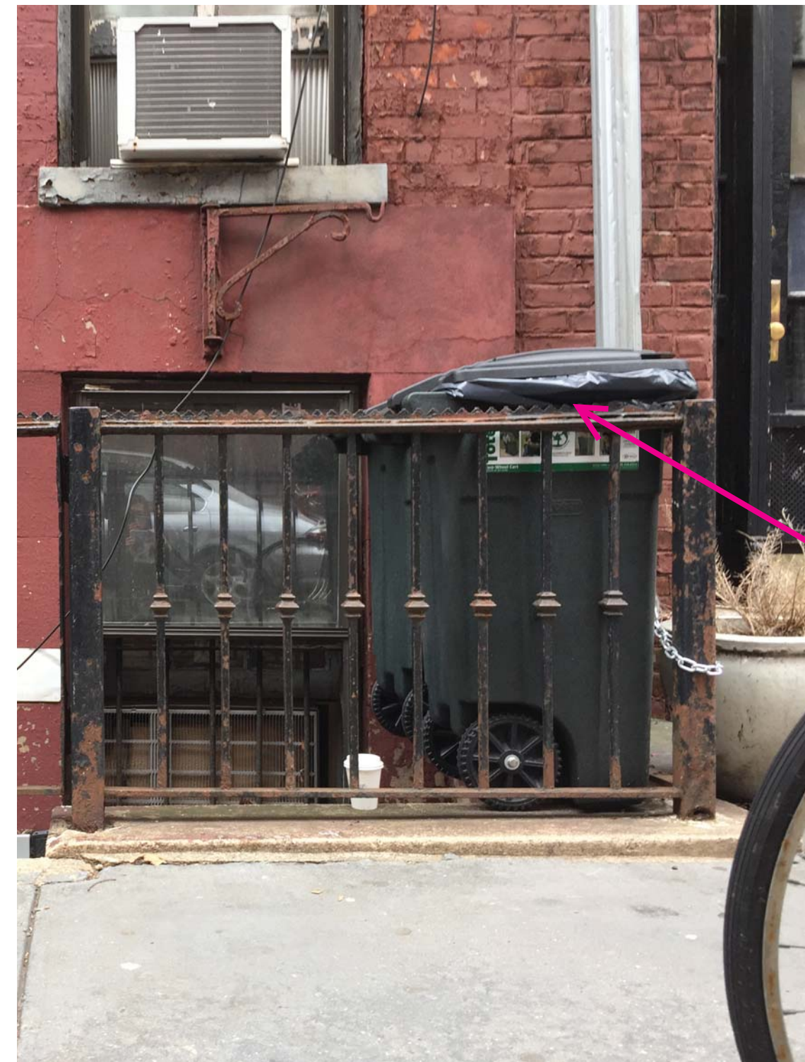
RAILING AT 182 WAVERLY PLACE (SQUARE COLLARS & RODS)
