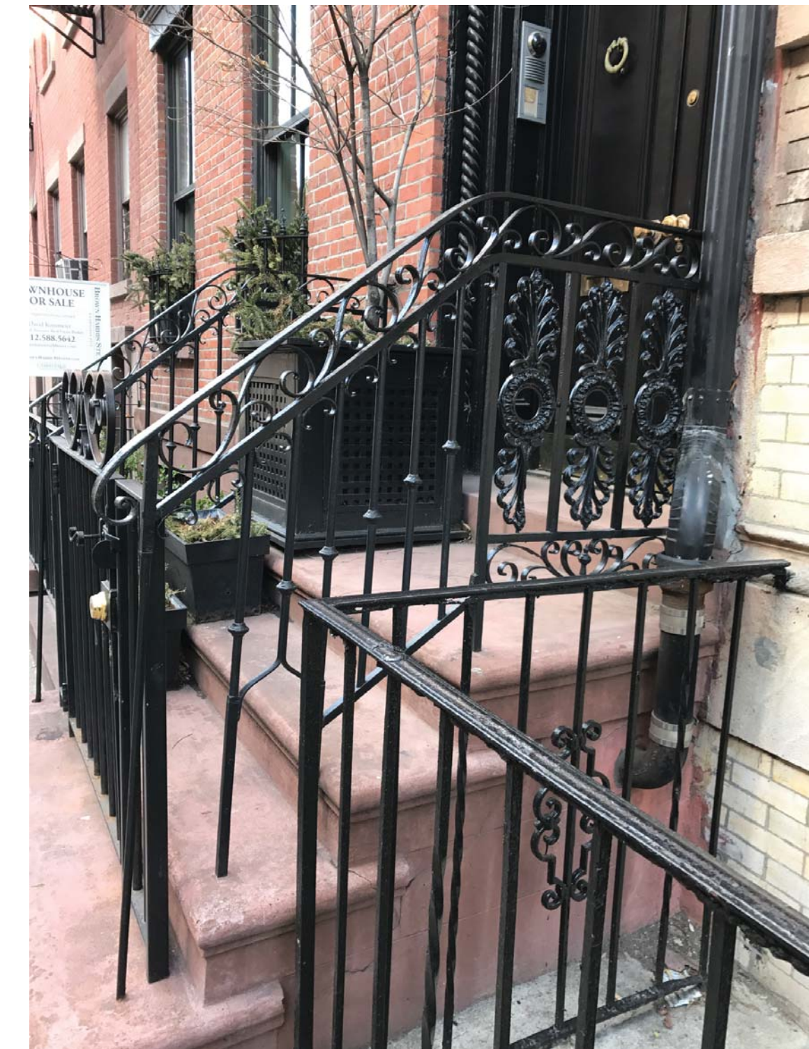
PRECEDENT RAILING AT 149W. 10TH ST. (SCROLL WORK)
