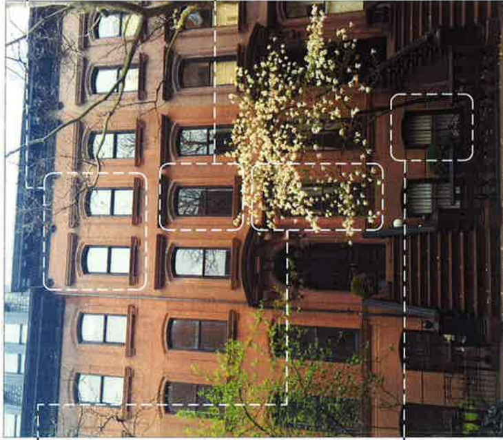
Window Head Condition: Straight Horizontal Top Rail at Upper Sash
