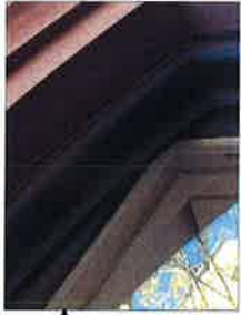
Window Head Condition: Straight Horizontal Top Rail at Upper Sash
