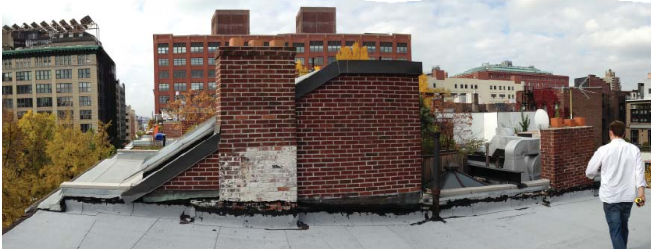
ROOF VIEW LOOKING WEST
