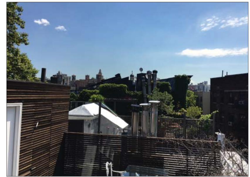
NEIGHBORING ROOFTOP ADDITIONS LOOKING EAST
