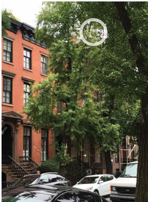
VIEW 3 ROOFTOP ADDITION NOT EXPECTED TO BE VISIBLE FLUE: SOME VISIBILITY EXPECTED
