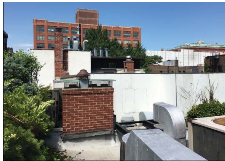
NEIGHBORING ROOFTOP ADDITIONS LOOKING WEST
