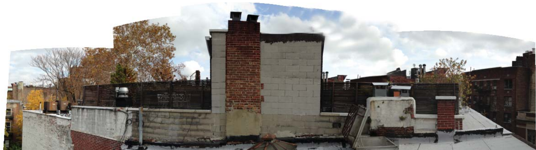
ROOF VIEW LOOKING EAST
