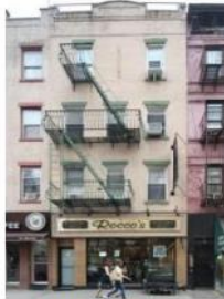
243 Bleeker Street Altered Federal c.1829; altered 1921
