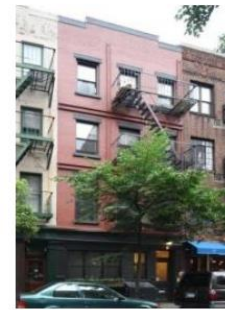
25 Bedford Street Altered Federal c.1828; altered 1888, and 1965
