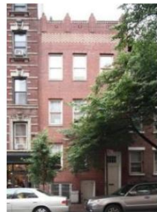
12-12 1/2 Bedford Street Federal, now vernacular Moderne
