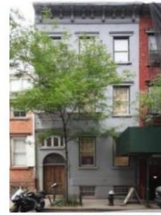
40 Bedford Street Altered Federal, with Italianate and Colonial Revival details 1835-36; altered 1877, and 1930
