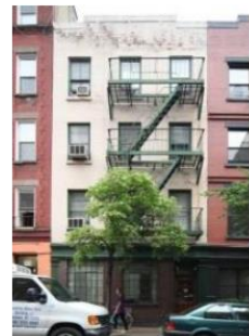
23 Bedford Street Altered Federal c.1828; altered 1885, and 1939
