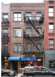
27 Bedford Street Altered Federal, now Moderne c.1828; altered 1888, and 1941
