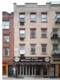
245 Bleeker Street Altered Federal c.1829; altered 1926
