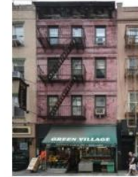
241 Bleeker Street Altered Federal, now Italianate/Neo-Grec c.1829; altered btwn 1876 and 1885
