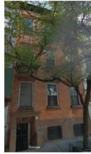
38 Bedford Street Altered Federal, with vernacular Classical details 1835-36; altered 1923, and 1930
