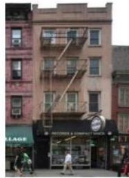
239 Bleeker Street Altered Federal c.1828; altered 1872
