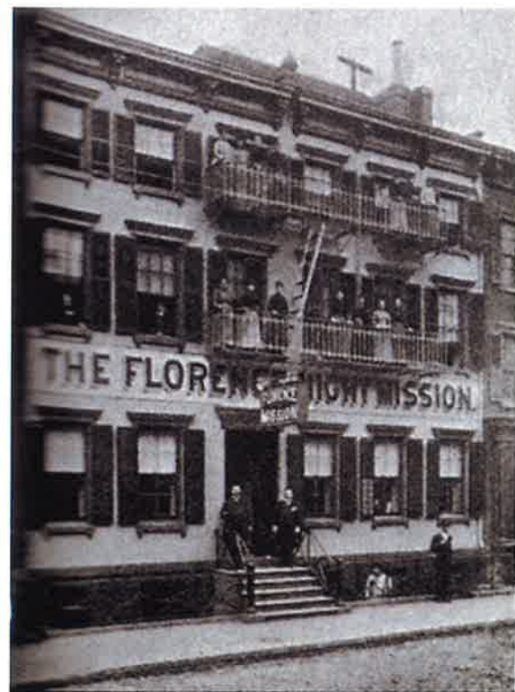
21-23 BLEECKER STREET PHOTO DATE C. 1893?
