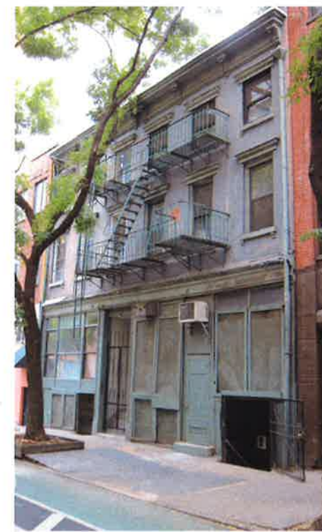
21-23 BLEECKER STREET PHOTO 10/2015 Source: Union Street Studio
