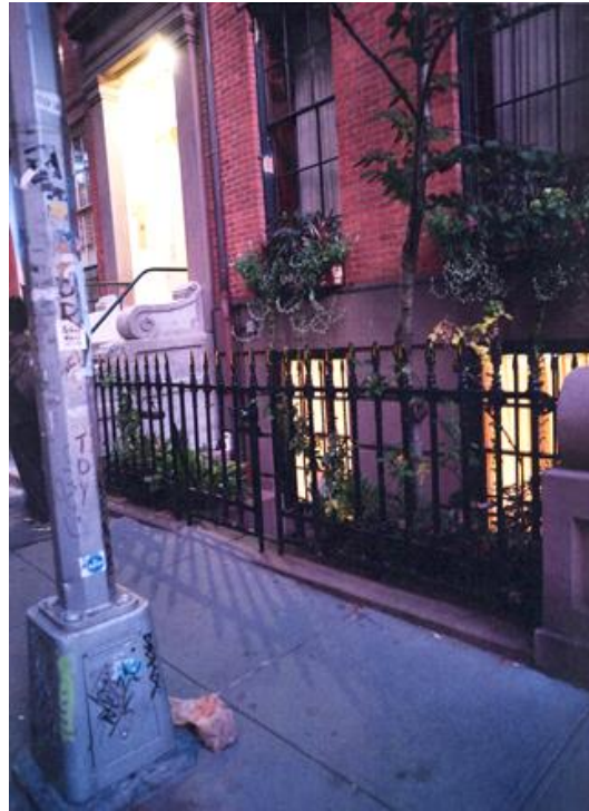
View of fence and parlor windows to be covered by grilles
