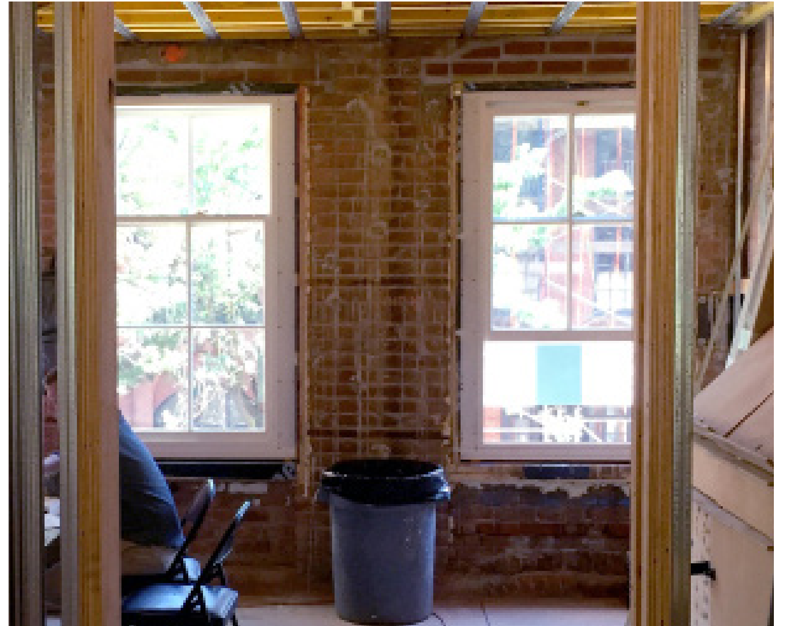
REMEDIATED BRICK South (Front) Facade
