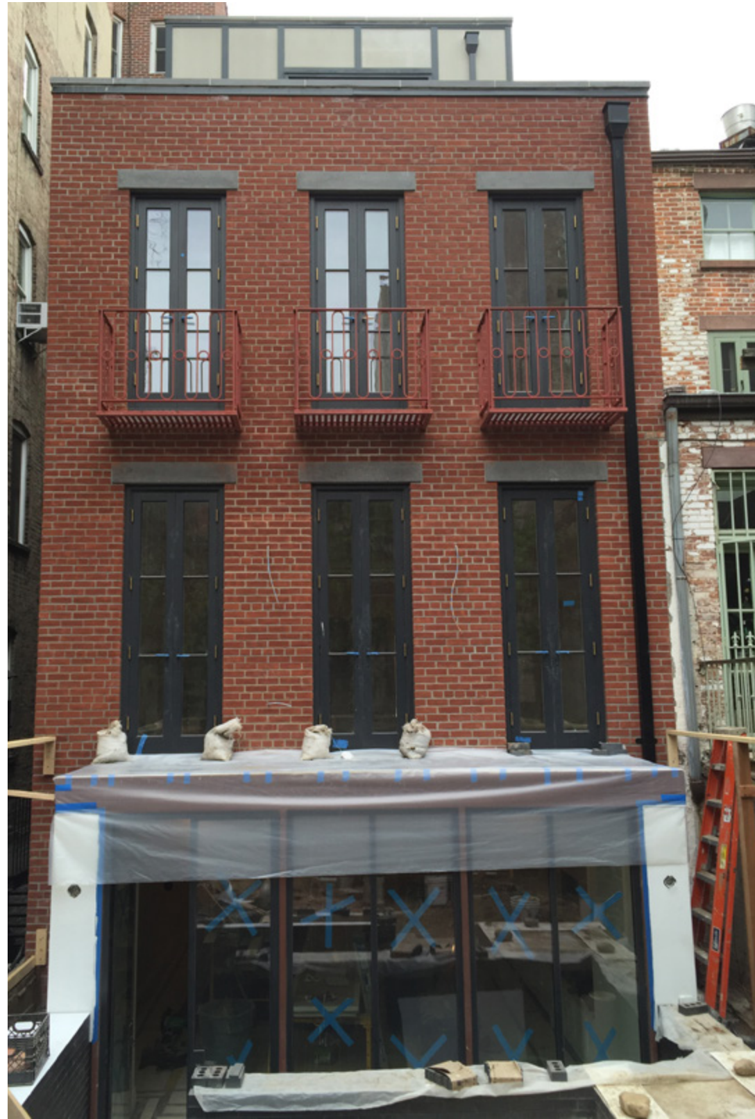
REAR FACADE Basement through Second Floor
