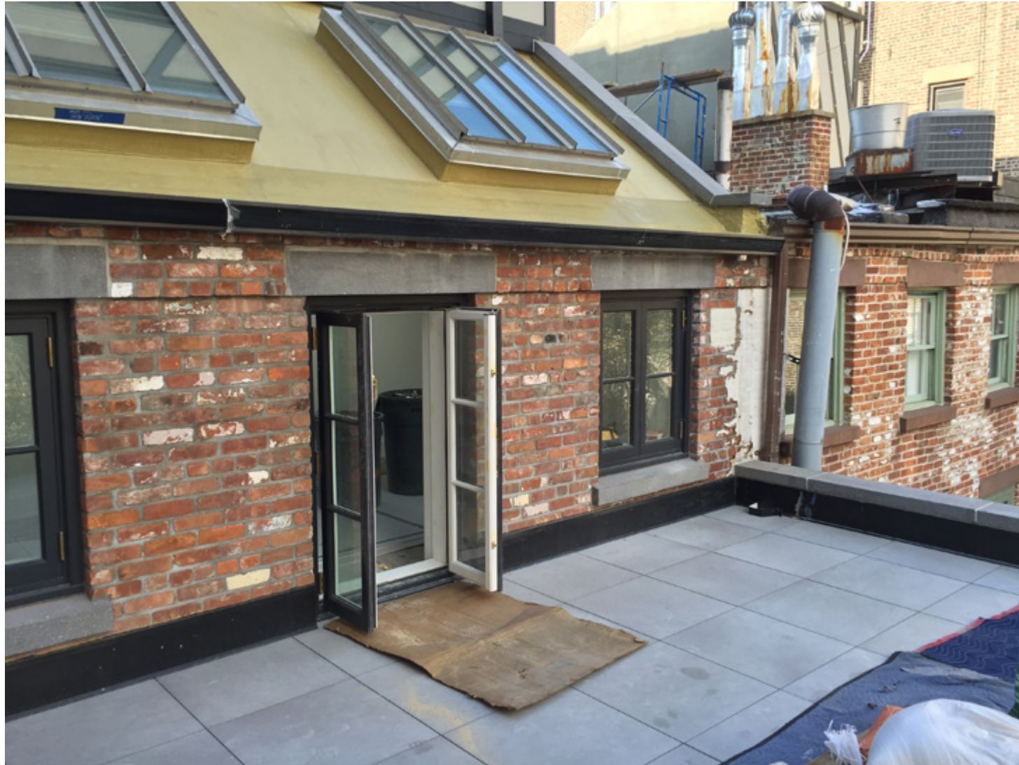
REAR FACADE Third Floor Rear Terrace
