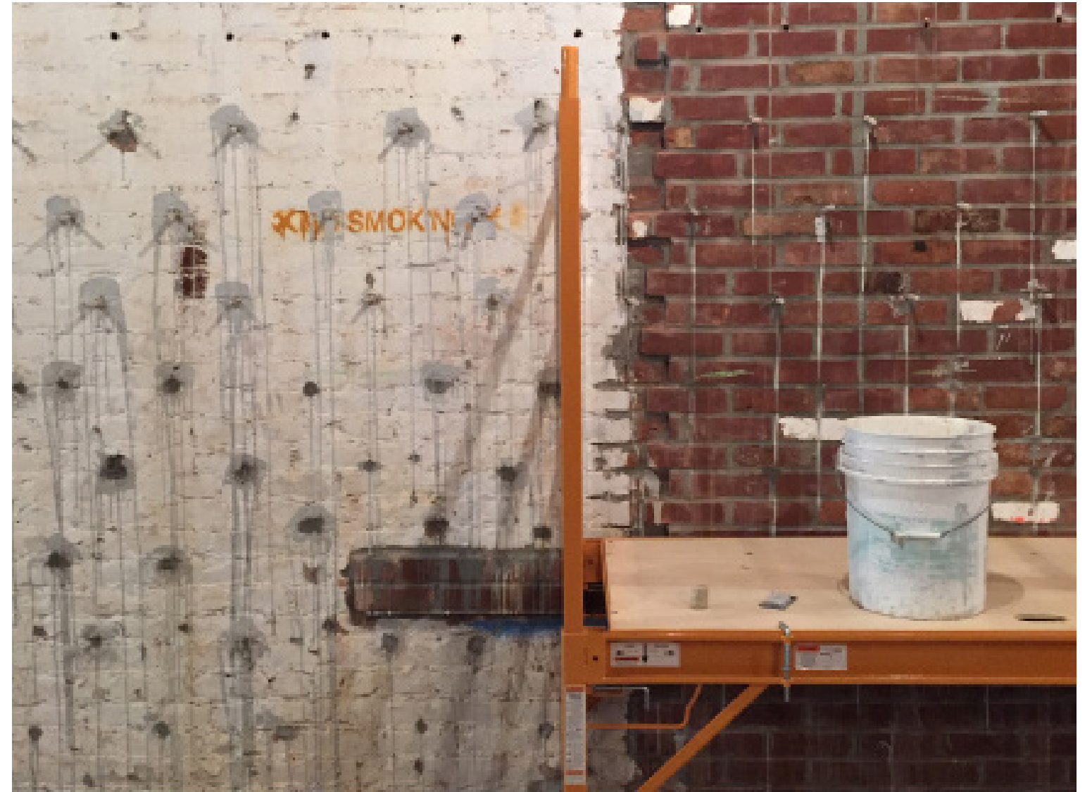
REMEDIATED BRICK East Wall
