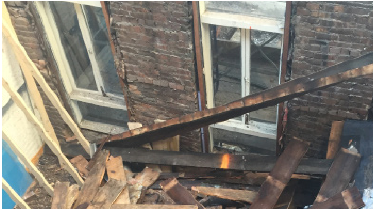
EXISTING DETERIORATED BRICK North (Rear) Facade
