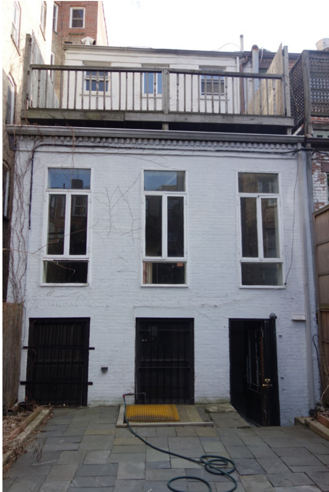
REAR FACADE Basement through Second Floor
