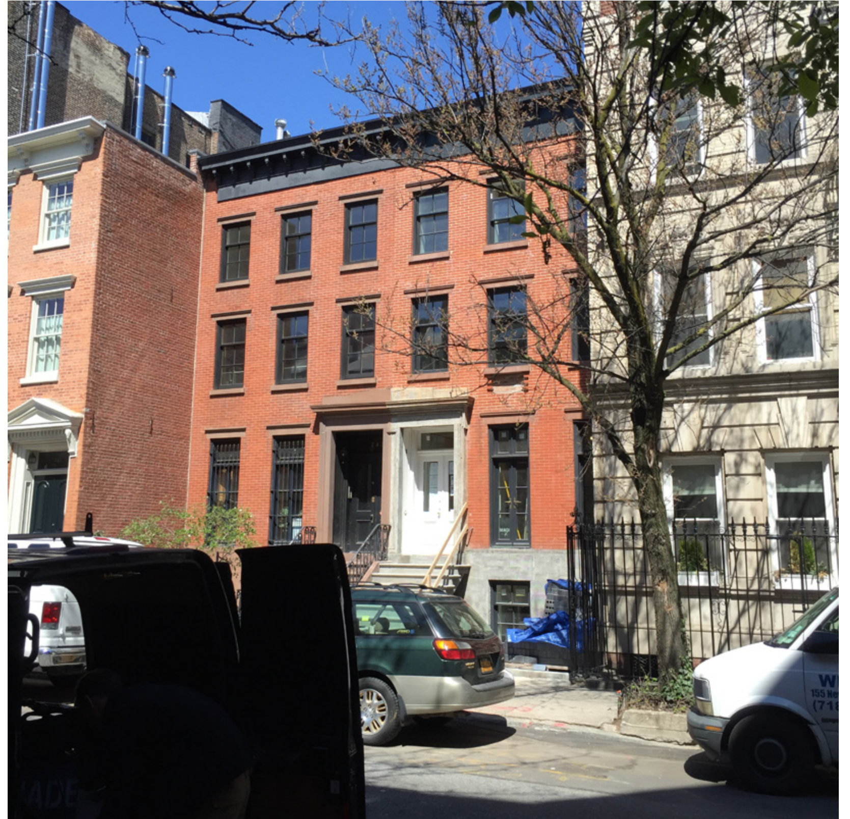
PHOTO Front Facade - Construction In Progress
