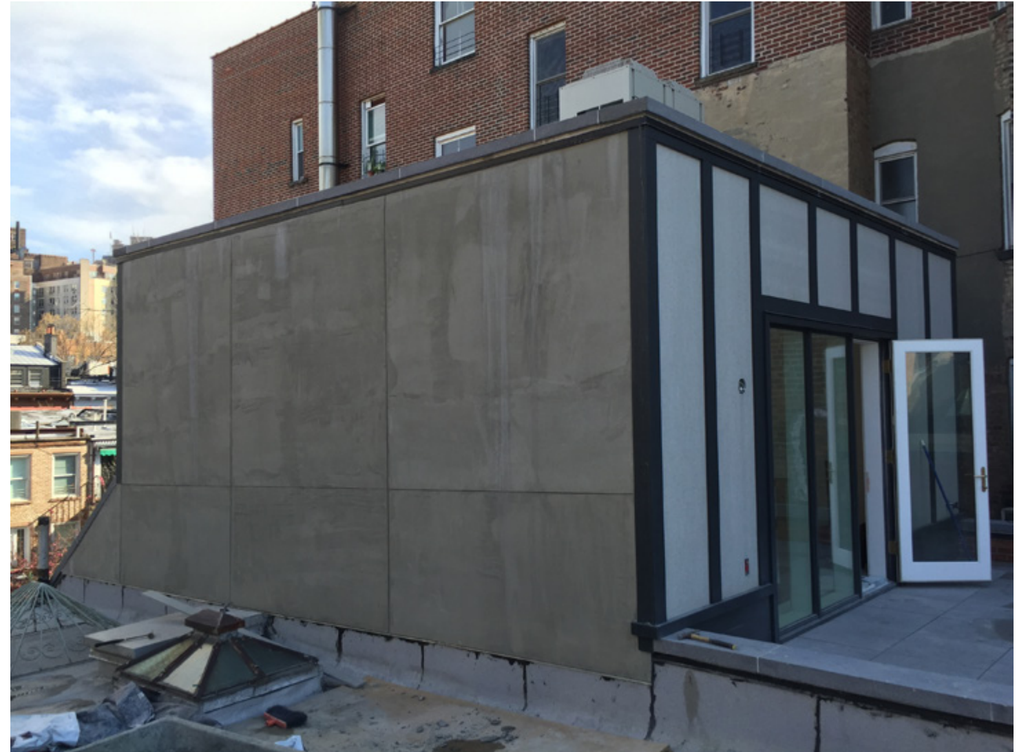
FRONT FACADE Mezzanine Terrace
