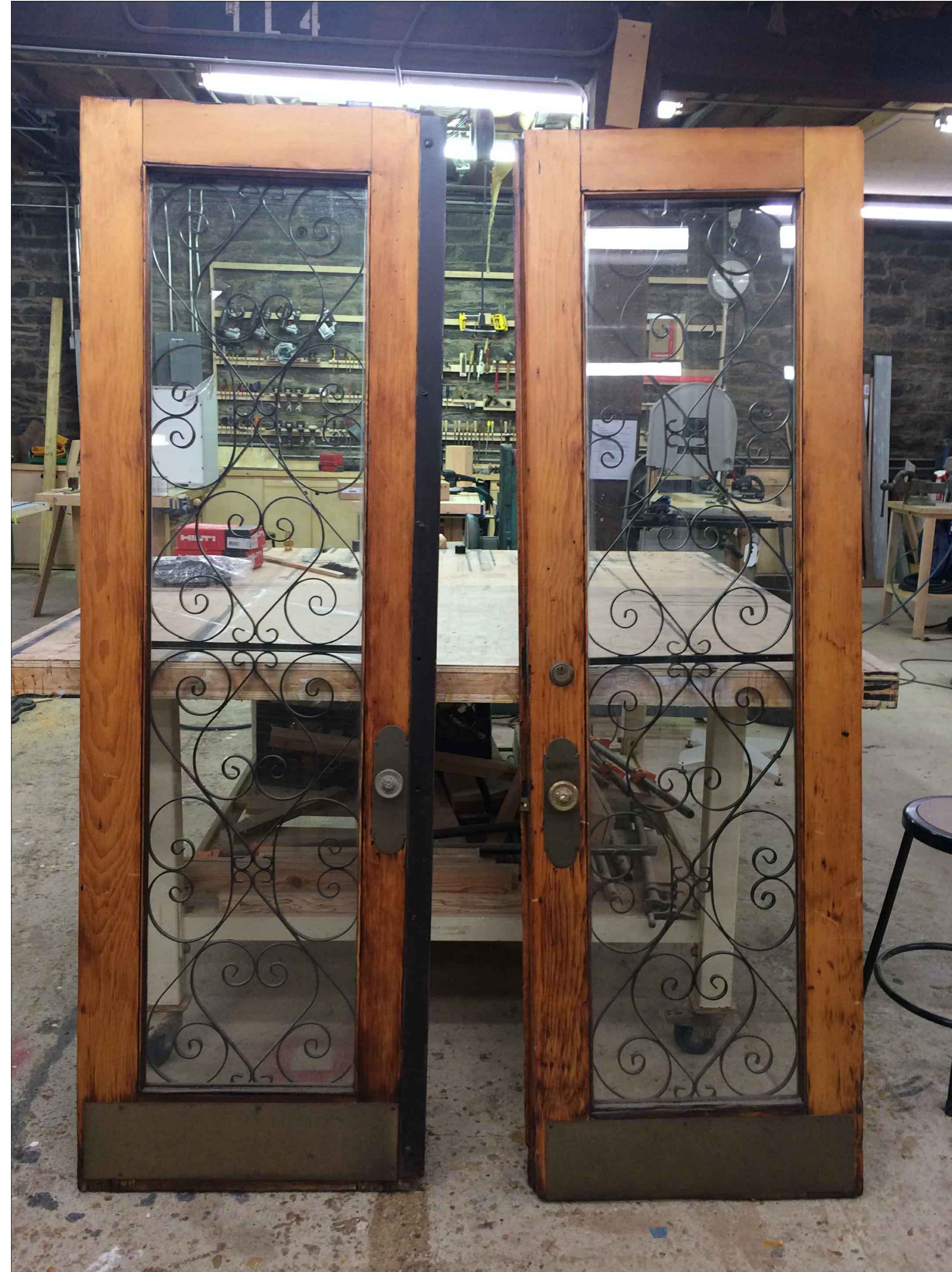
1 L-008 CONDITION OF EXISTING DOORS
