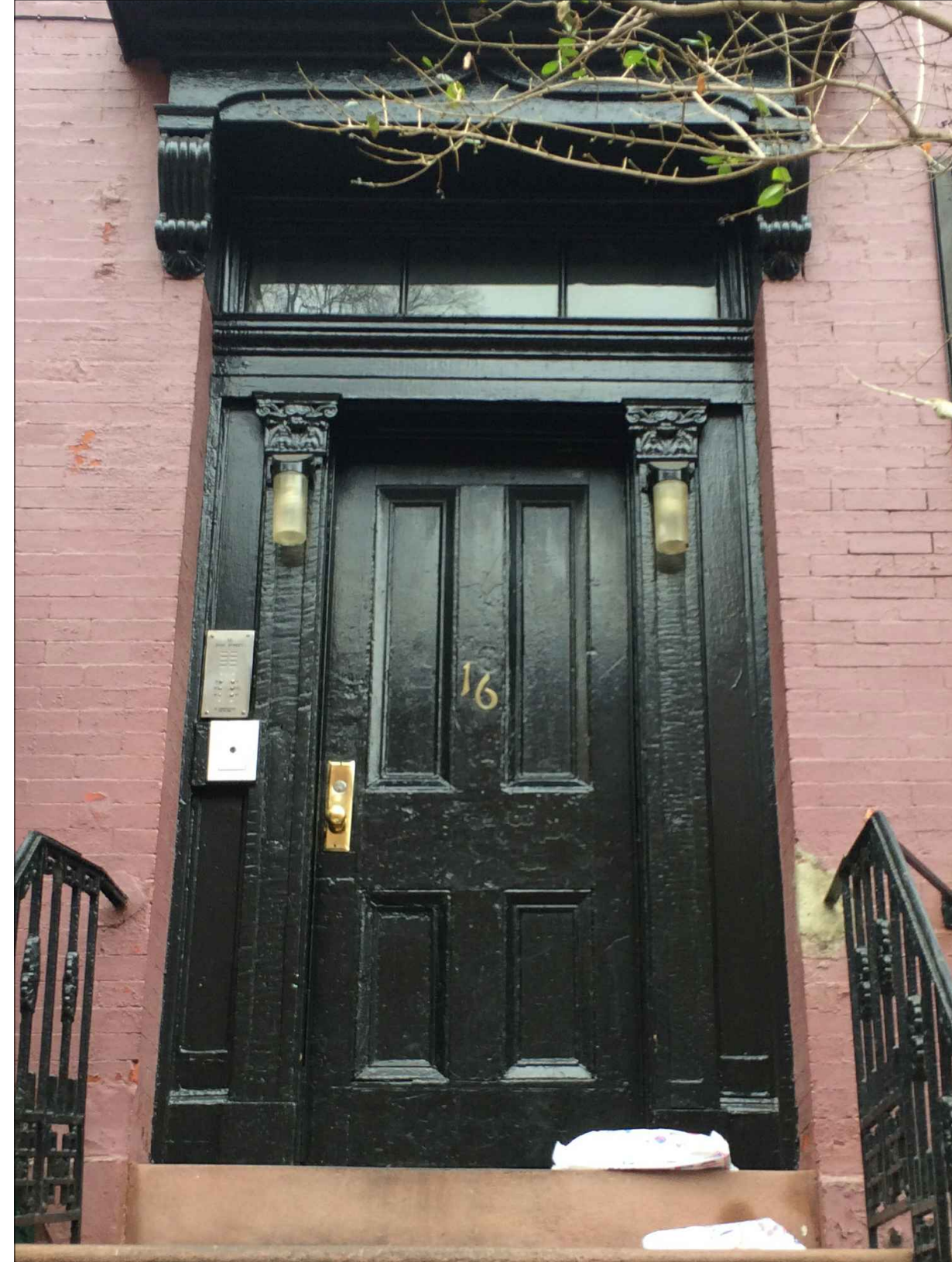
7 DOOR SURROUND AT 16 BANK STREET L-006
