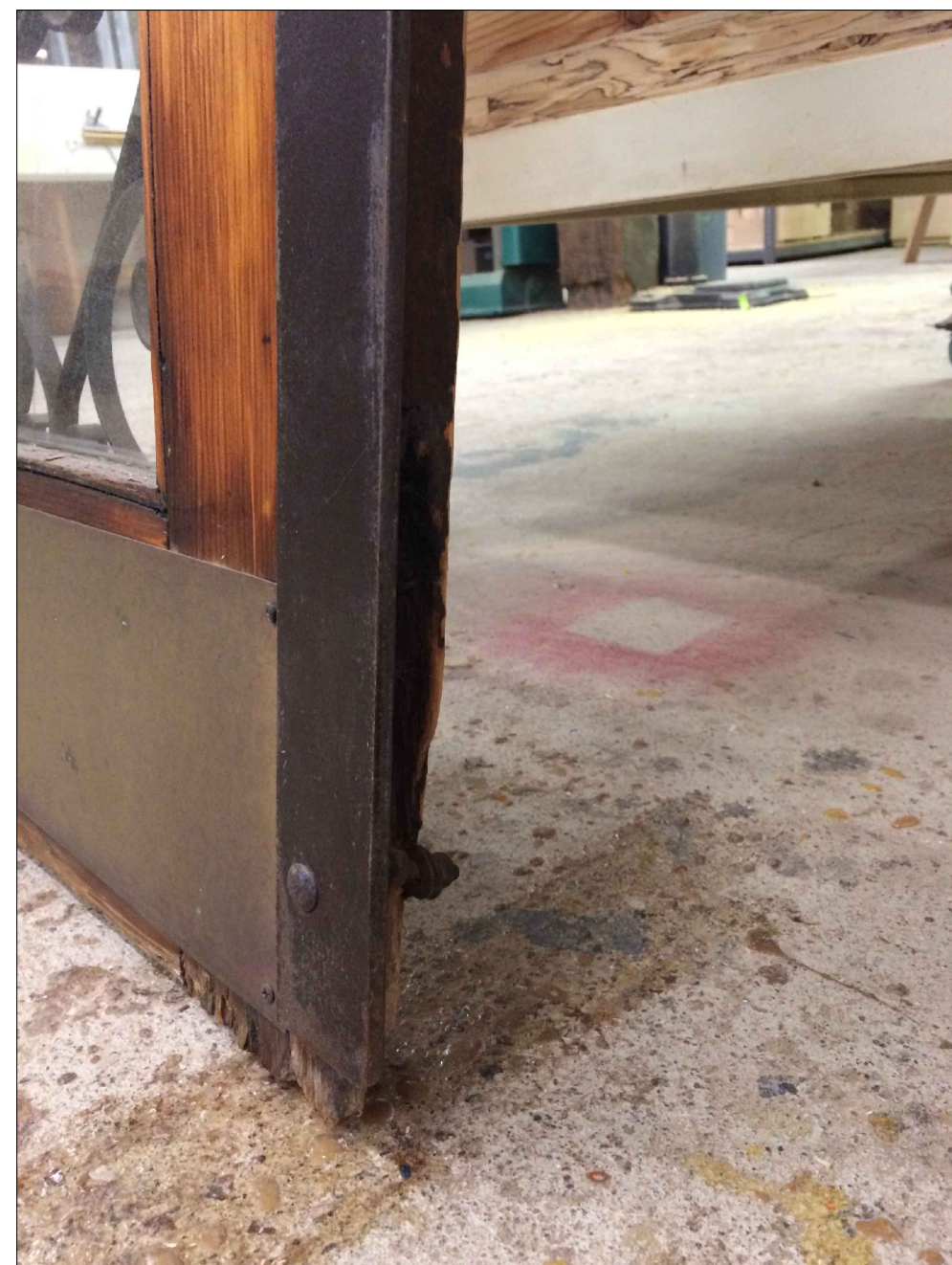
2 L-008 CONDITION OF EXISTING DOORS
