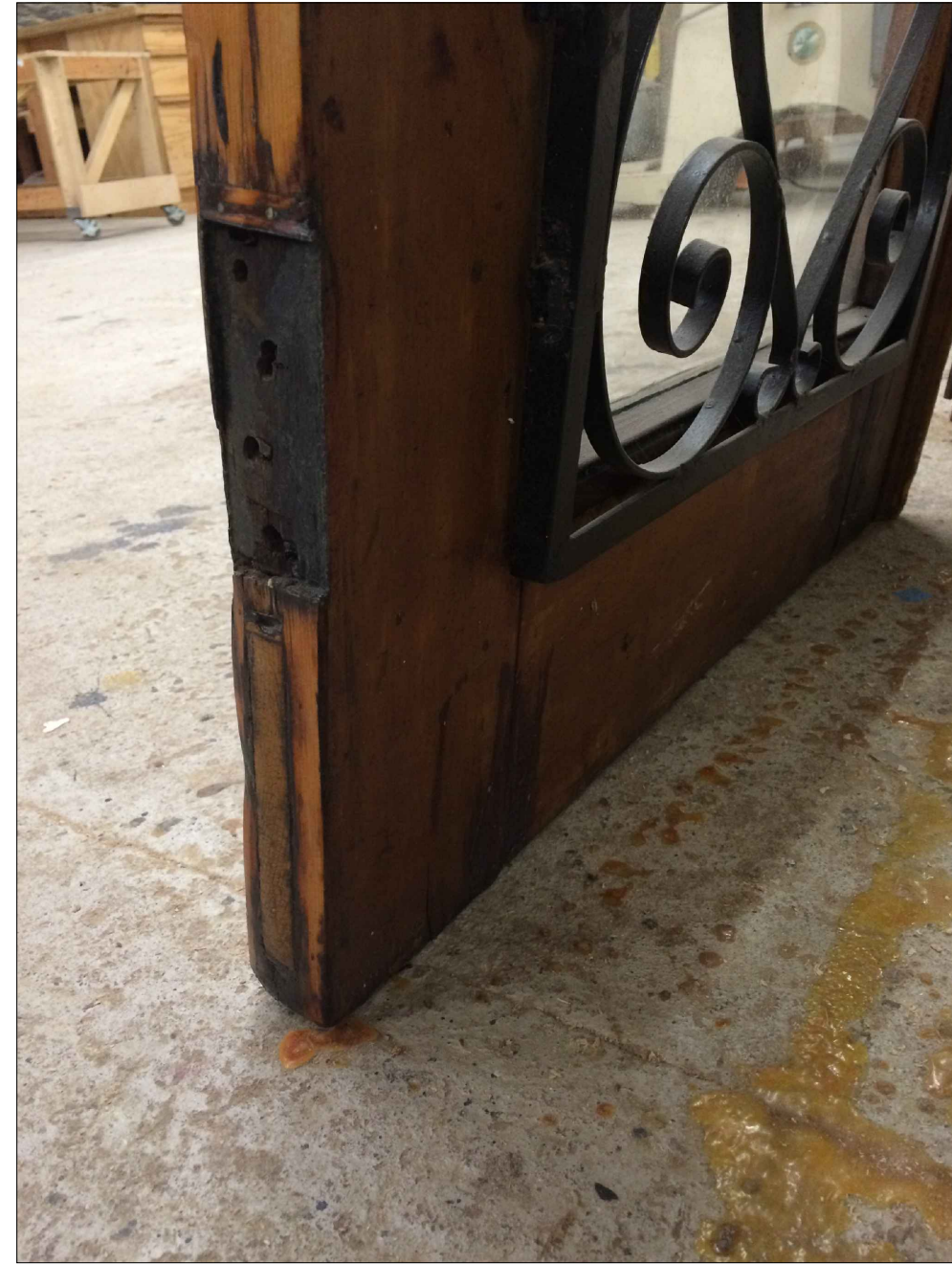
3 L-008 CONDITION OF EXISTING DOORS
