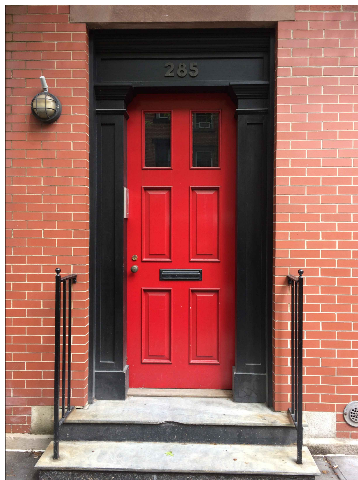
5 DOOR SURROUND AT 285 WEST 11TH ST L-006
