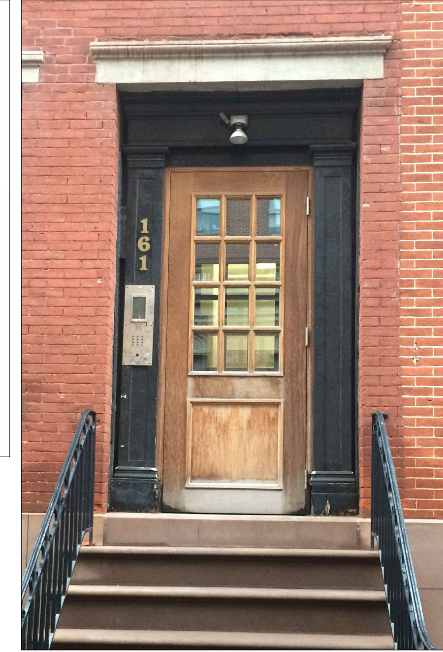
3 DOOR SURROUND AT 161 WEST 12TH ST L-006
