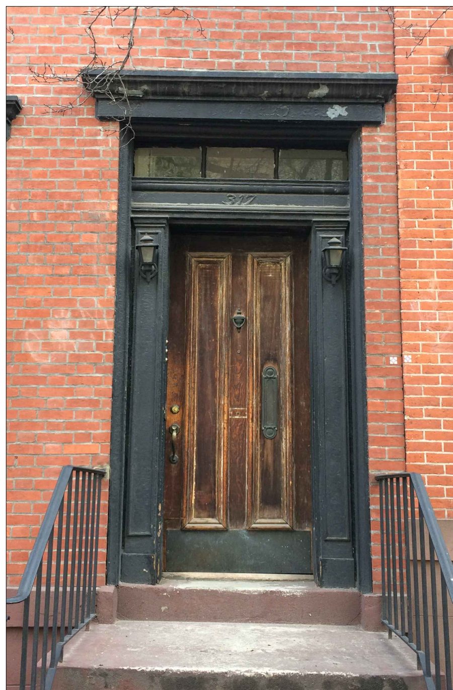
1 DOOR SURROUND AT 317 WEST 4TH ST L-006
