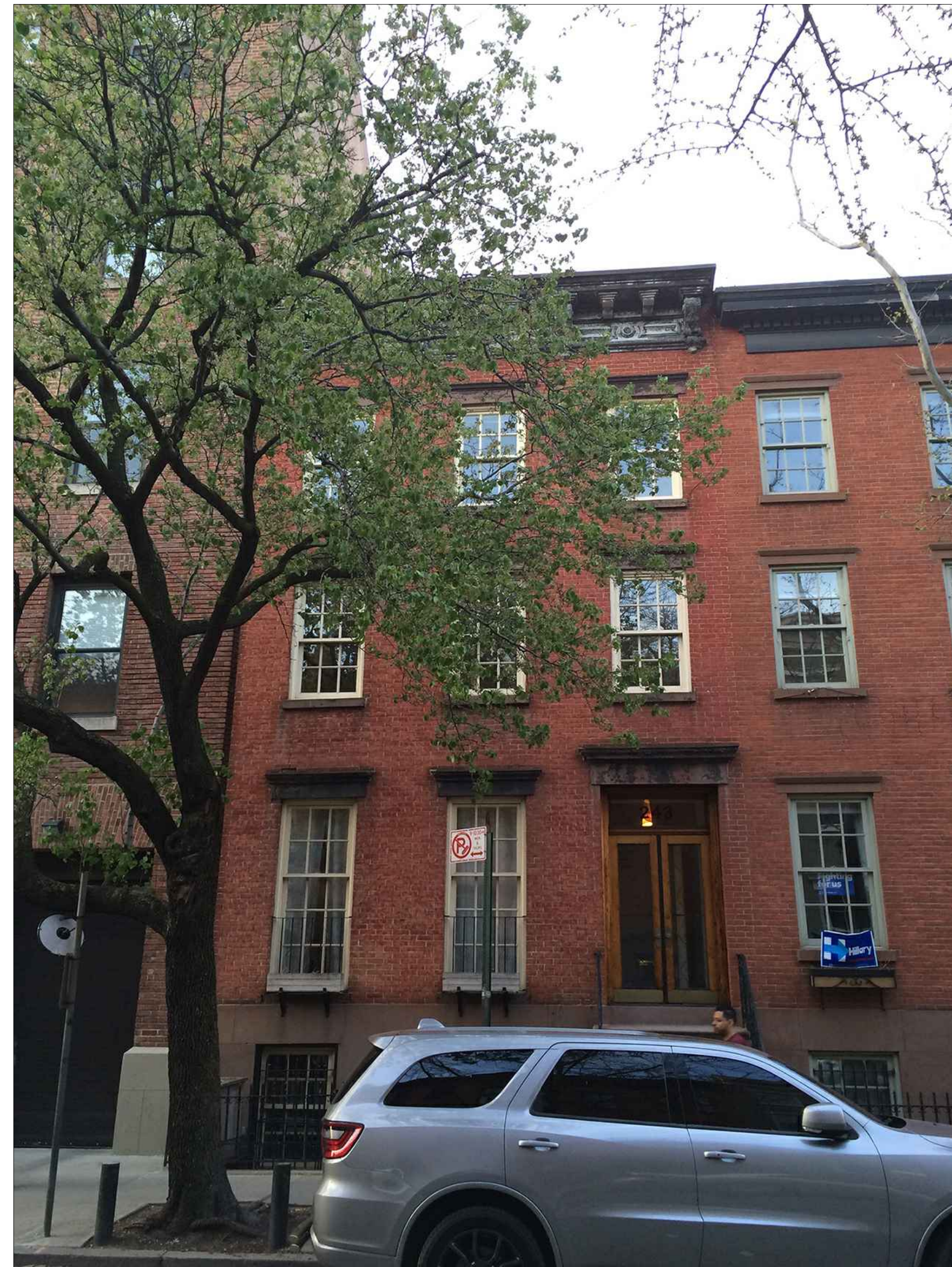
2 EXISTING DOOR AND SURROUND L-007
