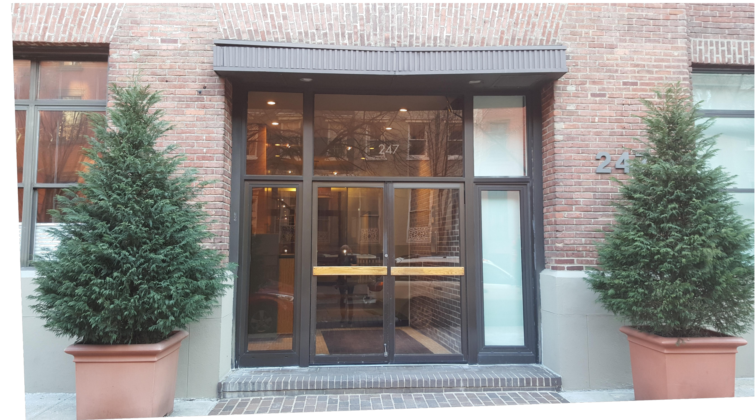
4 PHOTO OF EXISITNG BUILDING ENTRANCE NOT TO SCALE
