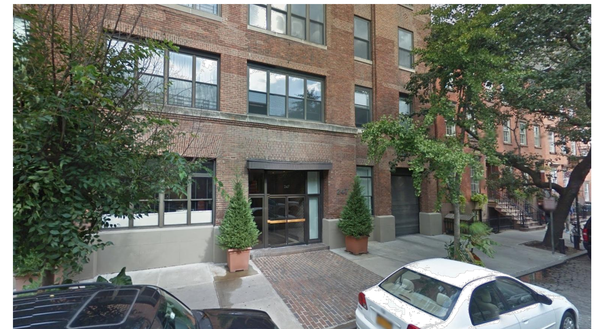
5 PHOTO OF EXISITNG BUILDING ENTRANCE NOT TO SCALE
