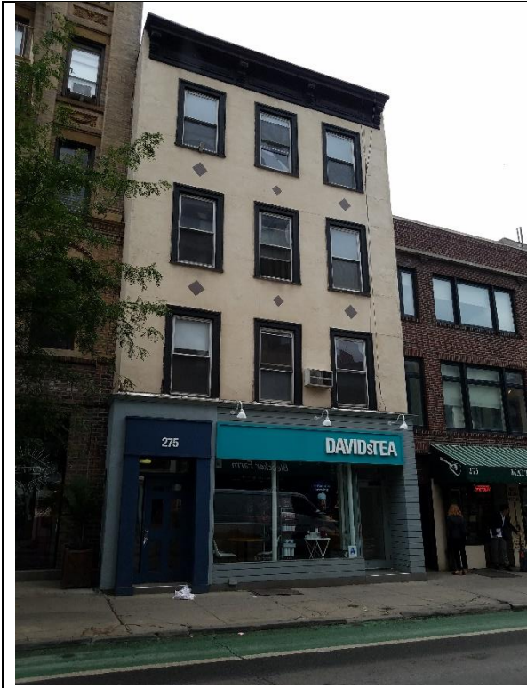
275 BLEECKER FRONT FAÇADE IN GOOD CONDITIONS
