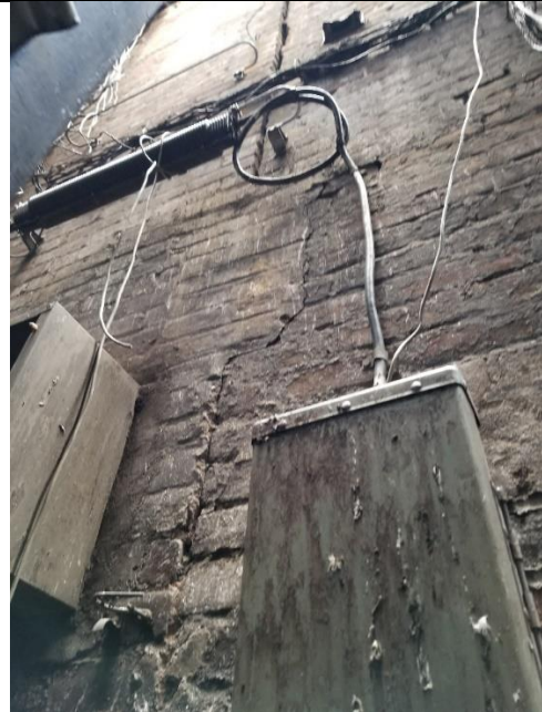
VERTICAL MEDIUM CRACK AT 275 BLEECKER SIDE FAÇADE
