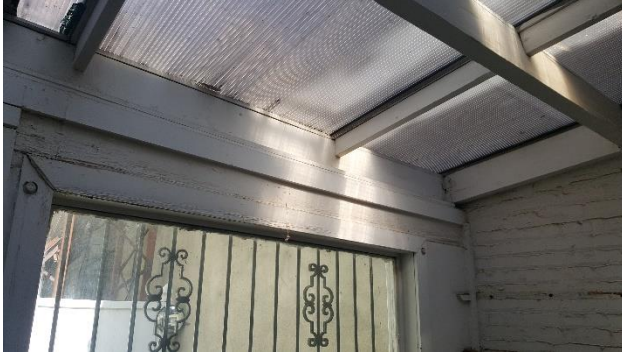
REAR EASTERN PORTION WOOD FRAMING
