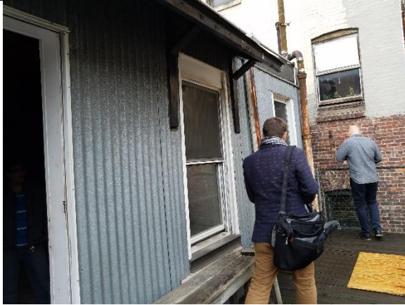
REAR FAÇADE FOURTH FLOOR CORRUGATED STEEL
