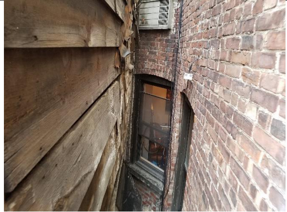
WEST FAÇADE FRONT PORTION WOOD CLADDING
