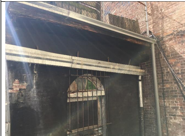
REAR FAÇADE FIRST FLOOR WESTERN PORTION
