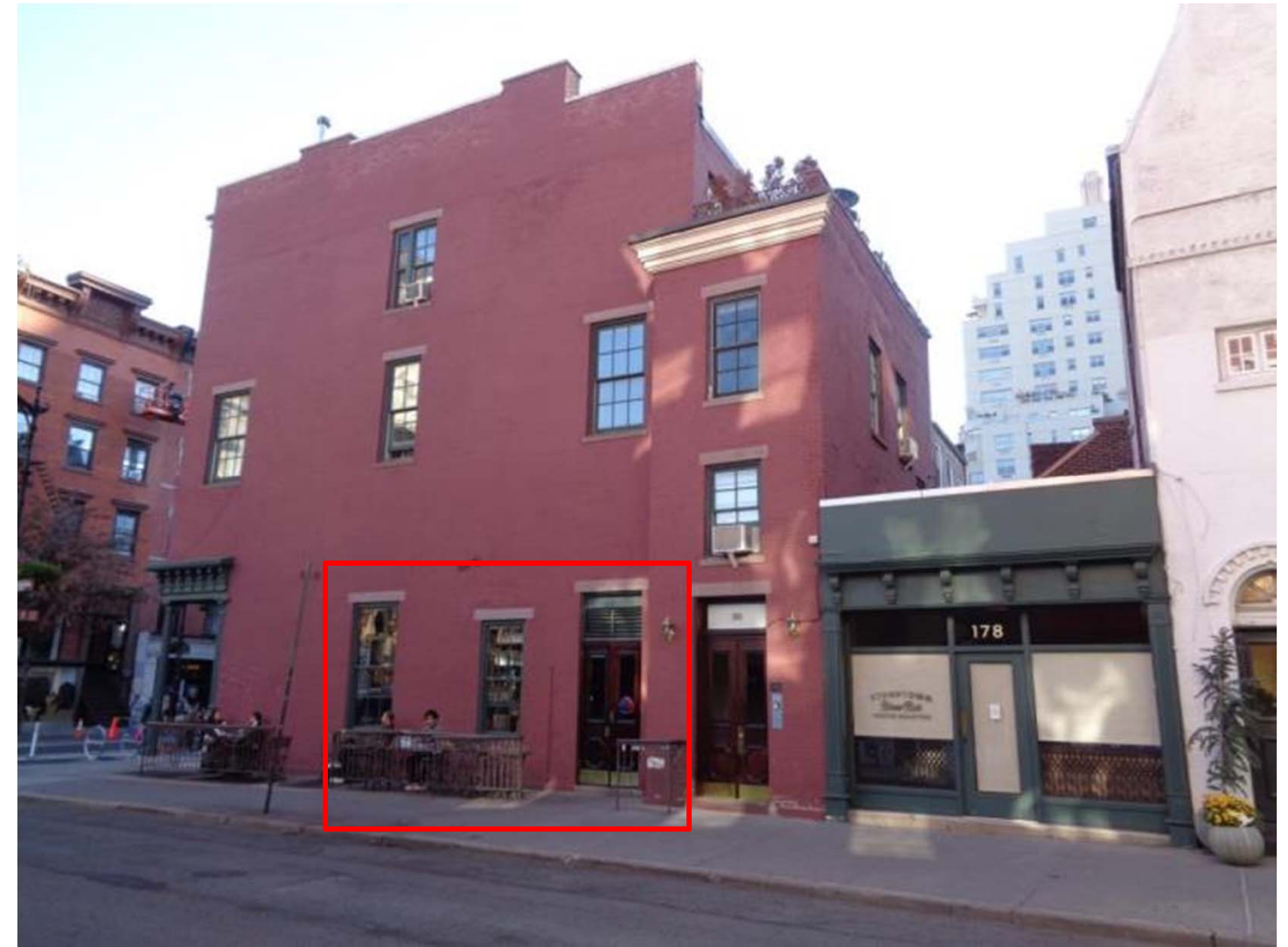
Photo 4: Current photo of the property showing the West (MacDougal Street) facing primary facade. Outline depicts the area of proposed work. Existing windows and facade elements to remain.
