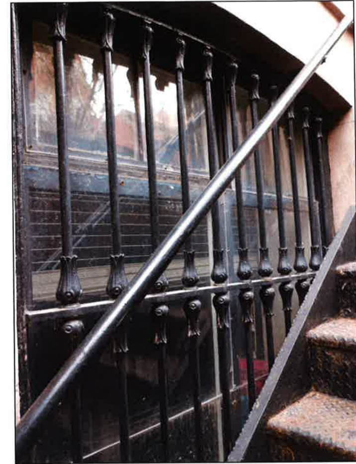
AREAWAY/ CELLAR WINDOW - 30 W 10TH ST
