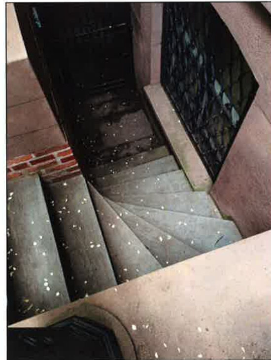
AREAWAY STAIR - 26 W 10TH ST
