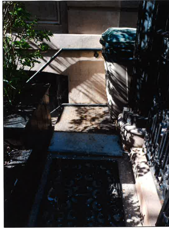
AREAWAY STAIR - 30 W 10TH STREET
