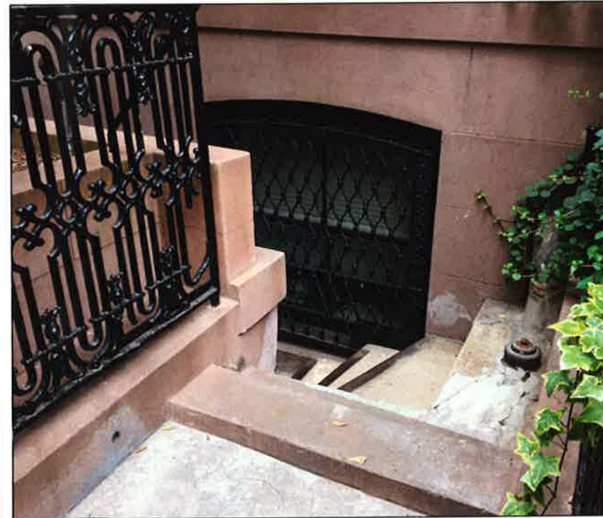
AREAWAY STAIR- 36 W 10TH STREET
