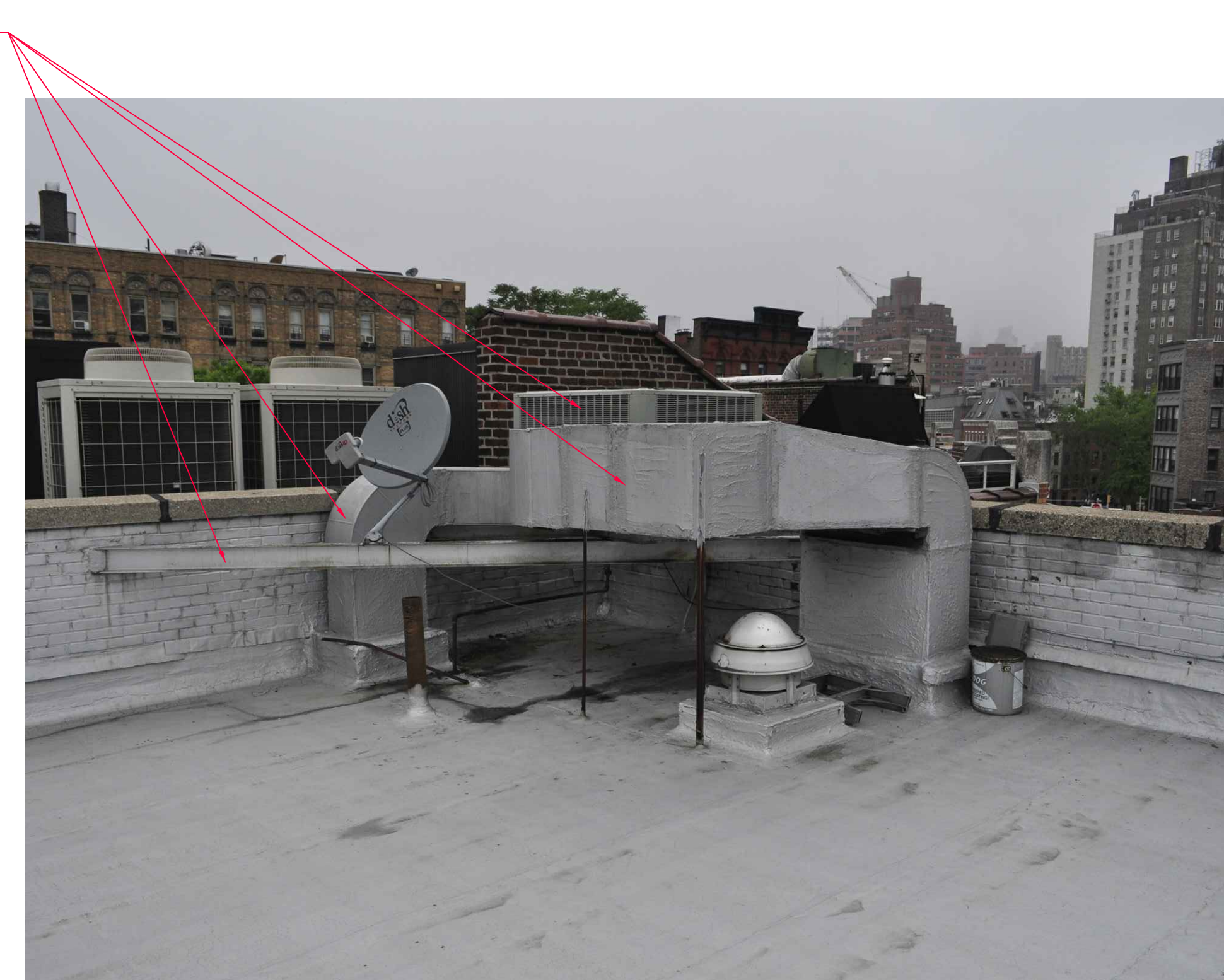
PHOTOGRAPH #8 3RD FLOOR ROOF - 84-86 7TH AVENUE SOUTH
