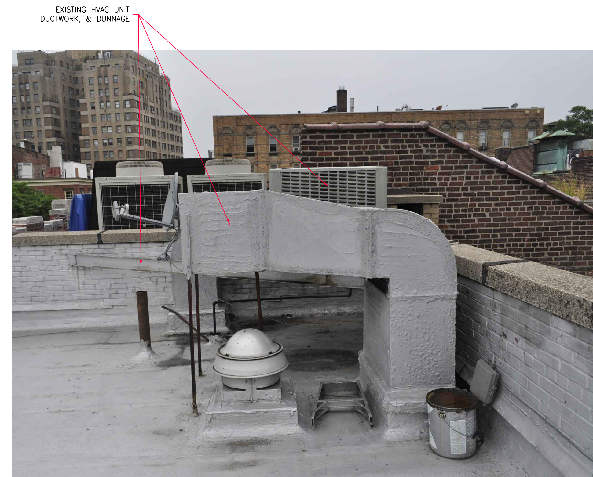
PHOTOGRAPH #6 3RD FLOOR ROOF - 84-86 7TH AVENUE SOUTH
