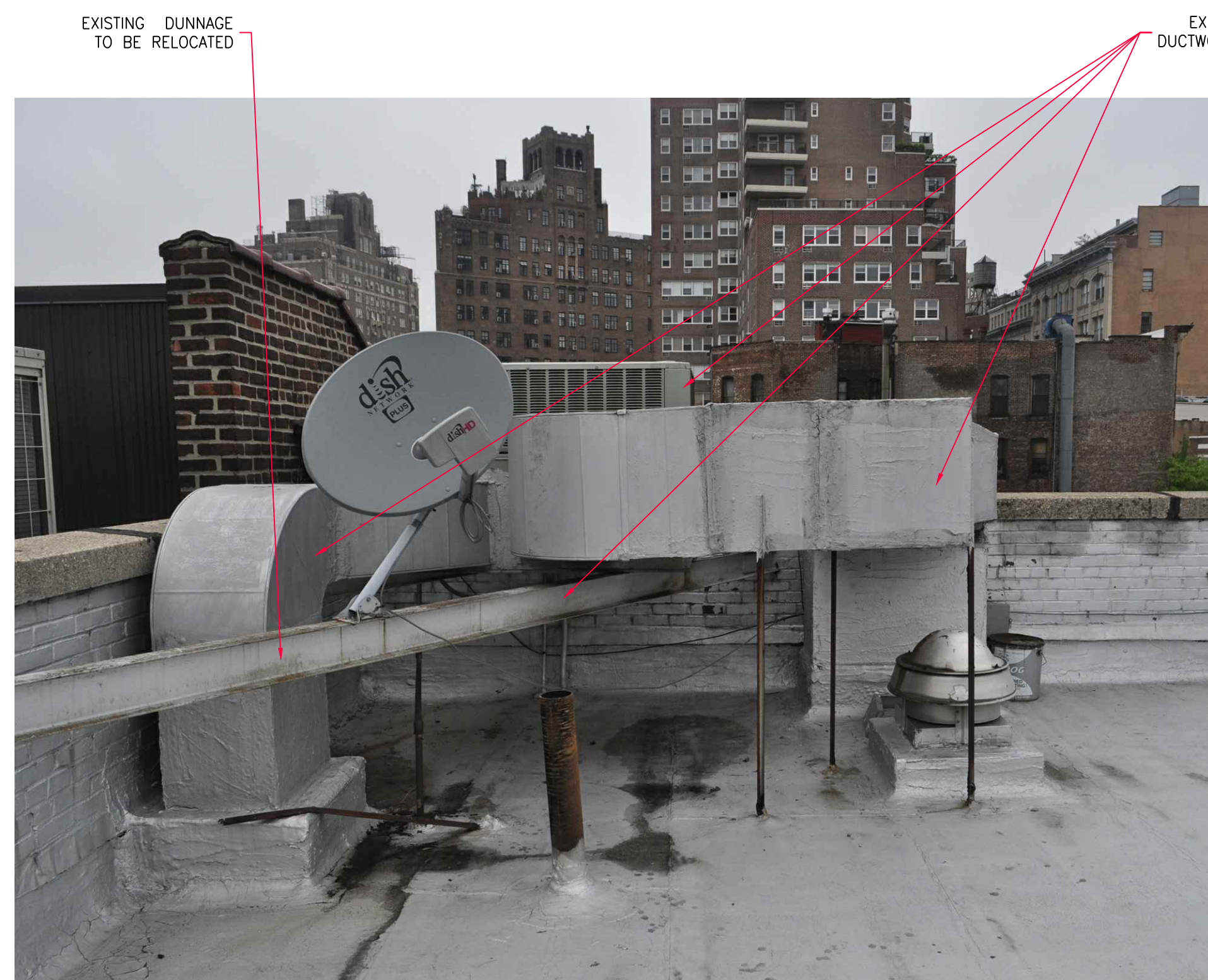
PHOTOGRAPH #7 3RD FLOOR ROOF - 84-86 7TH AVENUE SOUTH
