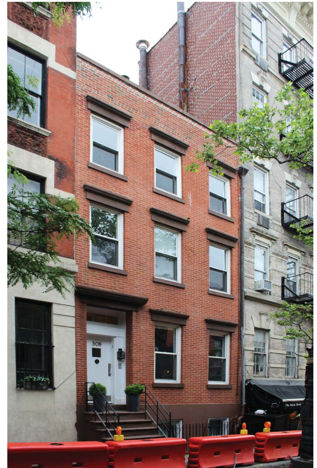
3. EXISTING CONDITION OF 308 WEST 4TH STREET
