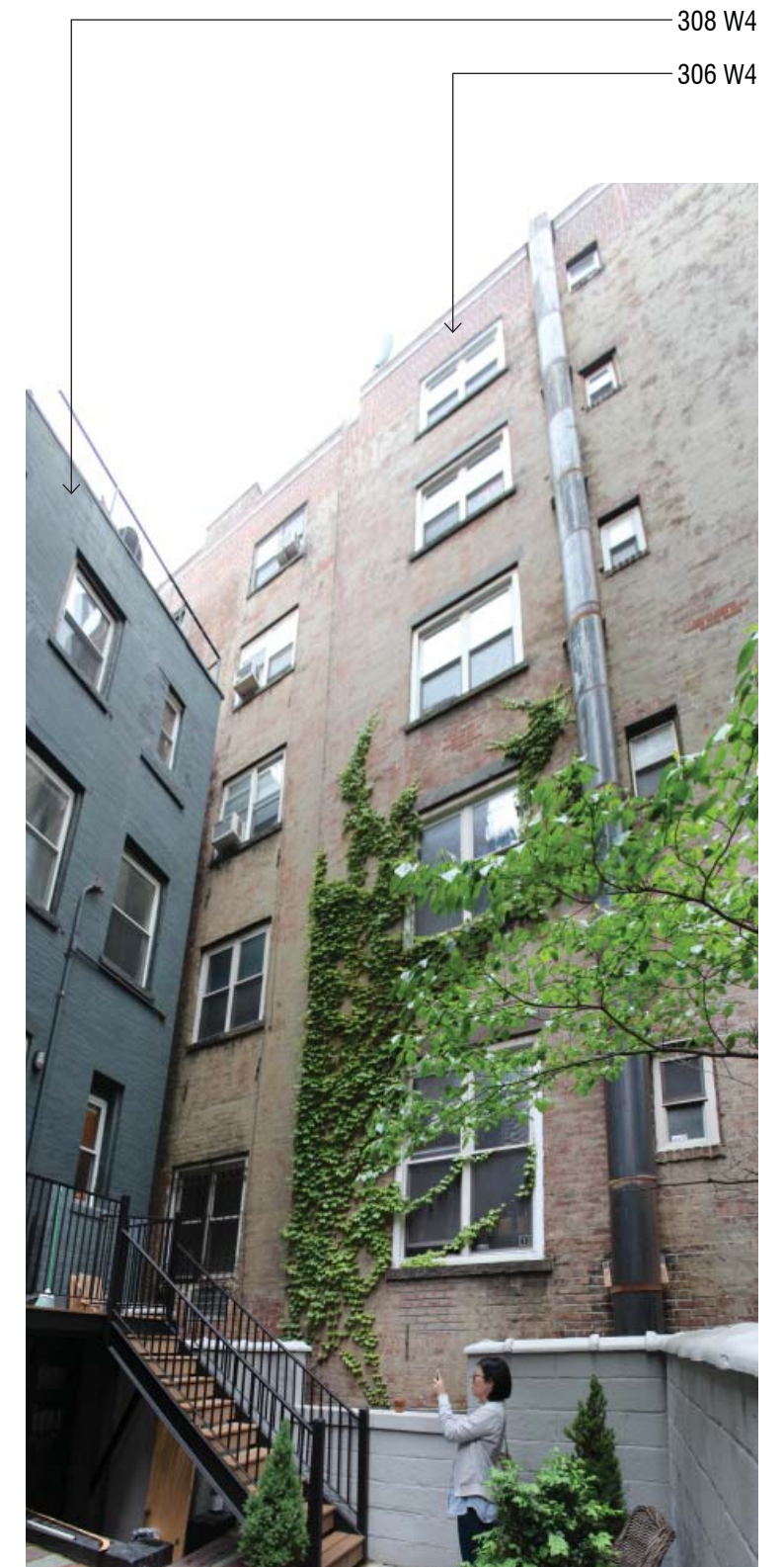
1. REAR YARD LOOKING SOUTH
