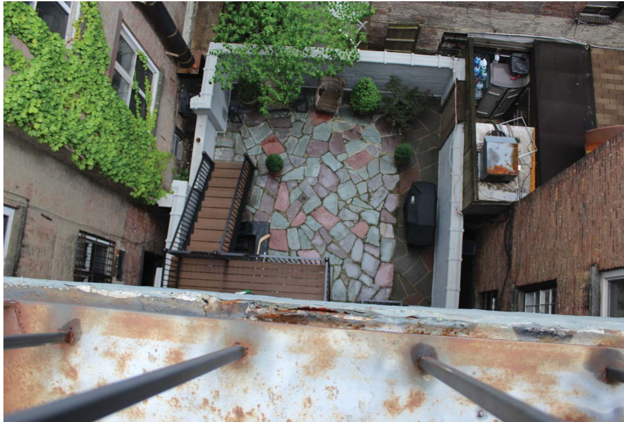
REAR YARD FROM ROOF
