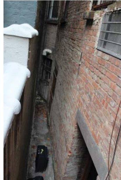
Light well to south
