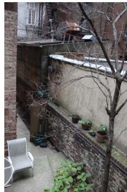
Rear yard wall from 306 West 4th Street, west of yard
