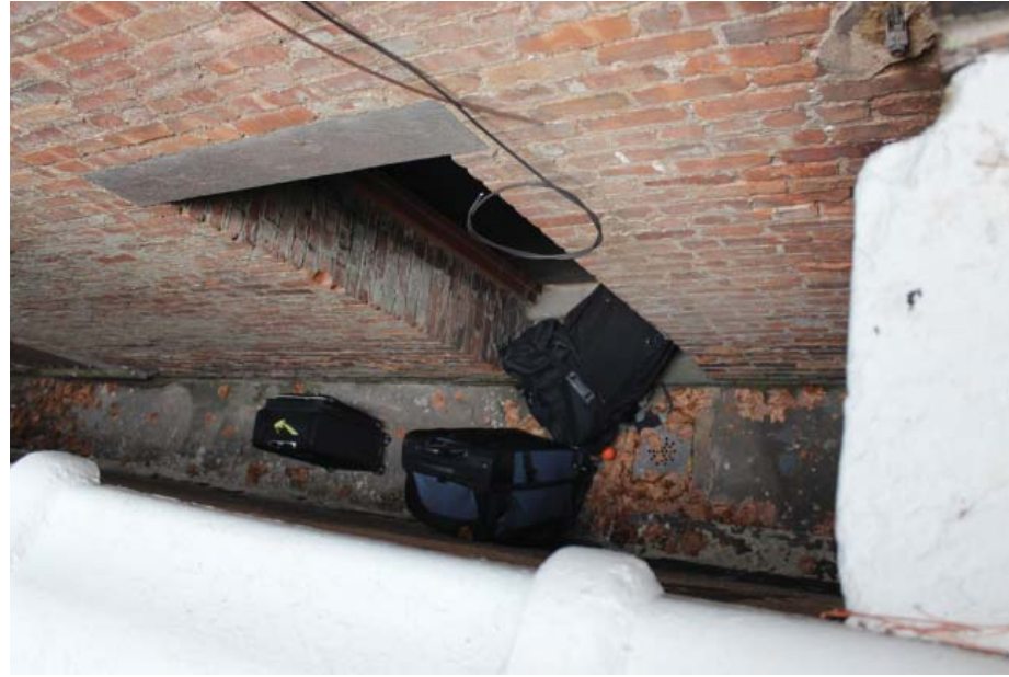
Light well to south
