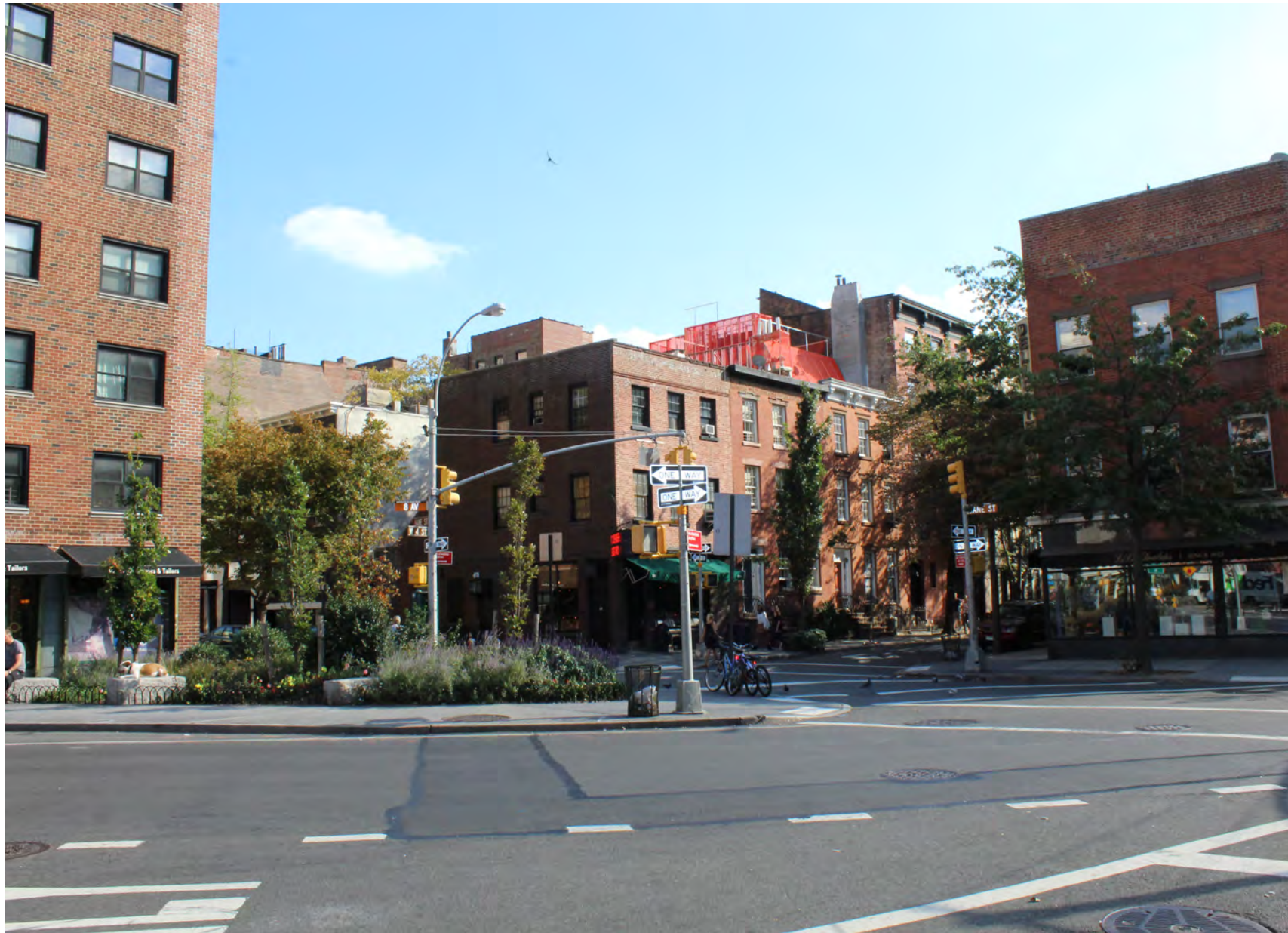
OCTOBER 25 MOCKUP IMAGE (10/19/2016): Seen from across 8th Ave. looking Southeast
