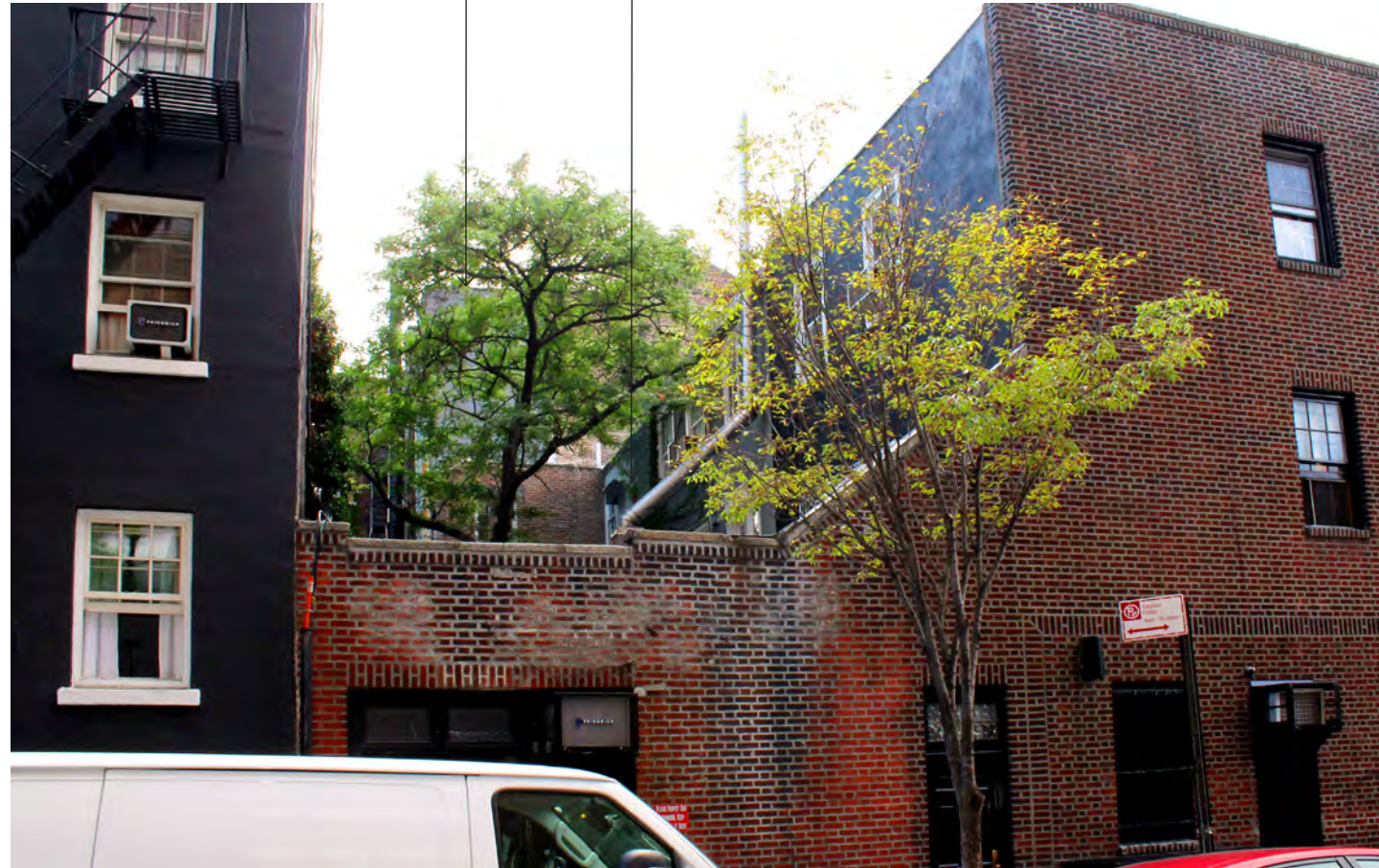
1. CURRENT PHOTO (2016): Jane Street looking south
