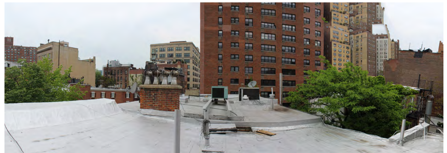
EXISTING ROOFTOP PHOTO (5/13/2016): Looking North
