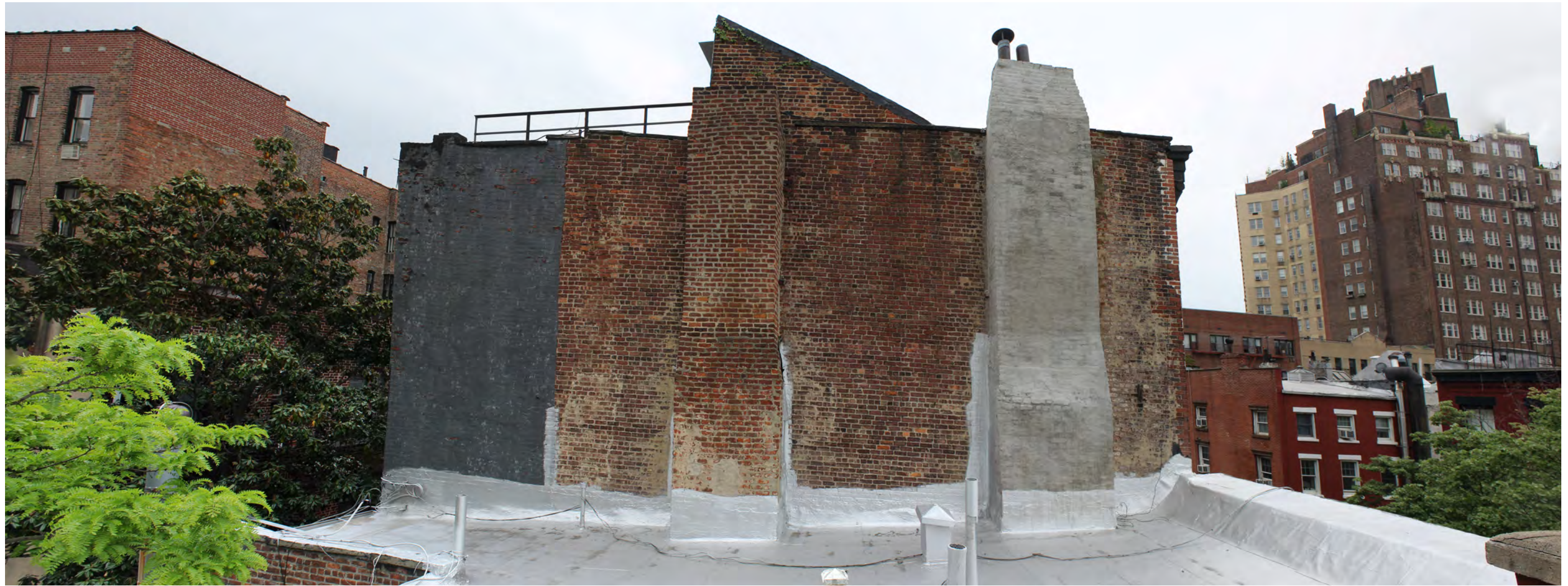
EXISTING ROOFTOP PHOTO (5/13/2016): Looking South
