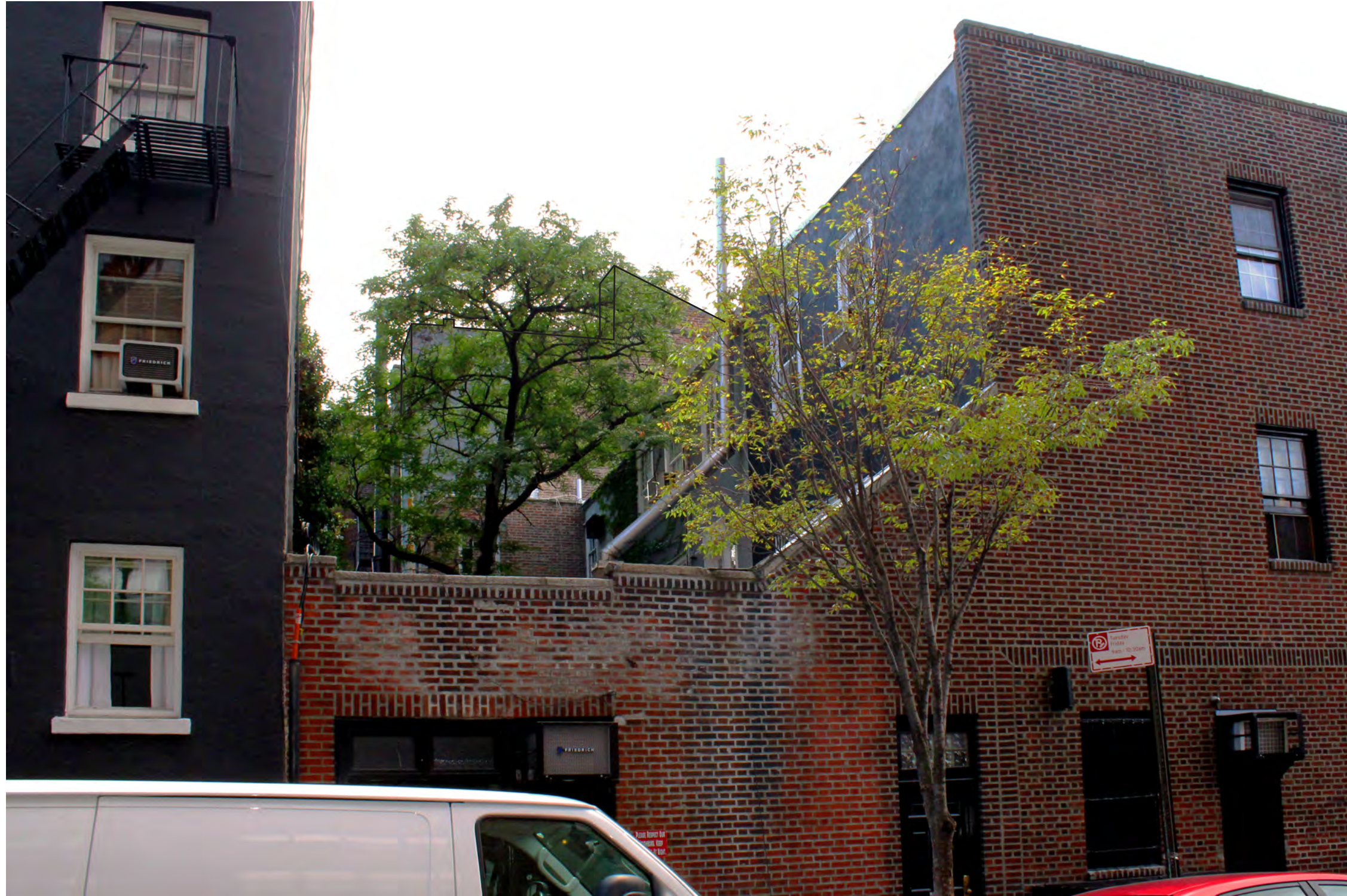
EXISTING BUILDING (5/13/2016): Seen from Jane Street
