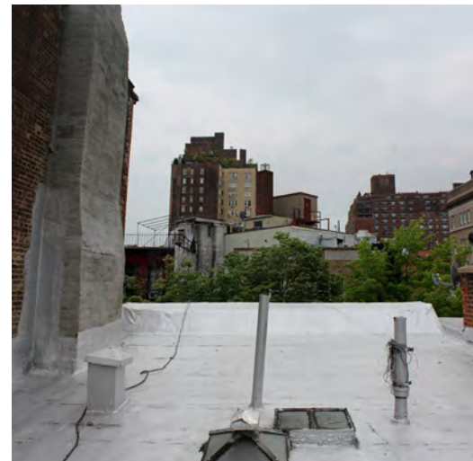
EXISTING ROOFTOP PHOTO (5/13/2016): Looking West
