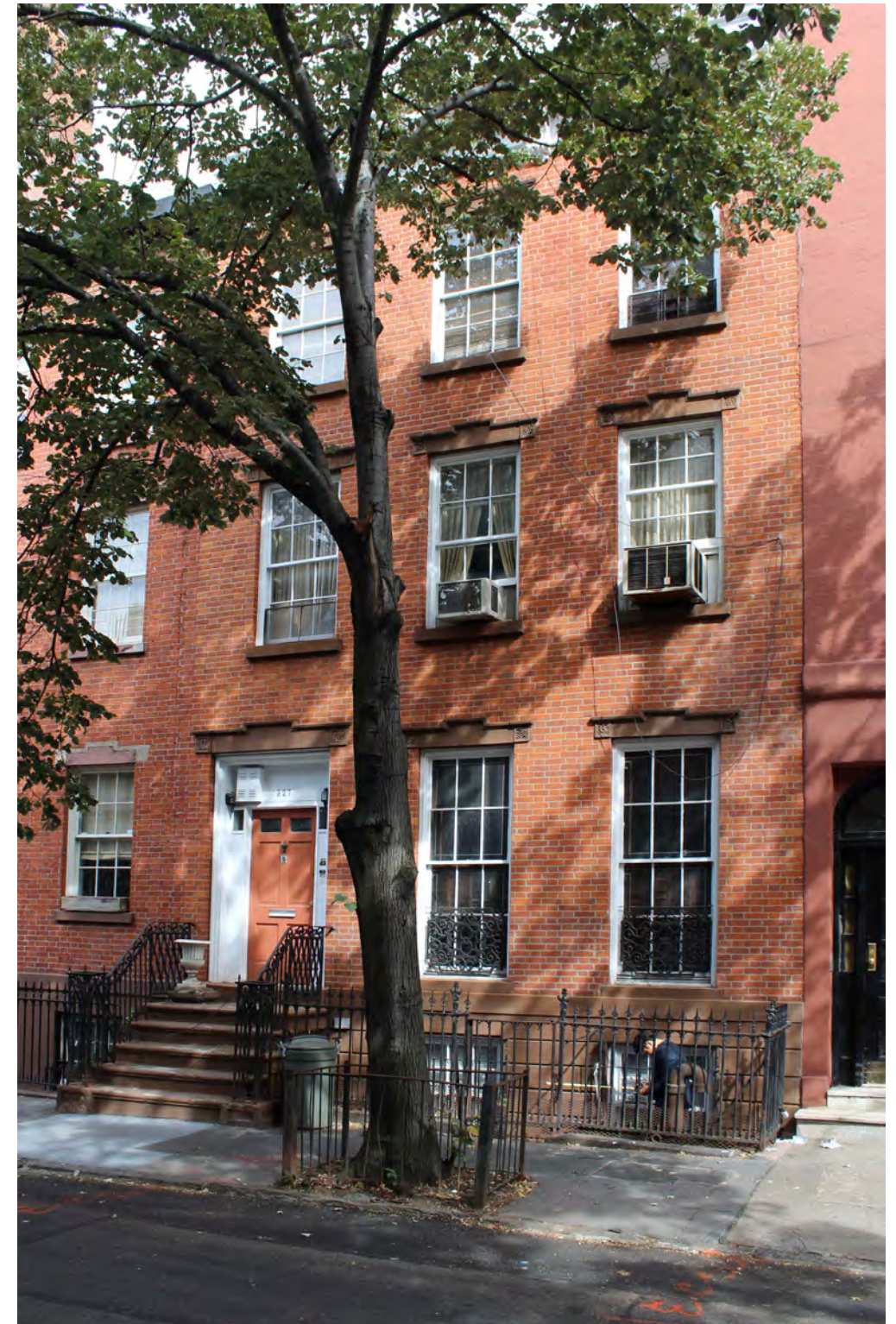
3. EXISTING CONDITION OF 327 WEST 4TH STREET
