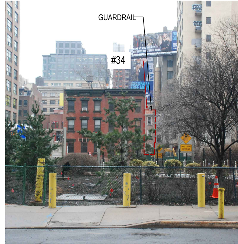
H WATTS ST. SIGHT LINE PHOTO NTS NOTE: SIGHT LINE WILL BE OBSTRUCTED BY 185' HIGH BUILDING, UNDER CONSTRUCTION
