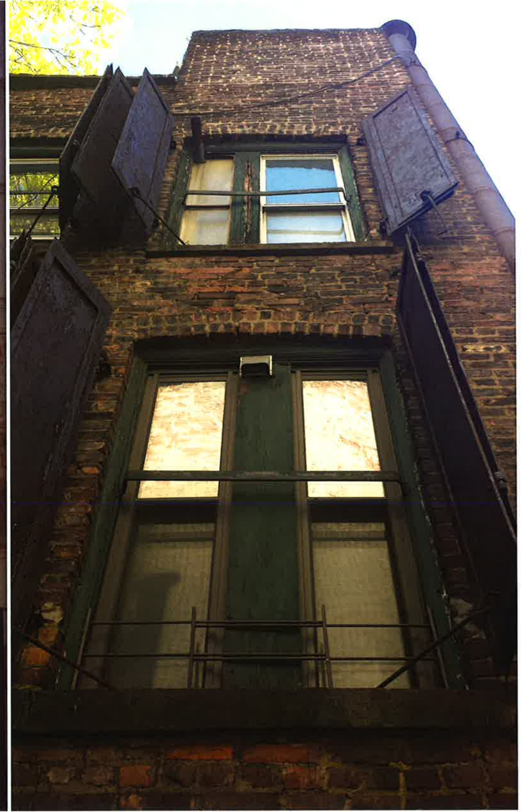
REAR OF THE BUILDING
