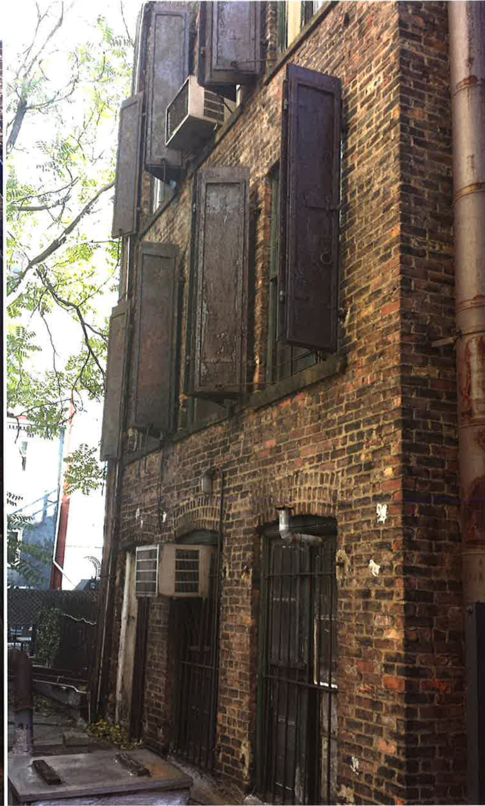
REAR OF THE BUILDING
