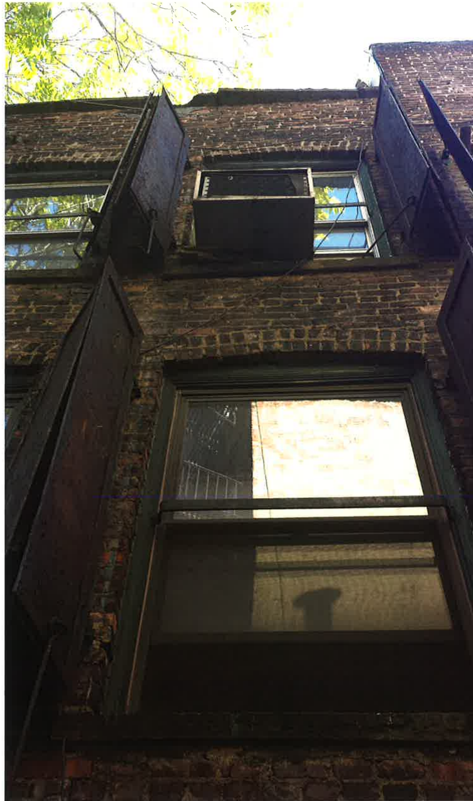
REAR OF THE BUILDING
