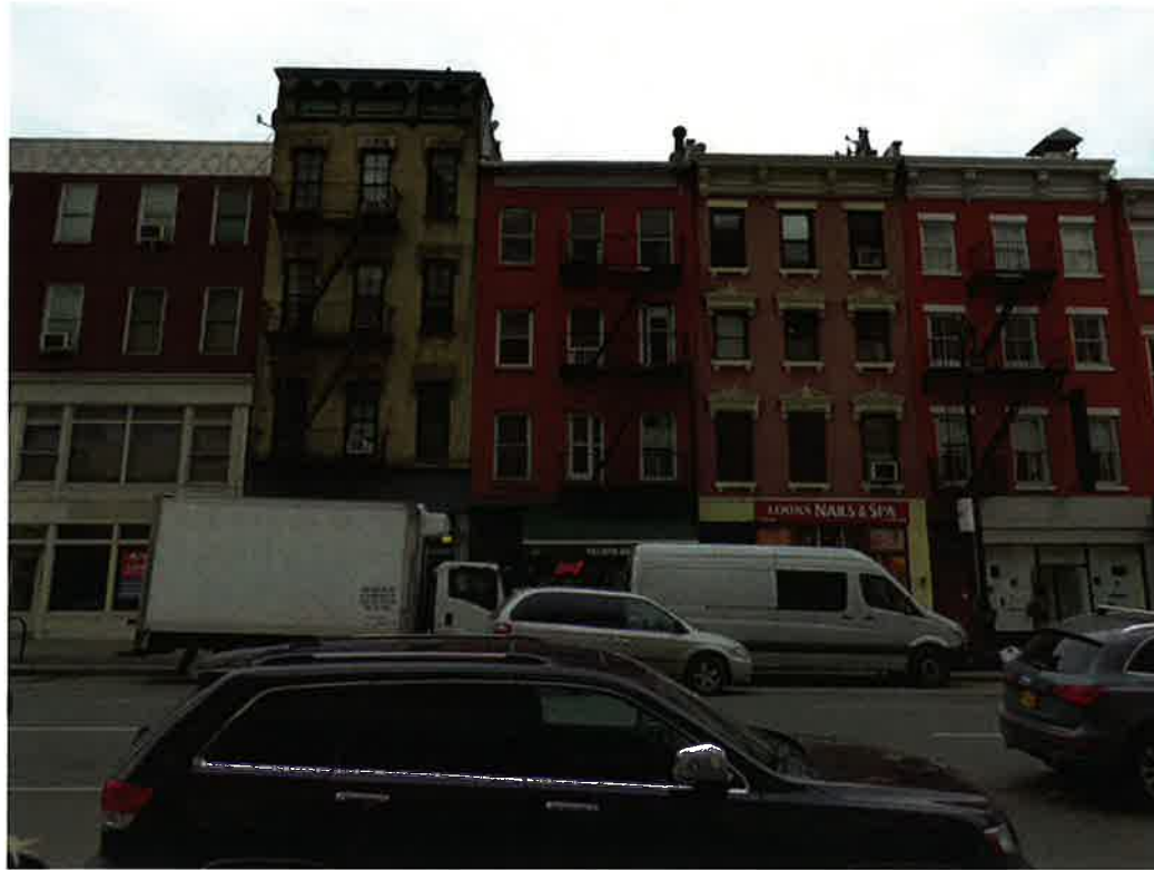
VIEW 1 - EXISTING CONDITION
