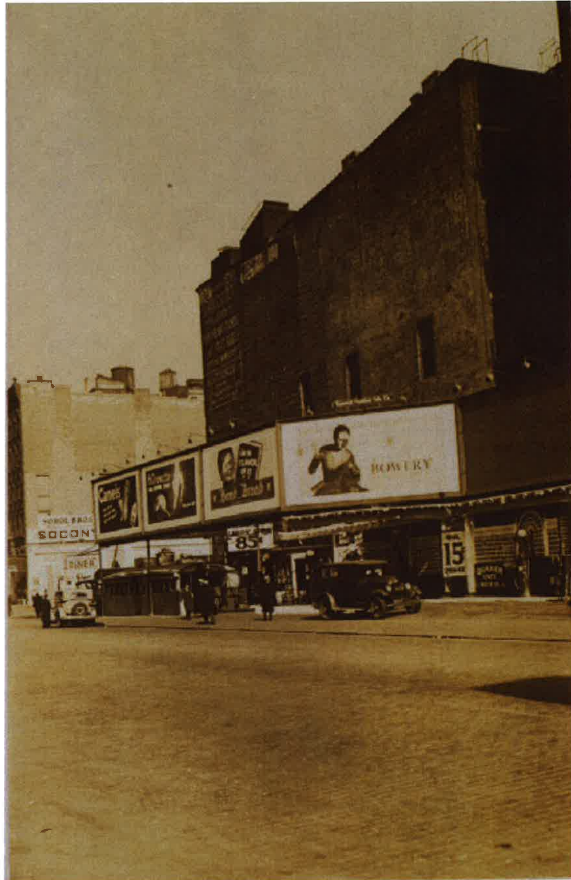
LAFAYETTE AND BOND LOOKING AT THE SITE - 1934
