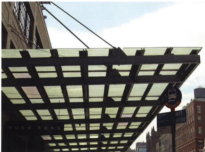
CANOPY WITH GLASS MATERIAL IN THE NEIGHBORHOOD - 401 W 14TH ST
