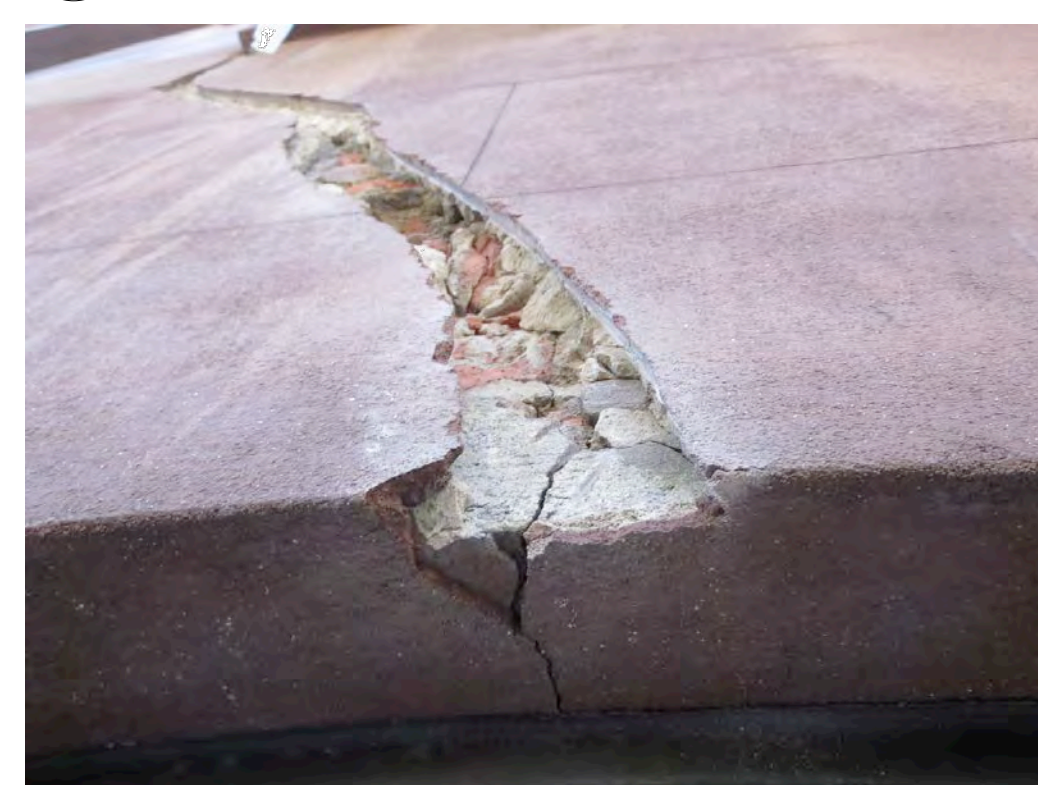
PH-7 PREVIOUS BRICK RECON. AT UNDERLYING MASONRY
