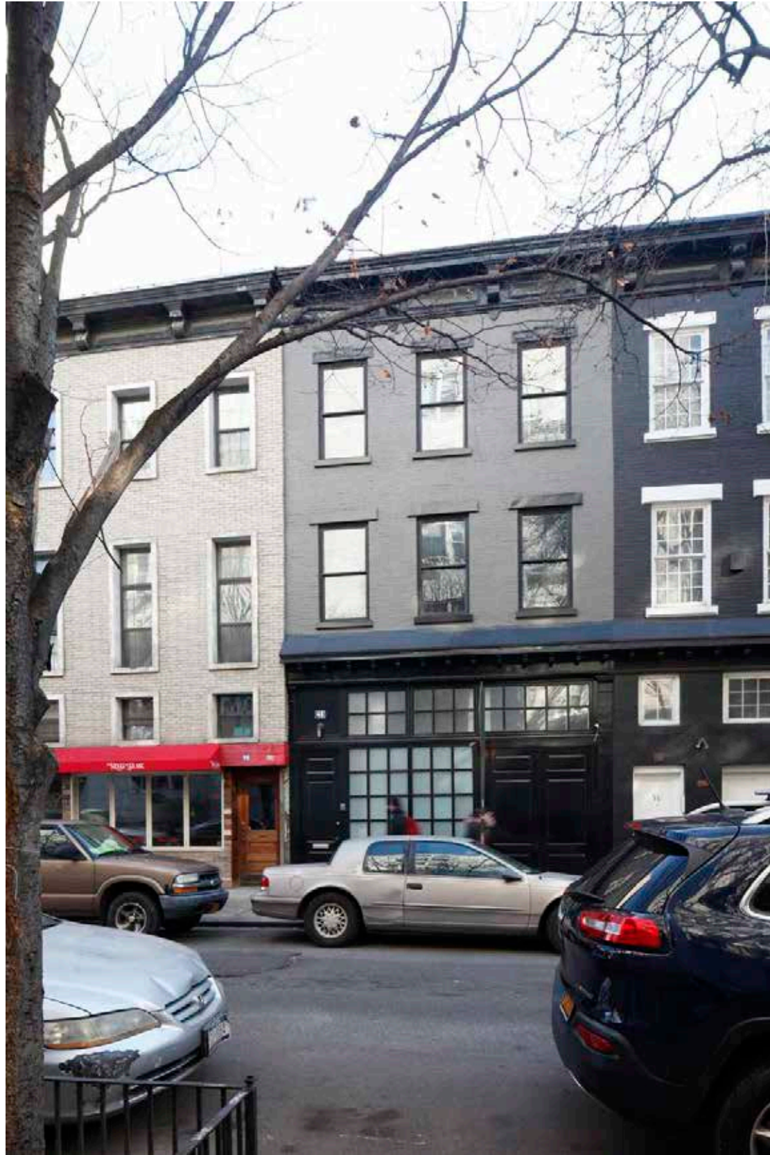
Designation Photo - November 2016 - Rooftop green wall removed for asbestos abatement
