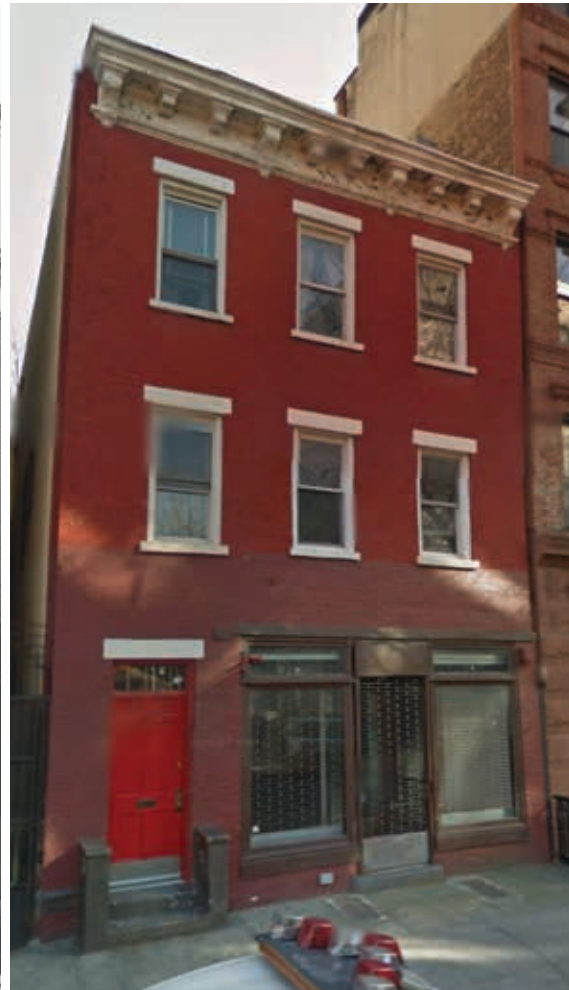
54 MacDougal St (Demolished)
