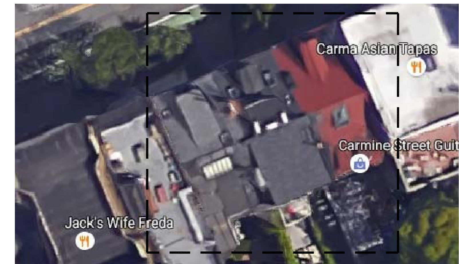
ARIEL VIEW OF SUBJECT PROPERTY W/ ADJACENT FEDERAL STYLE BUILDING ON CARMINE ST.
