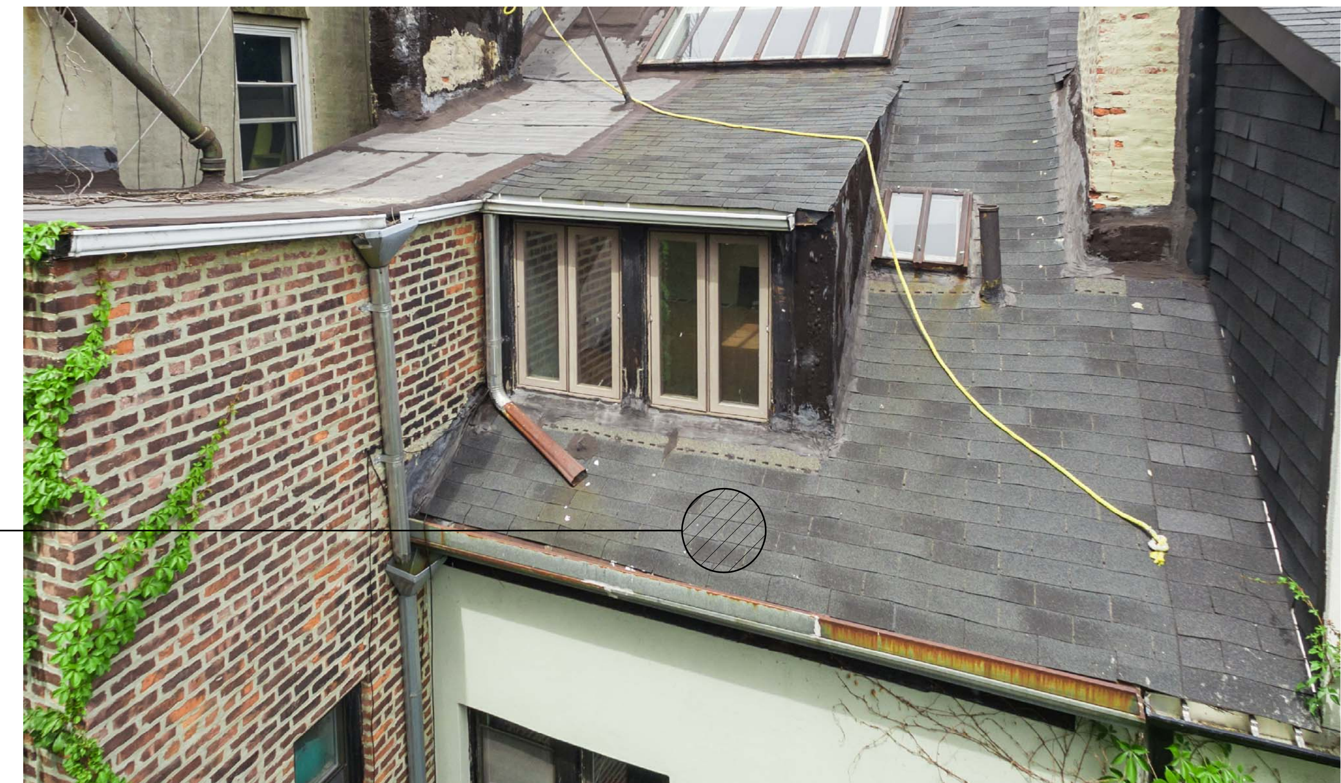
REAR ELEVATED VIEW OF SUBJECT PROPERTY SHOWING AREA OF WORK ON CARMINE ST.
