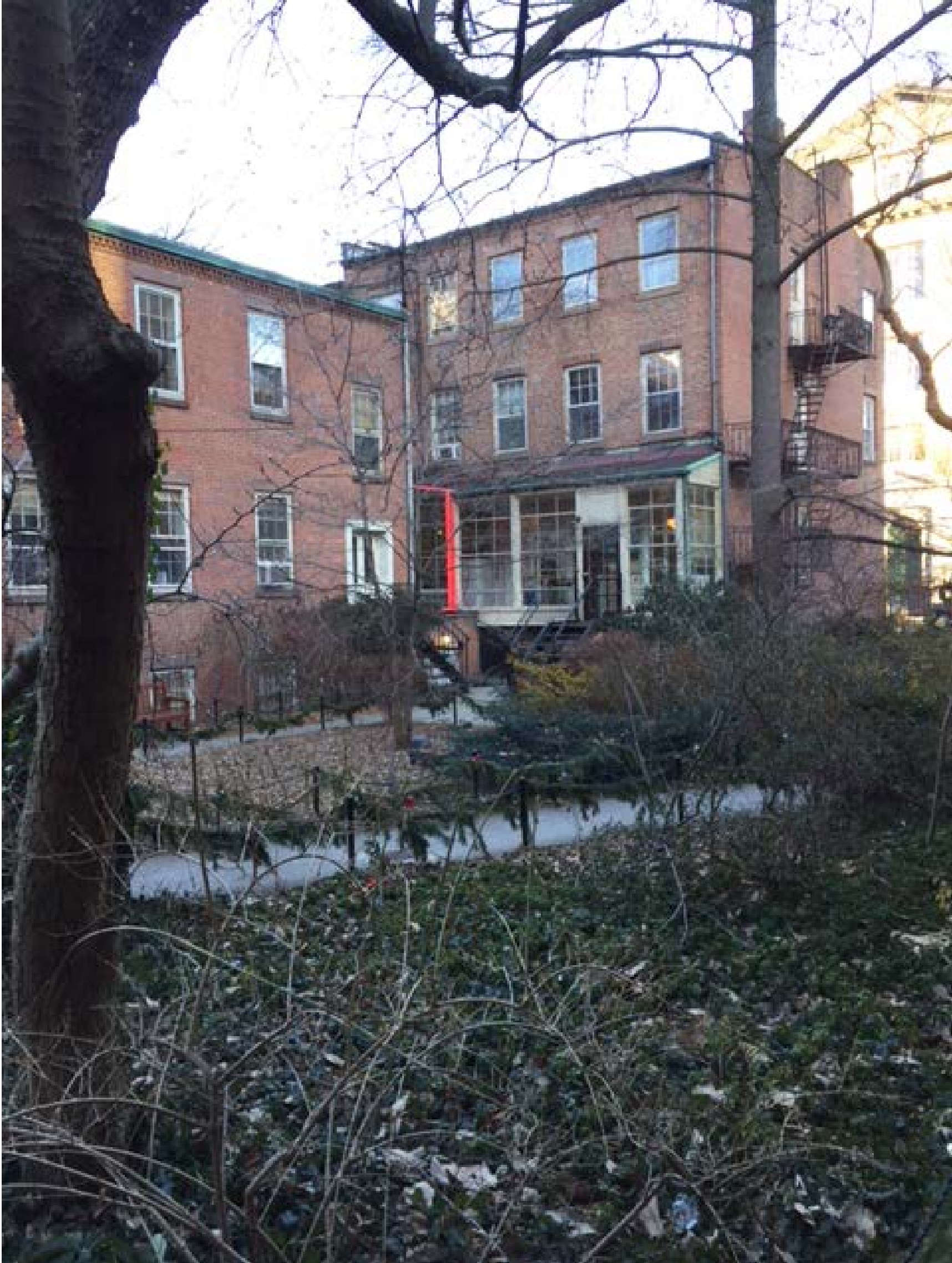
Mock Up Photograph: Porch/Annex addition. (Location of new structure shown in pink.) 8
