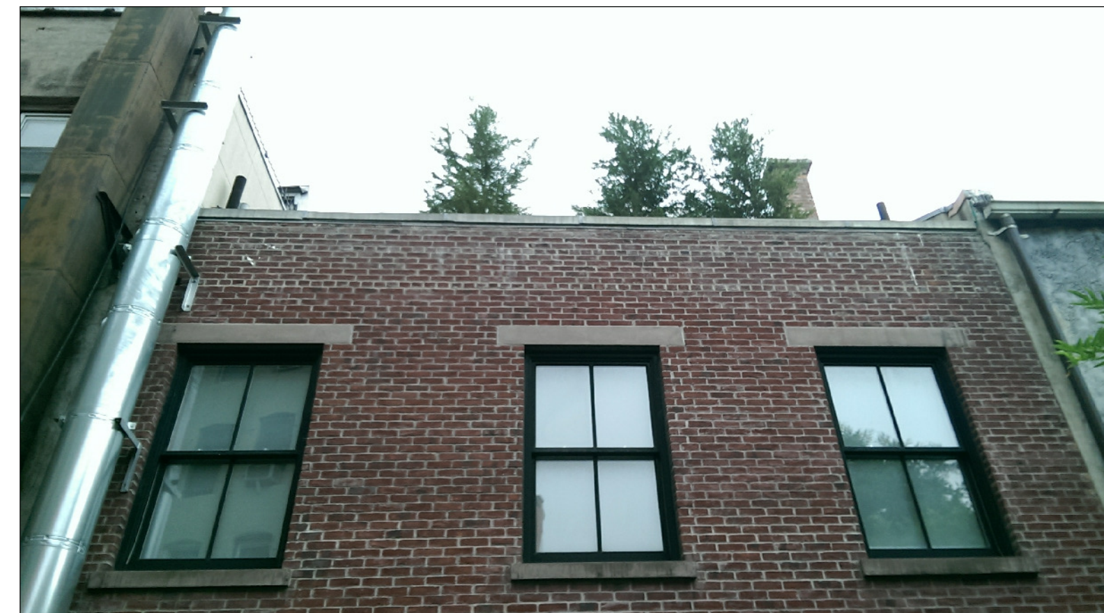
Existing rear 4th floor windows Scale : not to scale
