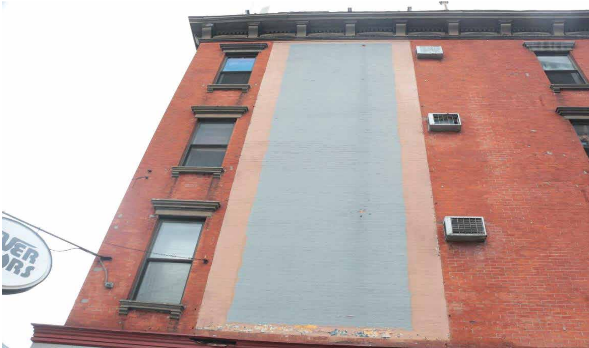
490 LaGuardia Place, existing painted wall sign
