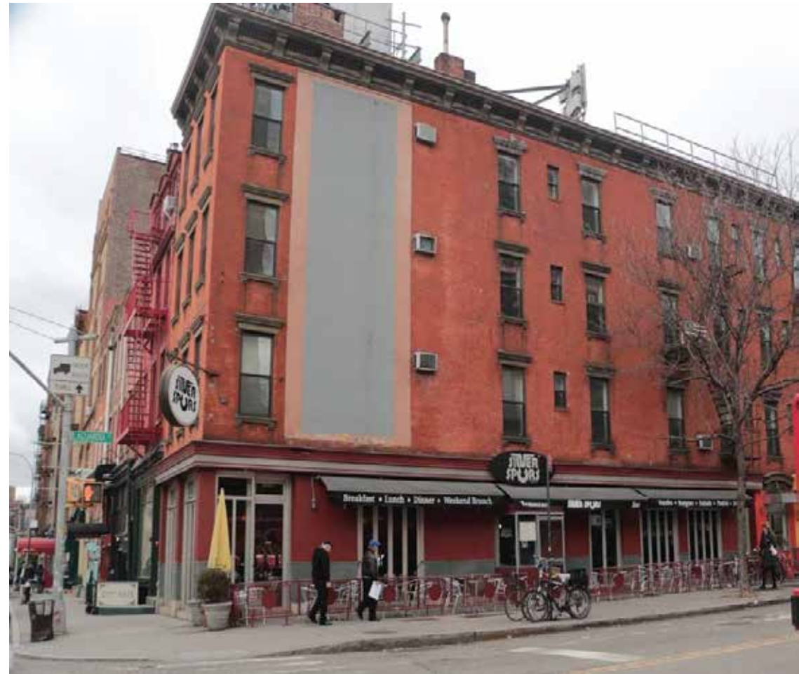
490 LaGuardia Place, viewed from the East side of LaGuardia Place
