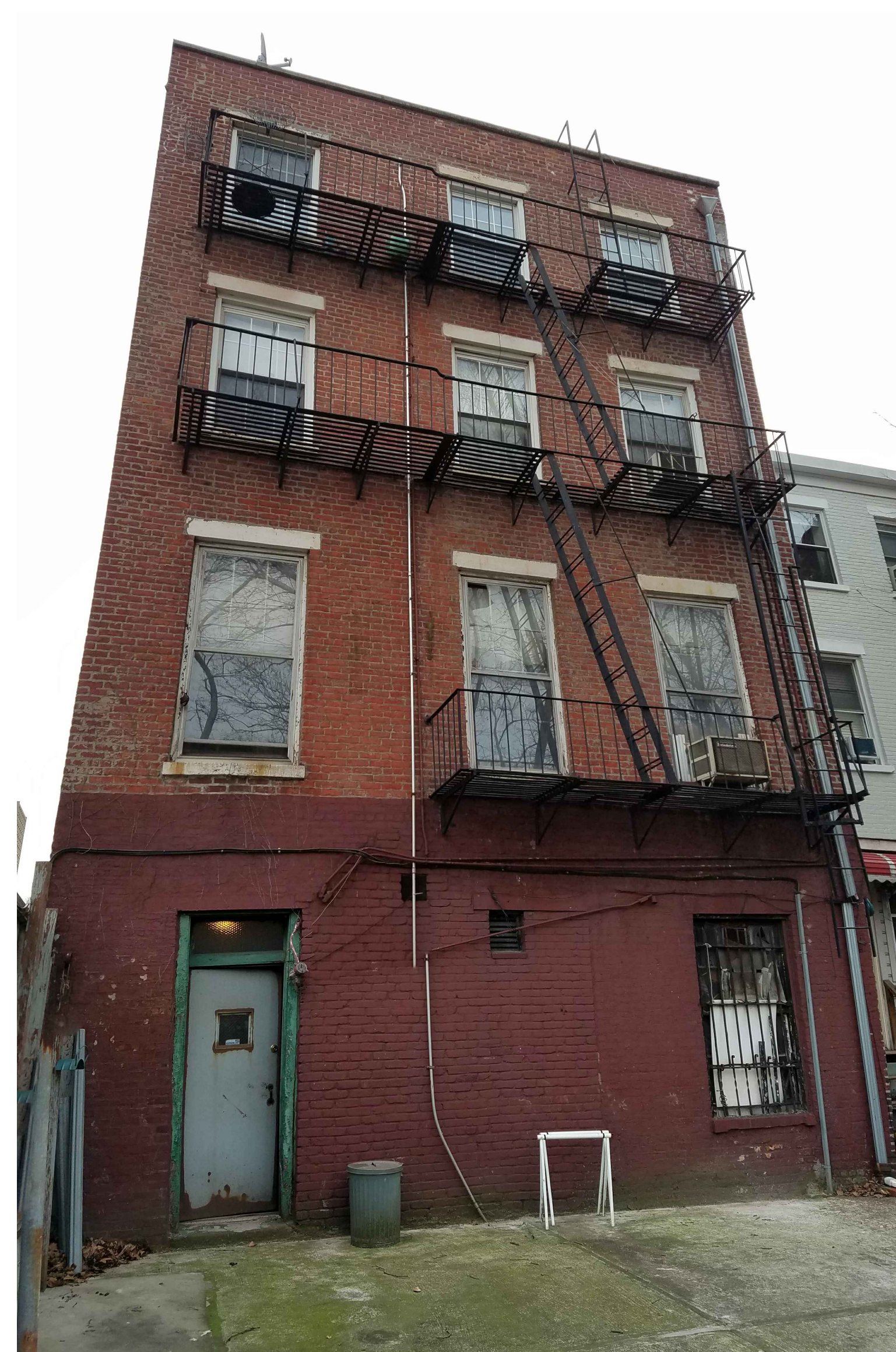
4 EXISTING BUILDING PHOTO
