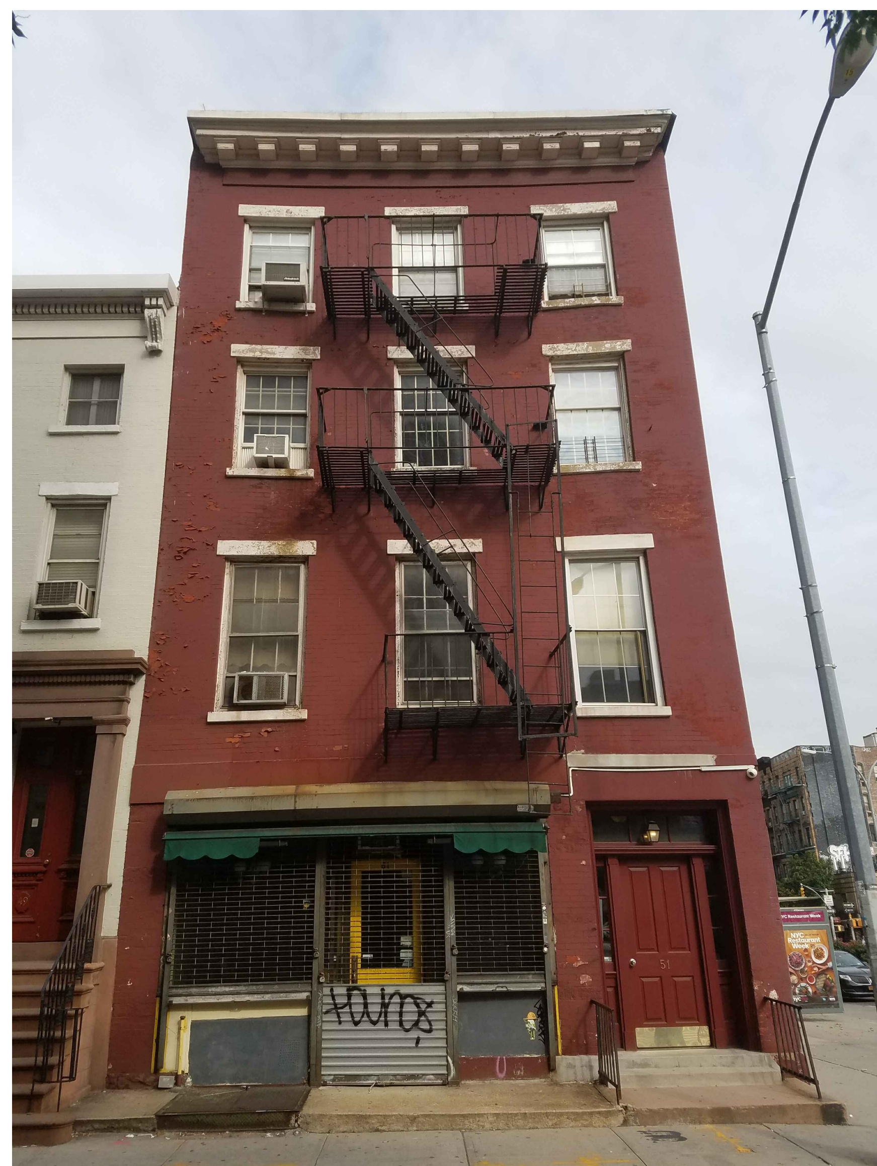
3 EXISTING BUILDING PHOTO
