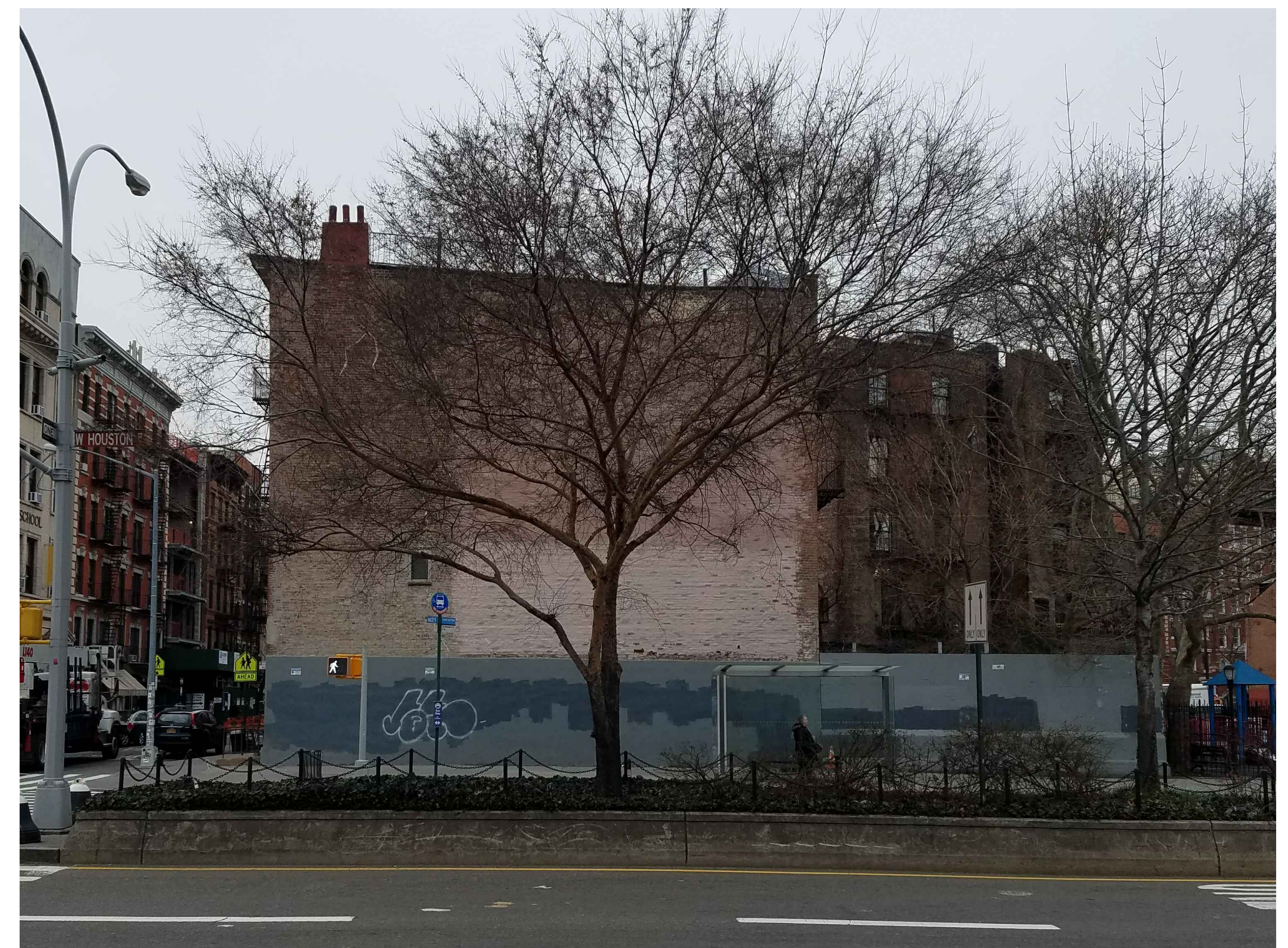
5 EXISTING BUILDING PHOTO
