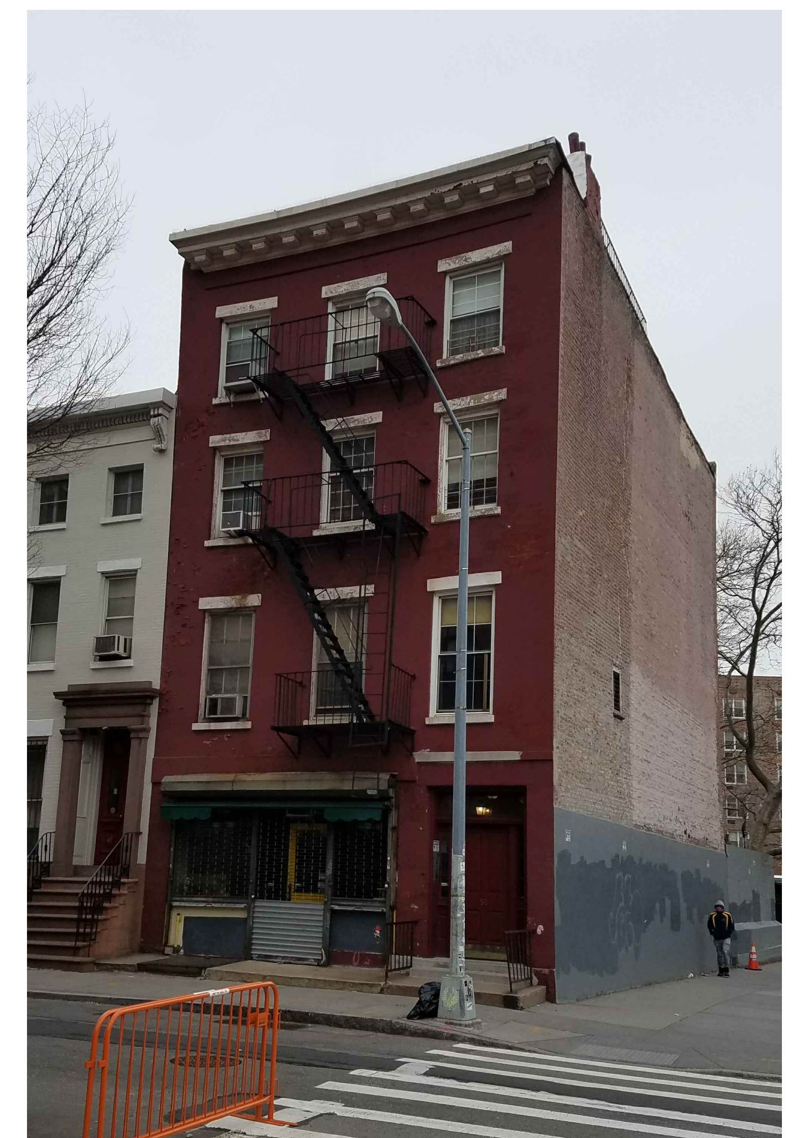
7 EXISTING BUILDING PHOTO
