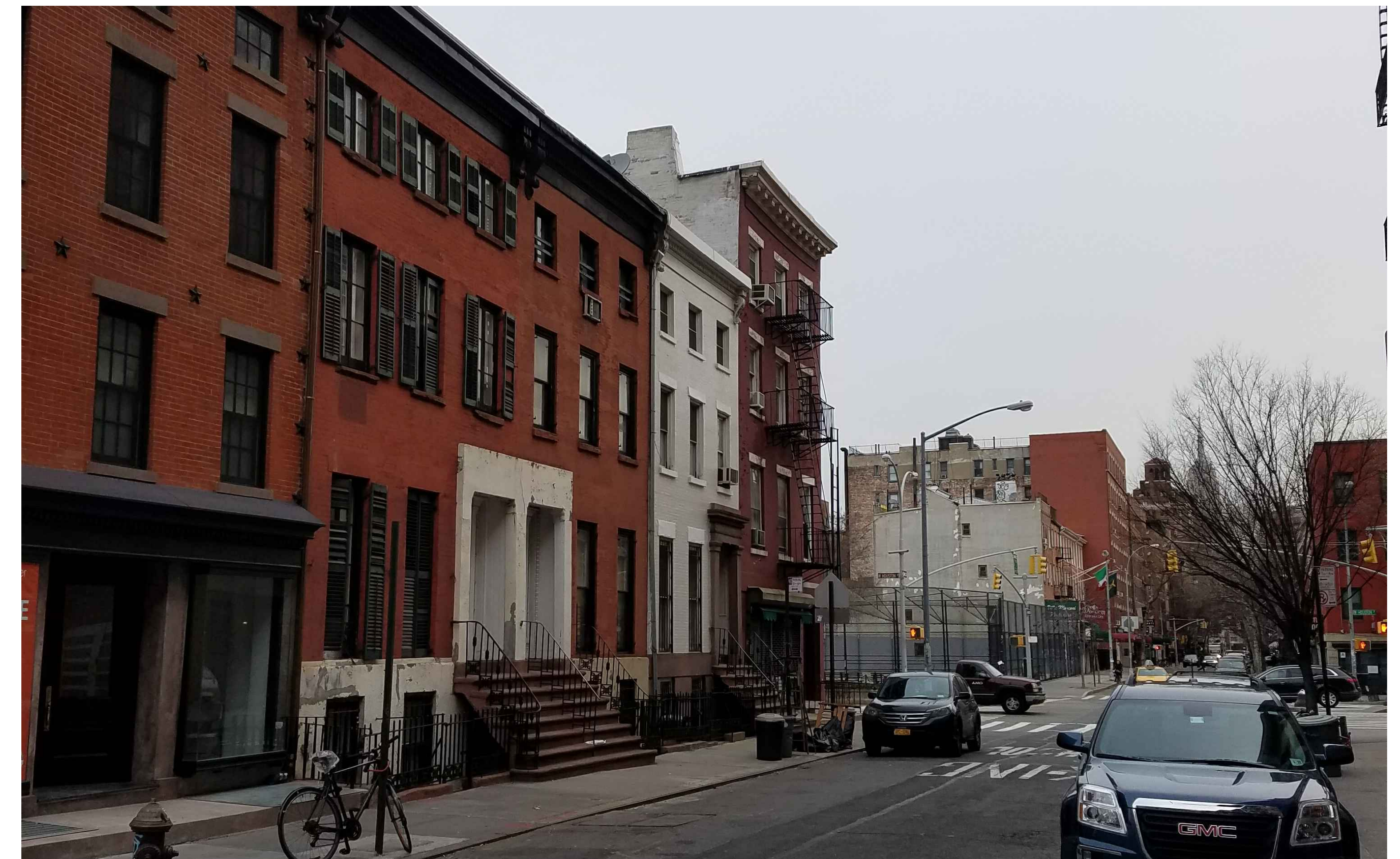
2 EXISTING BUILDING PHOTO
