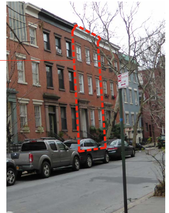
PHOTO OF EXISTING FRONT FACADE
