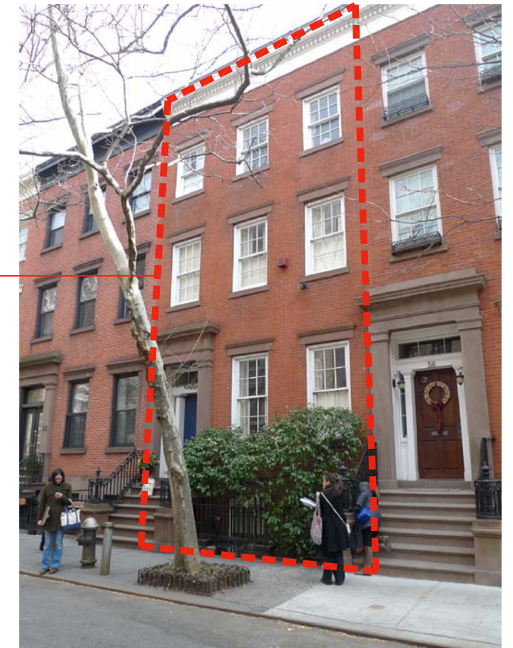
PHOTO OF EXISTING FRONT FACADE
