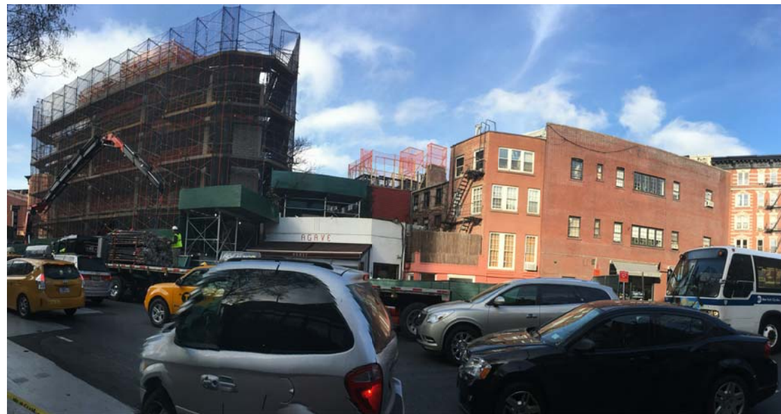
PHOTO 2: VIEW FROM EAST SIDE OF 7TH AVENUE
