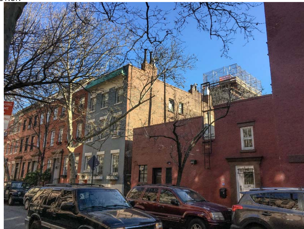
PHOTO 3: VIEW FROM 47 CHARLES STREET
