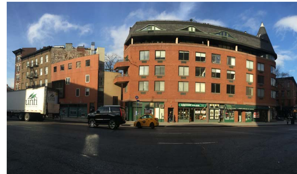
PHOTO 3: VIEW FROM EAST SIDE OF 7TH AVENUE
