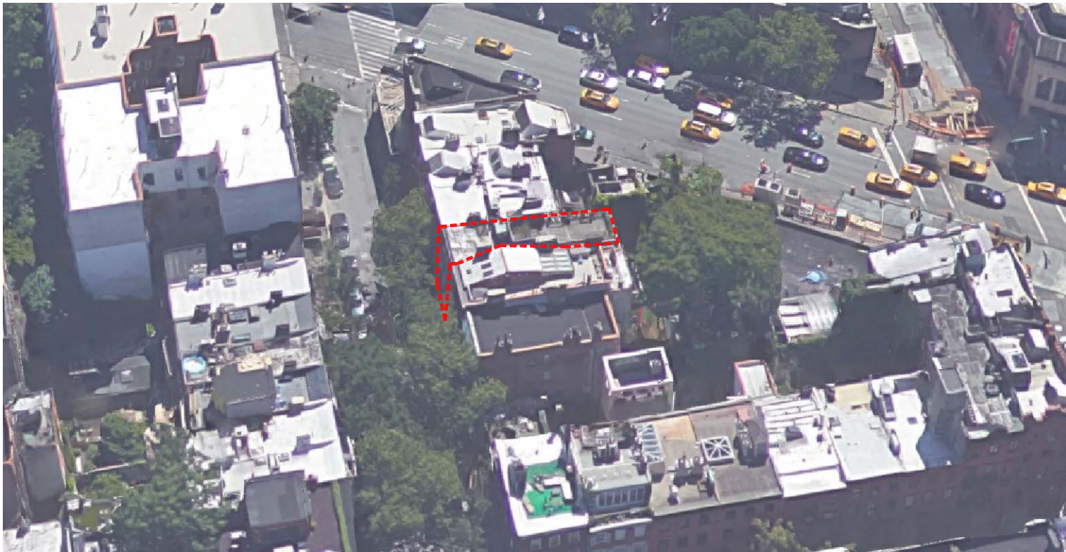
AERIAL VIEW- NORTH WEST
