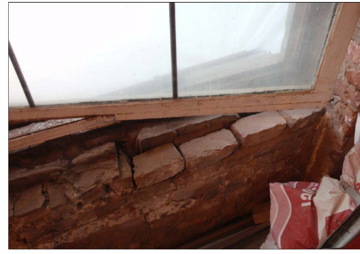
7 WINDOW SILL A-101 PHOTO
