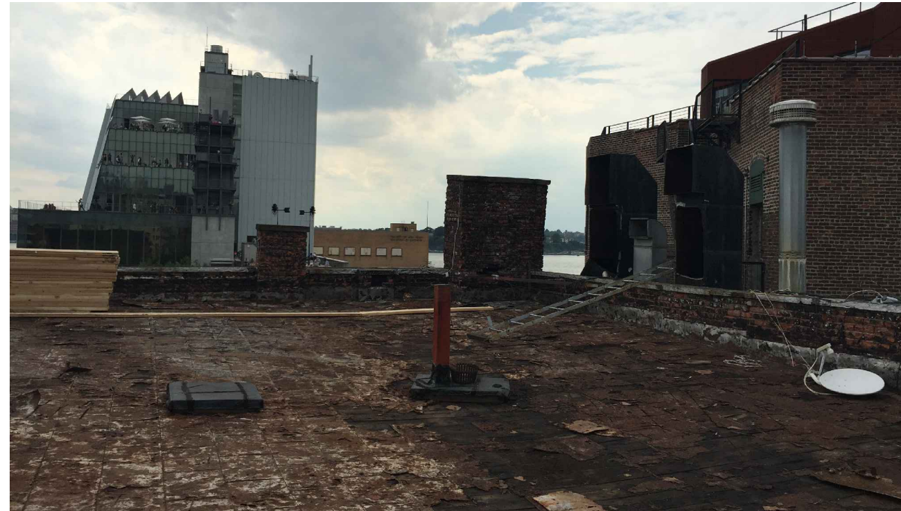
4 roof - view from east n.t.s. (soft demo for mock-up)
