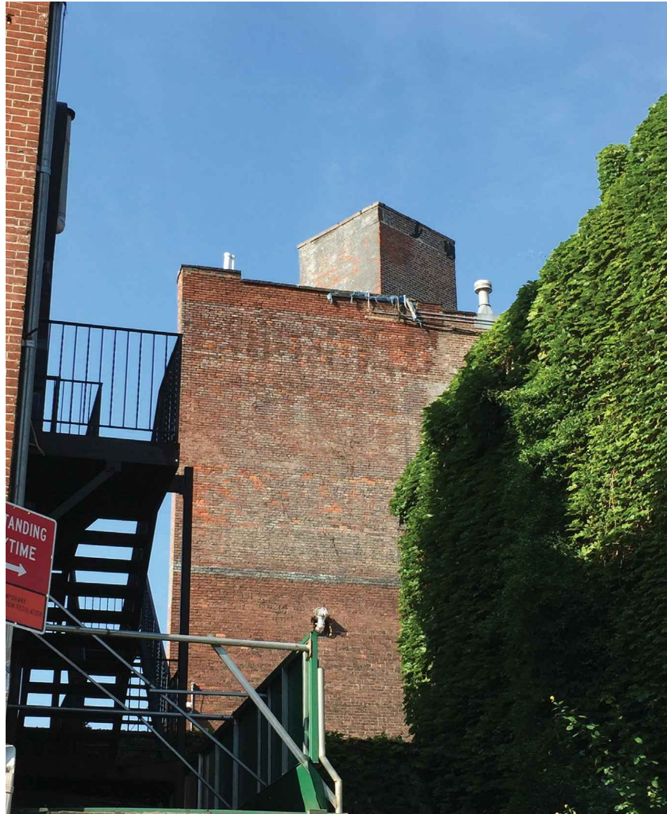
1 existing view of east corner from little w 12th st n.t.s.
