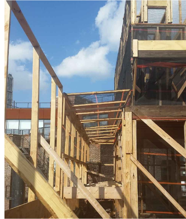
3 along west face side of bldg, looking north n.t.s.
