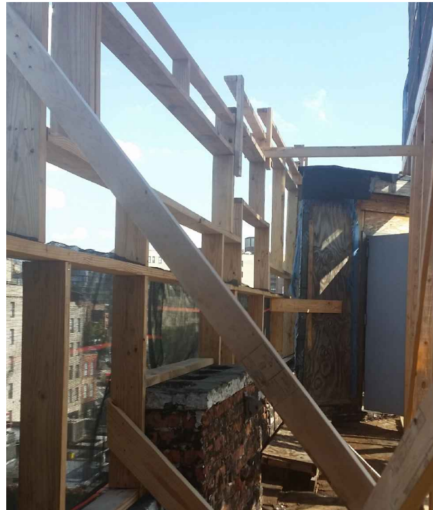
5 along north west side, looking east n.t.s.
