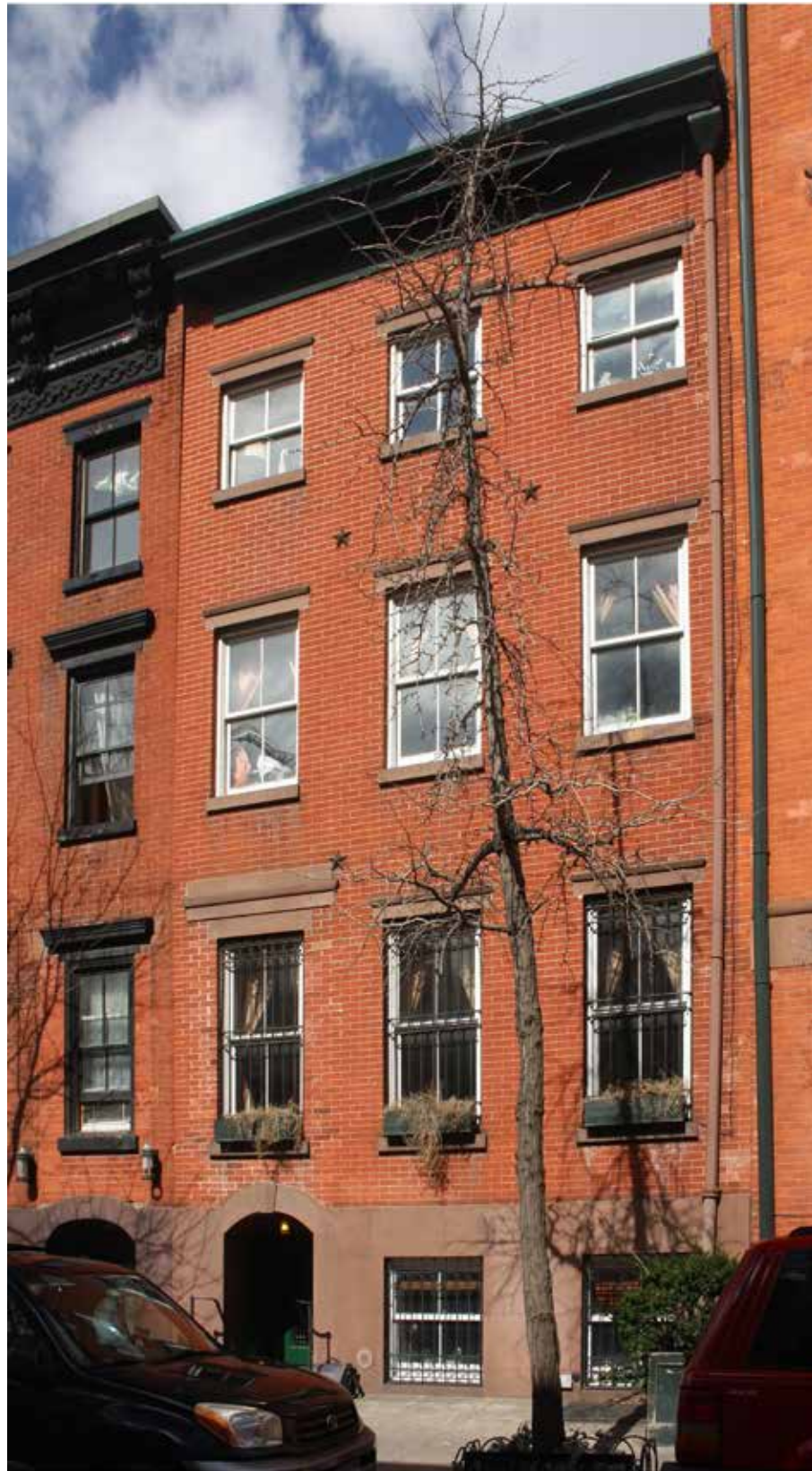
Existing Front Facade
