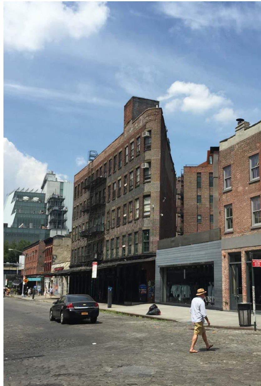
1 existing view from gansevoort st at 9th ave n.t.s.
