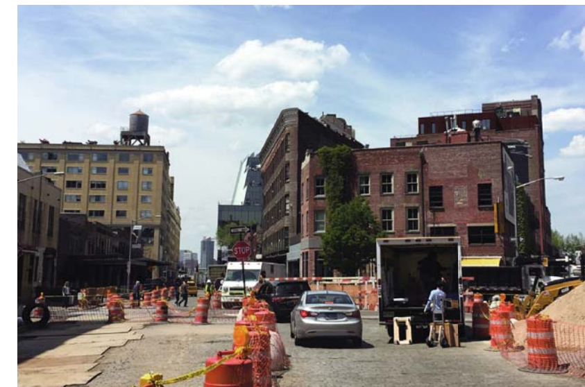
4 proposed rendering from gansevoort st between 9th ave and hudson st n.t.s.
