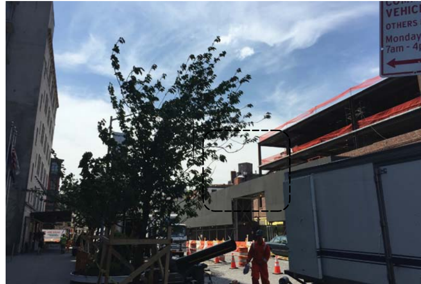
2 existing view from 9th ave between little w 12th st and w 13th st n.t.s.
