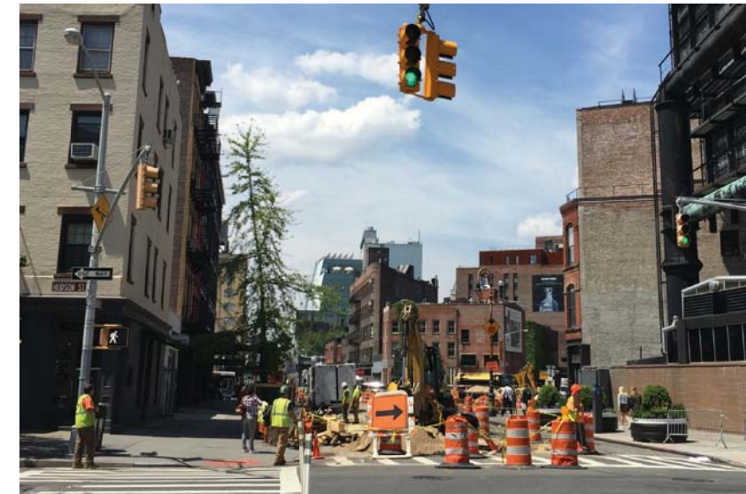
3 existing view from gansevoort st at 9th ave n.t.s.
