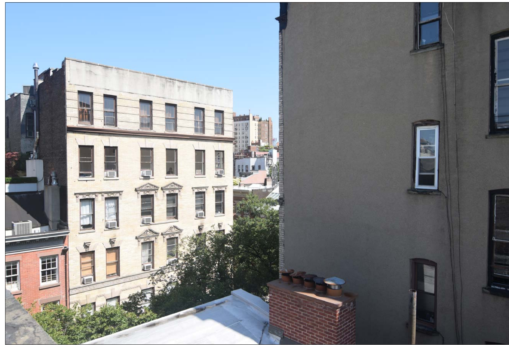
2 51 BANK - 6 STOREY BUILDING TO THE NORTHEAST
