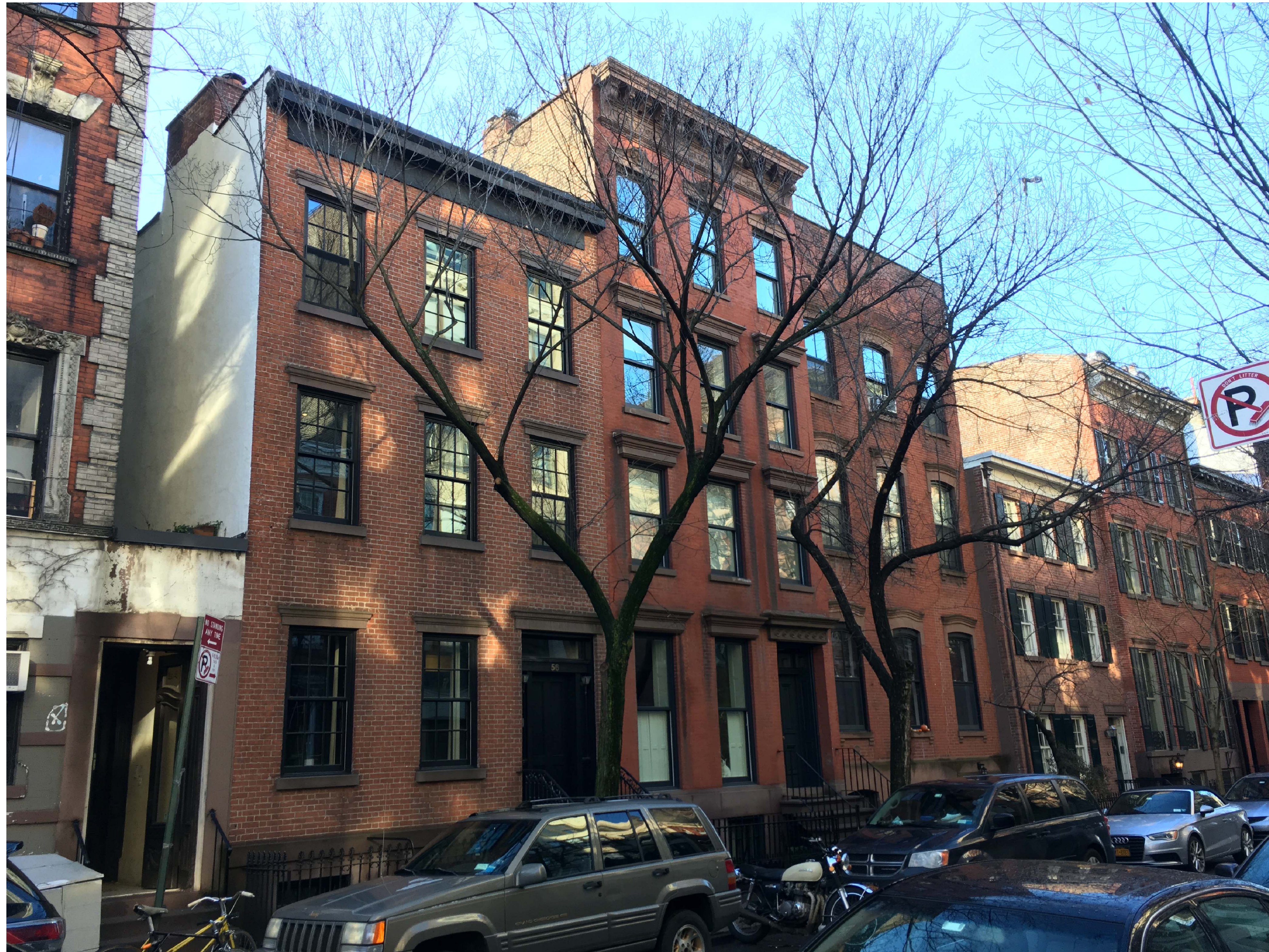
1 CURRENT SITE PHOTOGRAPH - 58 BANK STREET LOOKING SOUTHWEST
