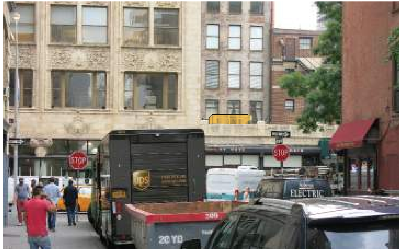
1A. CURRENTLY PROPOSED VIEW NORTH FROM CROSBY STREET. MECHANICAL EQUIPMENT IS VISIBLE.
