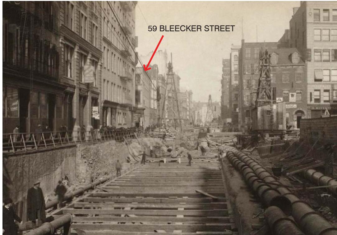
1901 CONSTRUCTION OF SUBWAY BENEATH LAFAYETTE STREET VIEW NORTH FROM E. HOUSTON STREET (NYPL)
