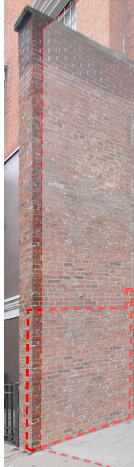
WING WALLS: NEWER BRICK AND CEMENTIOUS INFILL TO BE REPLACED TO MATCH HISTORIC BRICK
