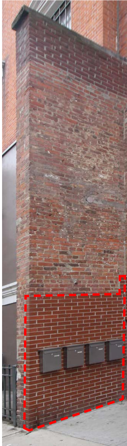
WING WALLS: NEWER BRICK AND CEMENTIOUS INFILL TO BE REPLACED TO MATCH HISTORIC BRICK
