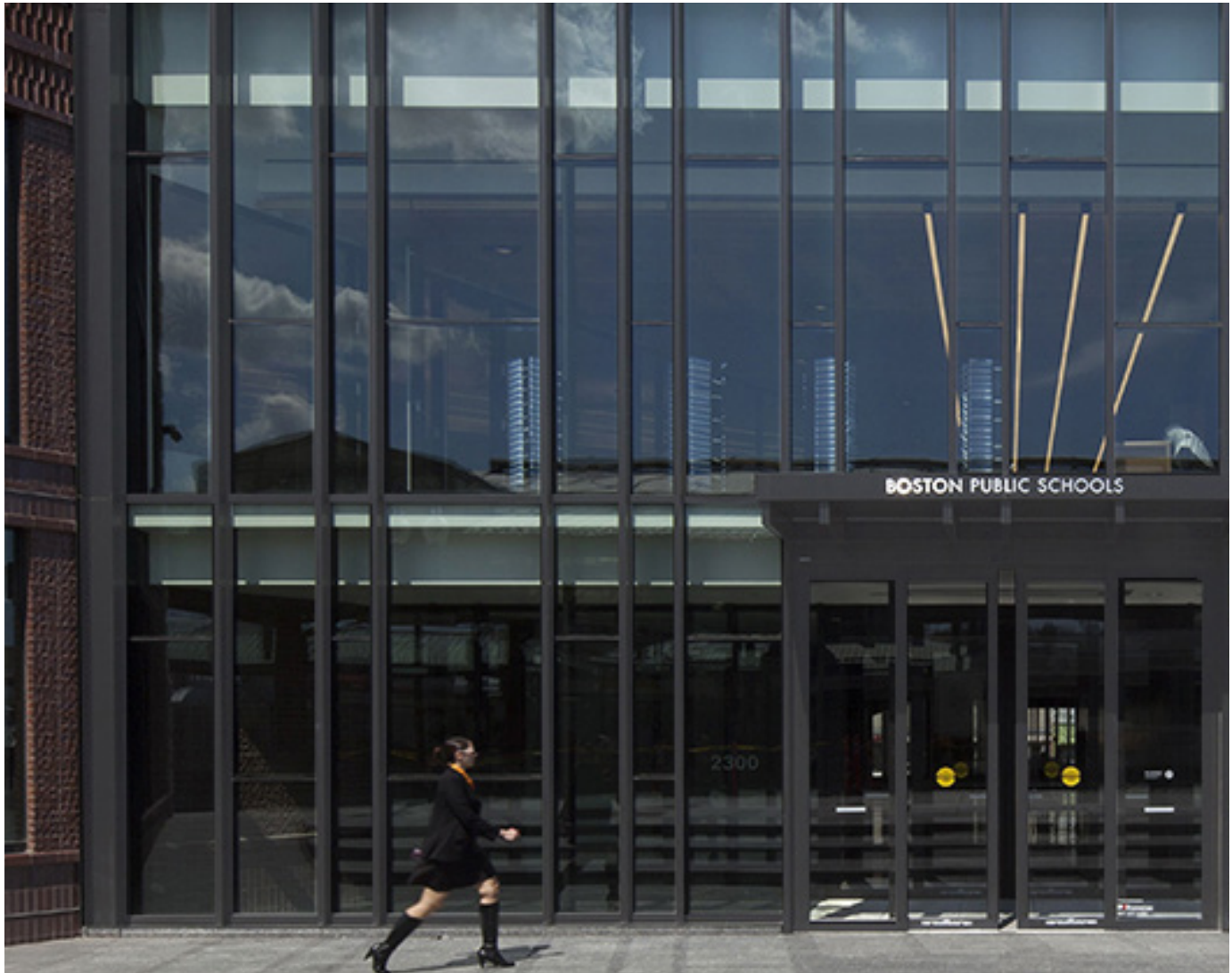
NEW STOREFRONT: STEEL MULLIONS WITH RECESSED GLAZING
