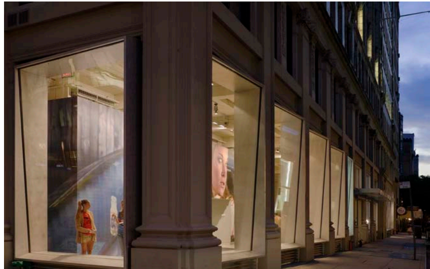
NEW STOREFRONT: ALUMINUM MULLIONS MATTE FINISH WITH RECESSED GLAZING
