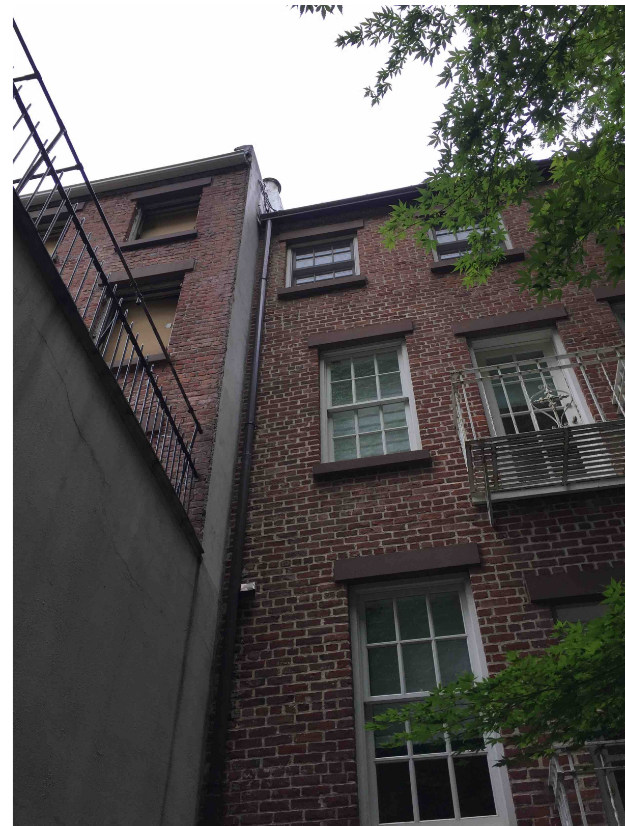
4 VIEW OF REAR FACADE FROM GARDEN c. JUNE 2017 NTS
