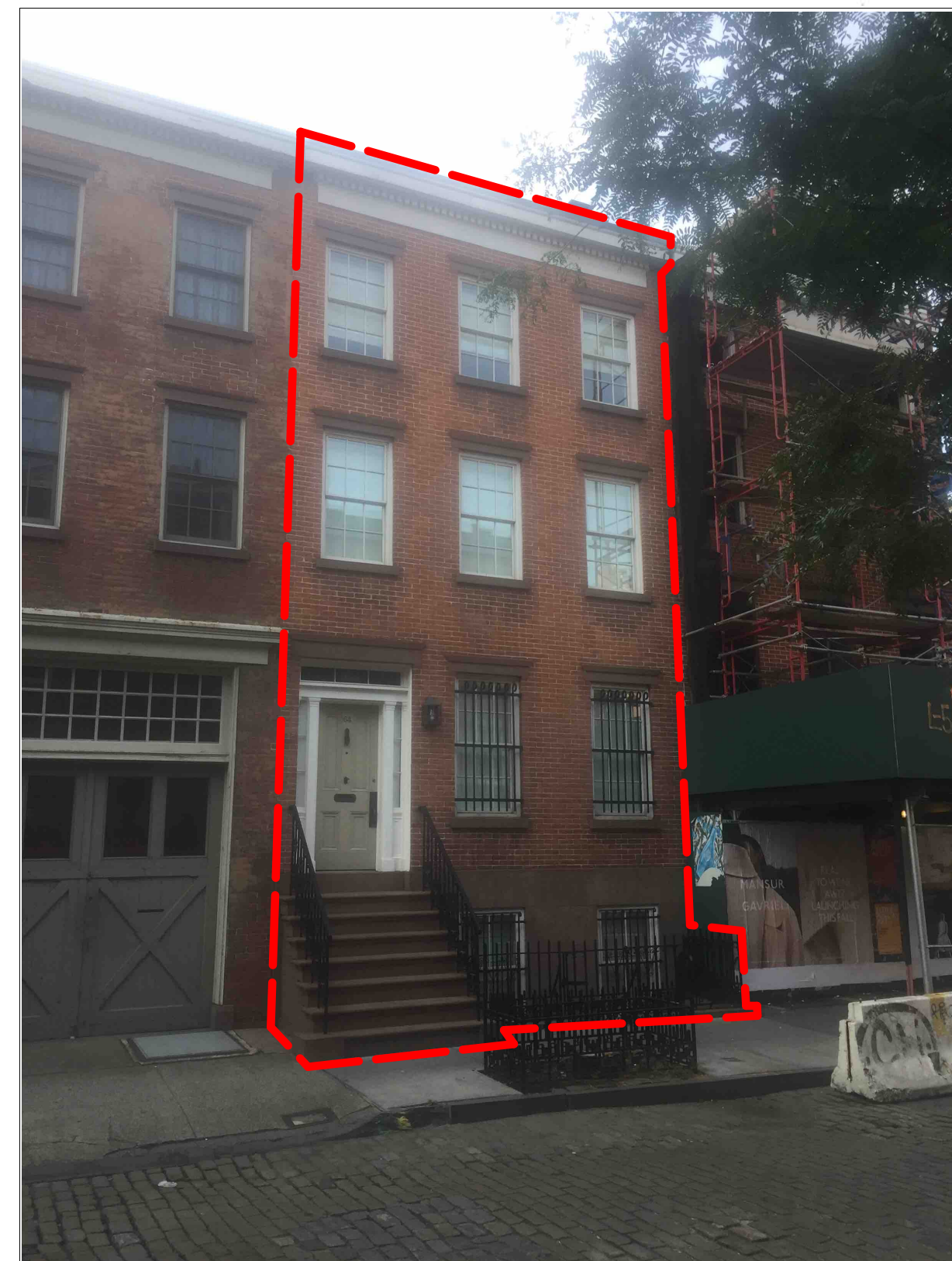
6 VIEW OF HORATIO STREET FAÇADE c. JUNE 2017 NTS
