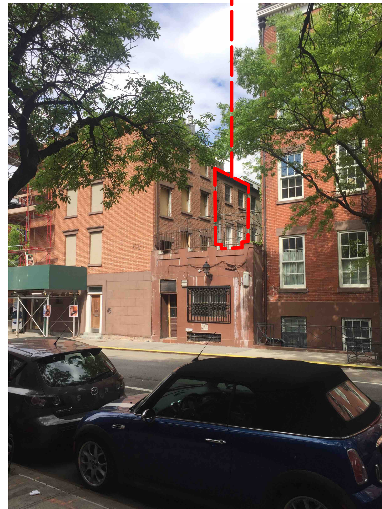
2 VIEW OF REAR FACADE FROM GREENWICH STREET c. JUNE 2017 NTS
