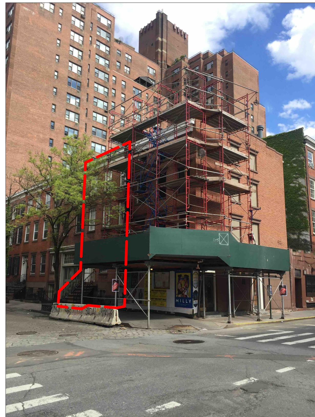
7 VIEW OF HORATIO STREET FAÇADE c. JUNE 2017 NTS
