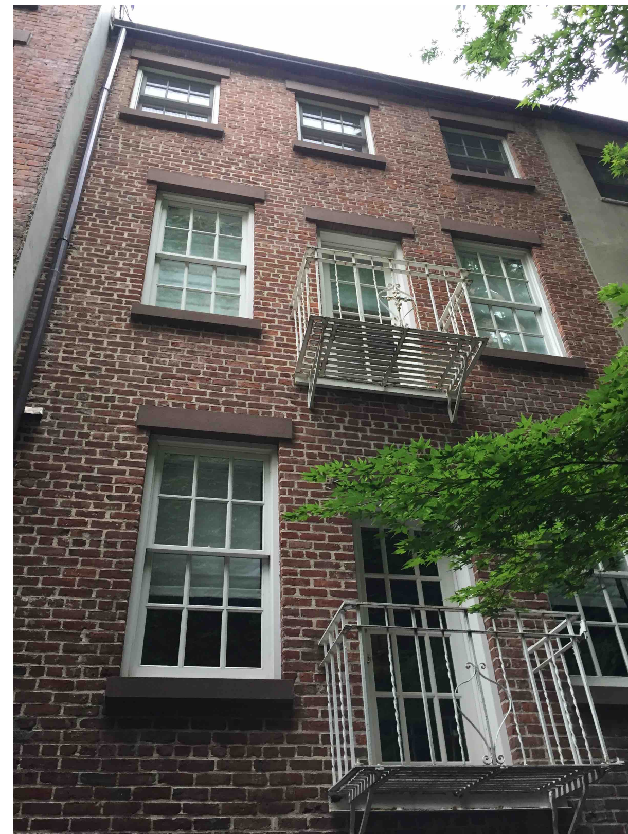
3 VIEW OF REAR FACADE FROM GARDEN c. JUNE 2017 NTS
