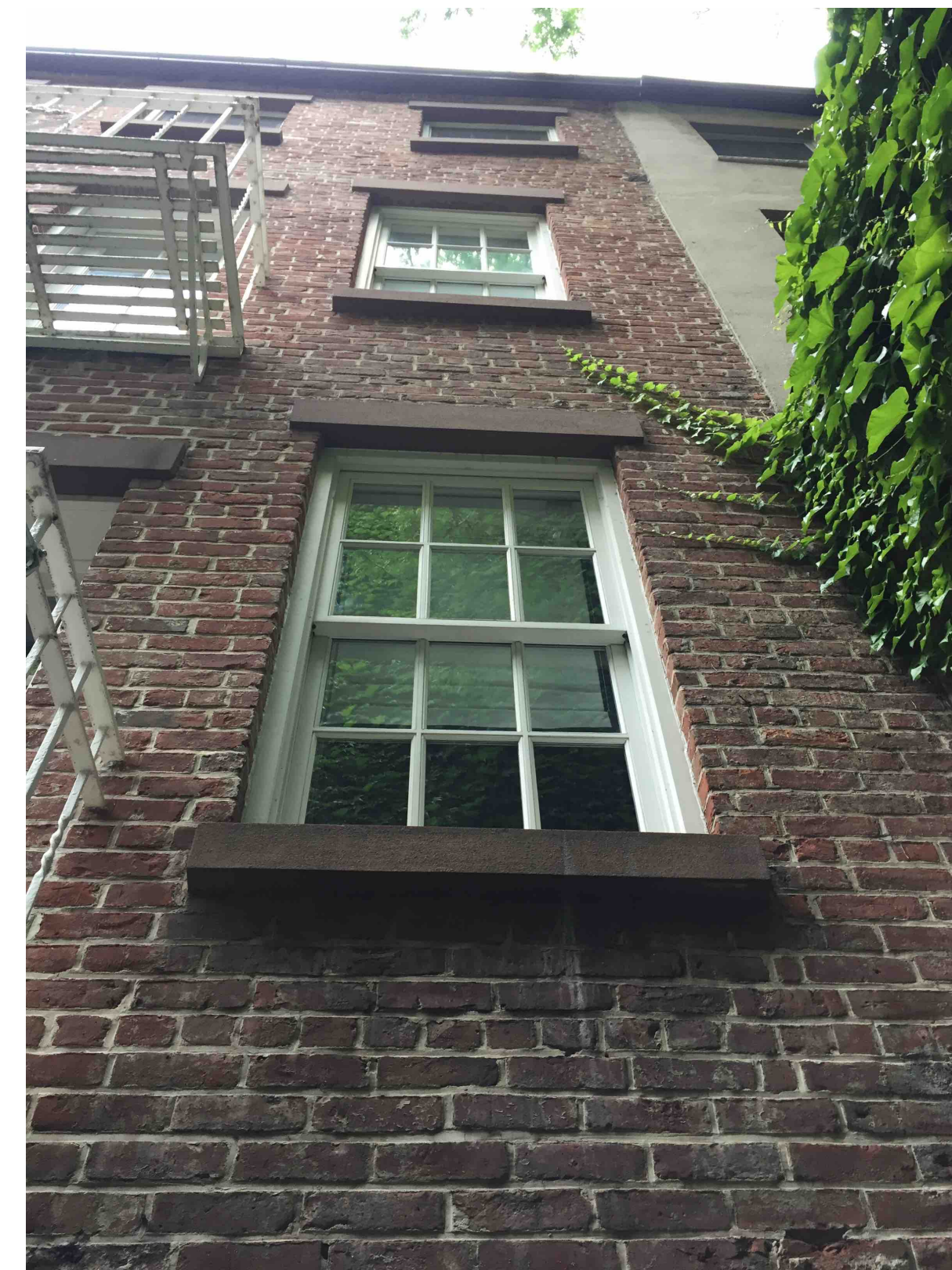
2 VIEW OF REAR FACADE FROM GARDEN c. JUNE 2017 NTS
