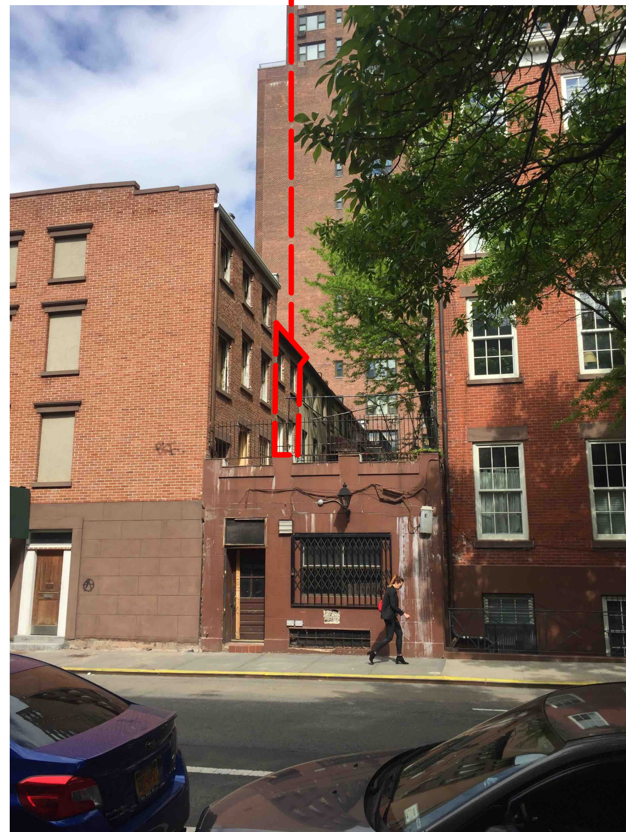
3 VIEW OF REAR FACADE FROM GREENWICH STREET c. JUNE 2017 NTS
