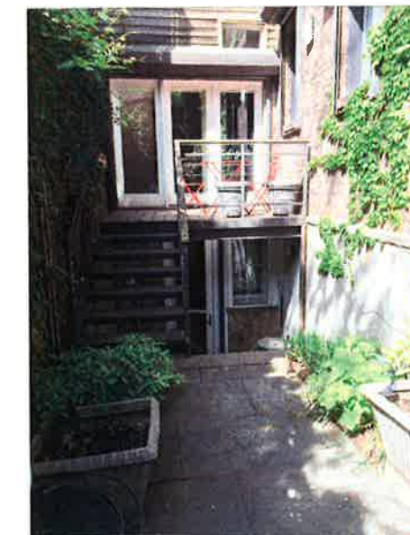
5 REAR DECK - #66 EXISTING
