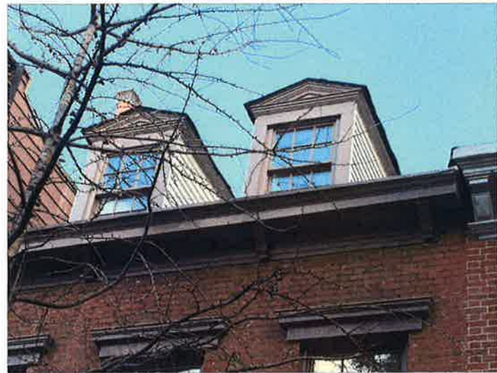
3 66 BEDFORD STREET - existing dormers Scale: none
