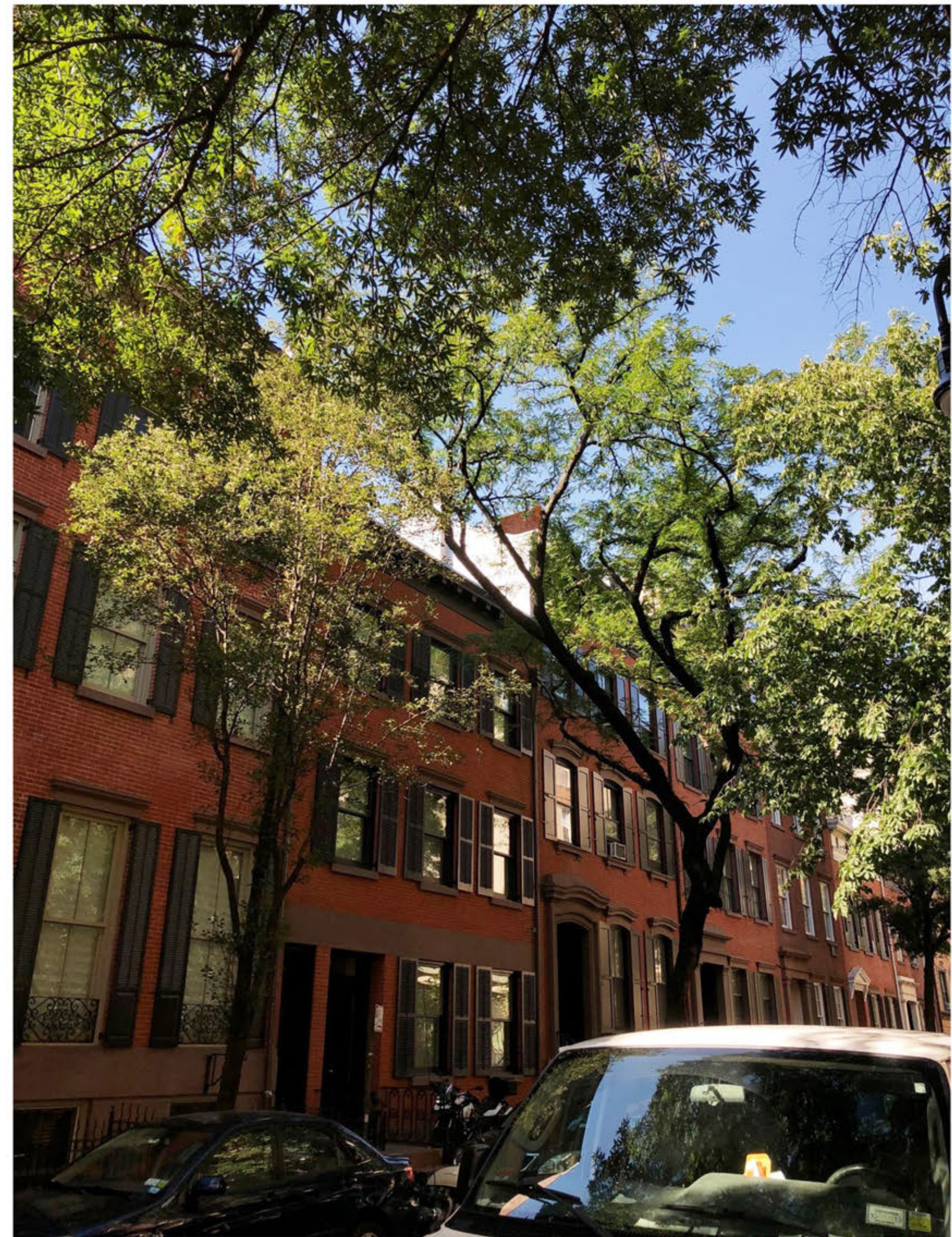
EXISTING CONDITION - LOOKING SOUTH FROM BANK STREET
