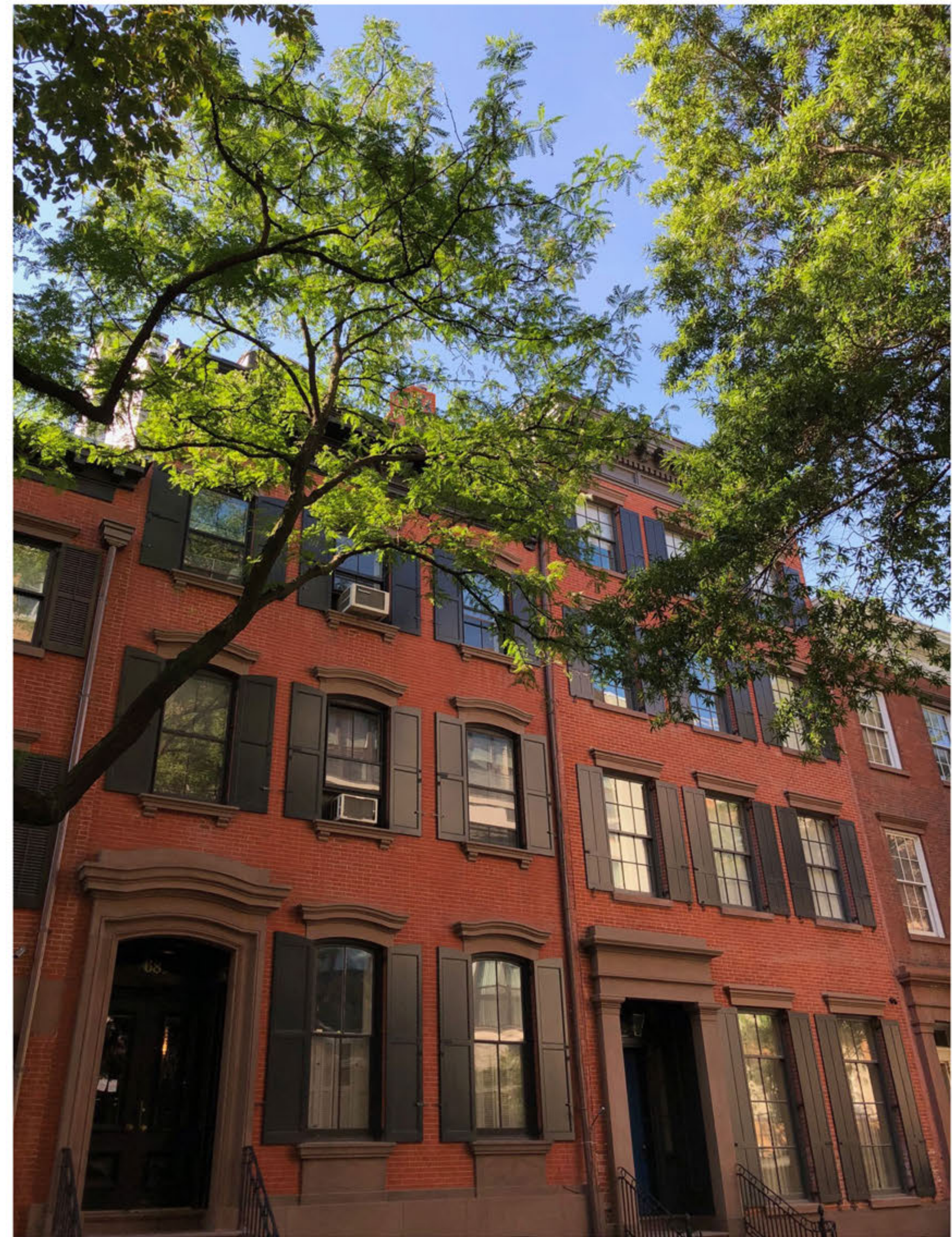
EXISTING CONDITION - LOOKING SOUTH FROM BANK STREET
