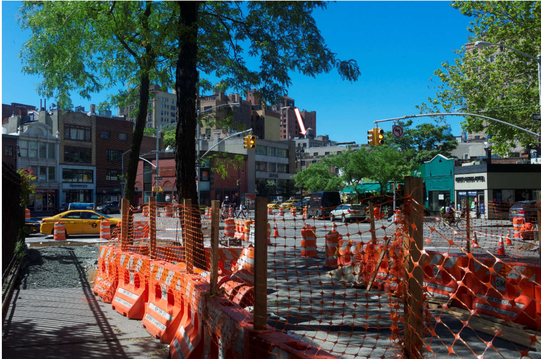
Photograph 6. Taken from the north side of Greenwich Avenue between West 9 th Street and West 10 th Street, looking southeast along Greenwich Avenue. The cooling tower at 79 Washington Place occupies a space in the field of view that is many times smaller than that of the overhead traffic signals as a percentage of the overall field of view.
