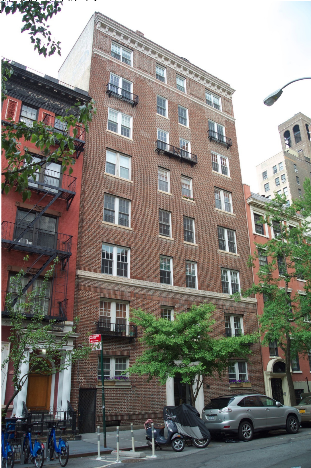
Photograph 1: Taken from the south side of Washington Place between Sixth Avenue and MacDougal Street, looking northeast. 79 Washington Place is the eight-story red brick building at center. The cooling tower at 79 Washington Place is not visible from Washington Place.
