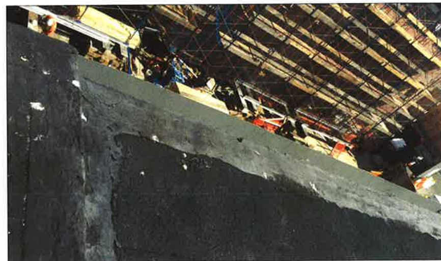
EXISTING FRONT PARAPET @ 12LW12
