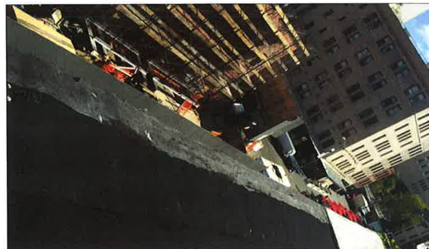
EXISTING FRONT PARAPET @ 8&10LW12
