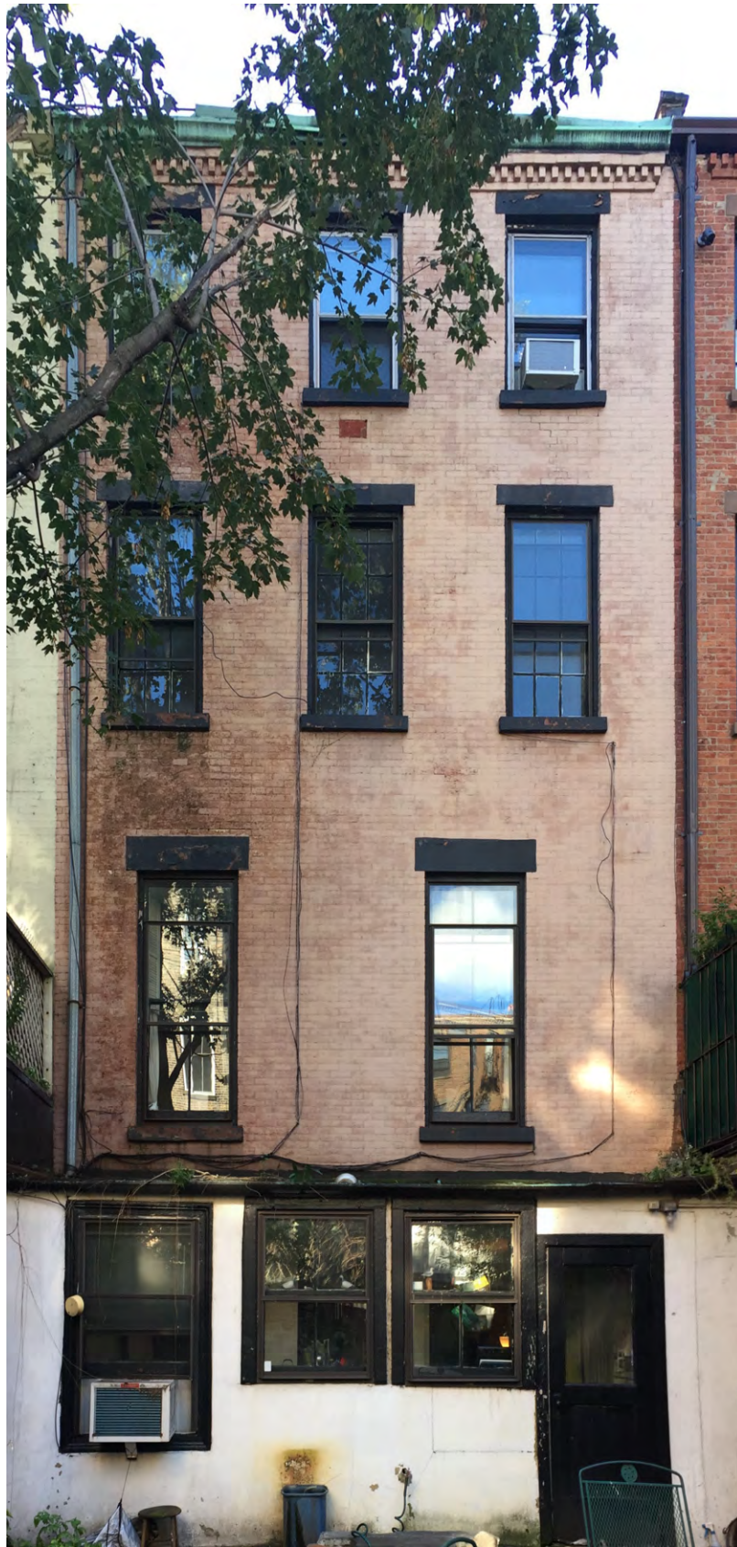
EXISTING REAR FACADE
