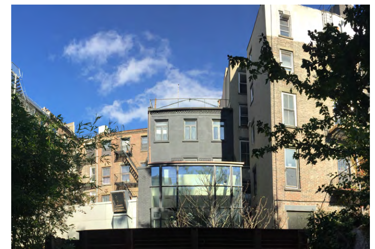
FACADES OPPOSITE (NORTH) OF PROPERTY
