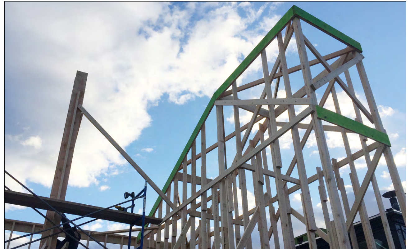
81 CHARLES ST - MOCK UP - ROOF VIEW 2 (LOOKING SOUTH @ STAIR BULKHEAD)
