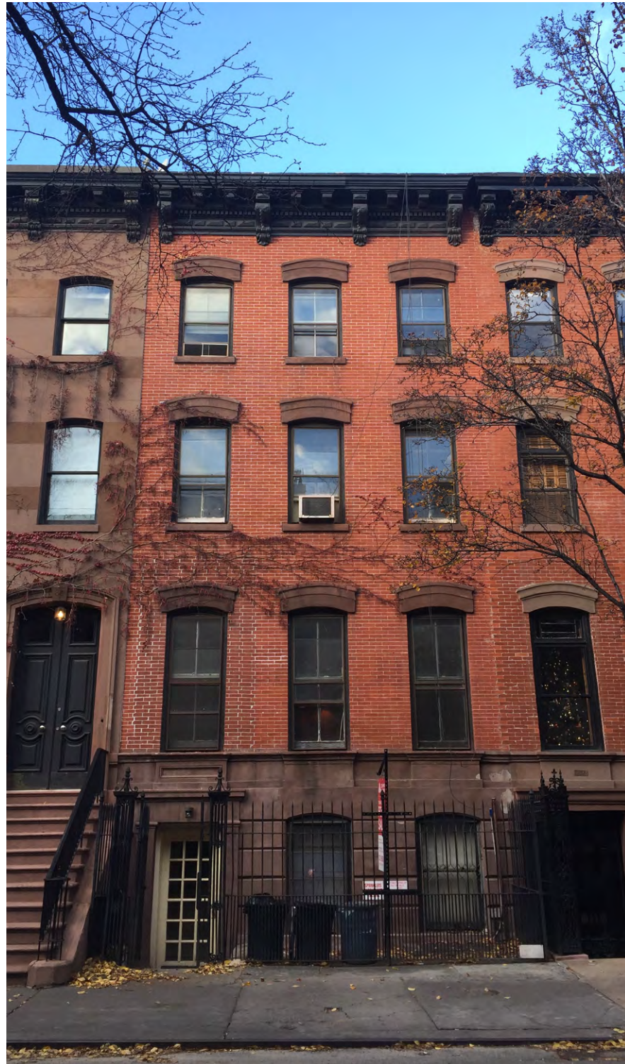
CURRENT FRONT FACADE
