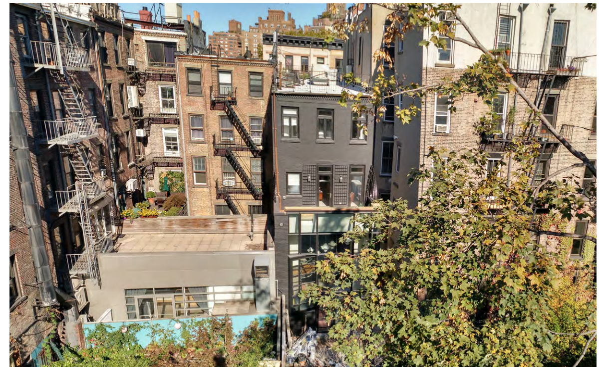
FACADES OF THE INSIDE OF THE BLOCK (NORTH)
