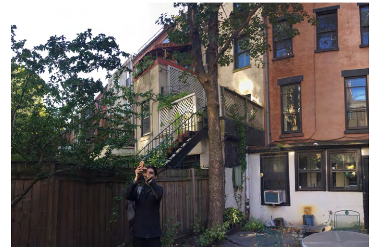
NEIGHBORS ADJACENT REAR FACADES (EAST)
