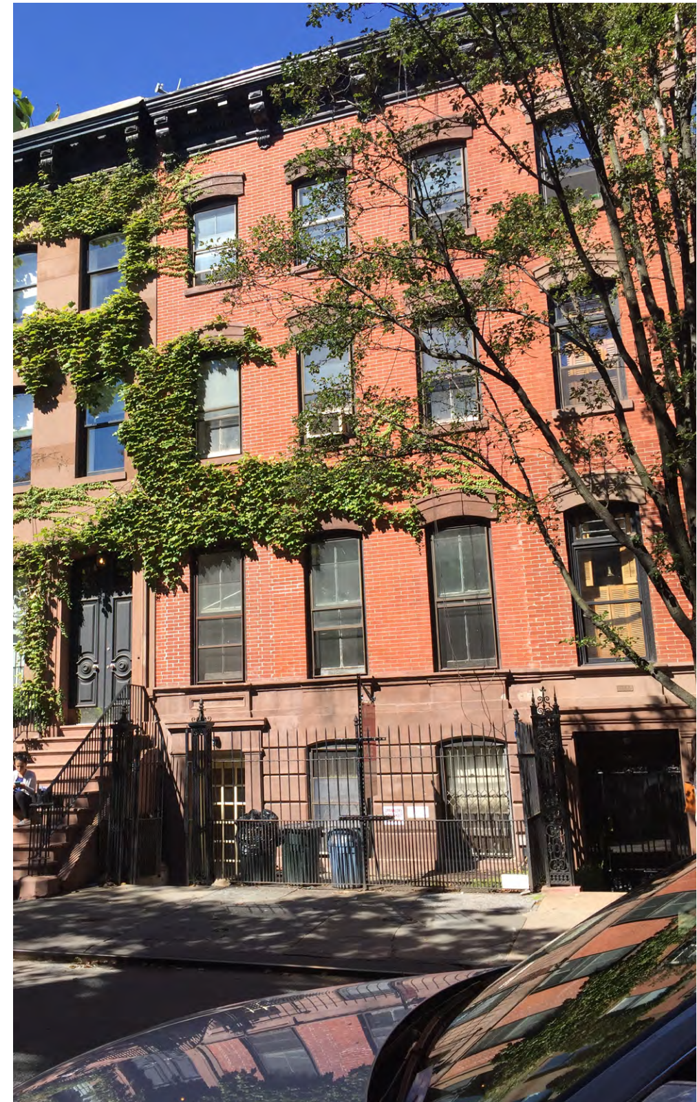
CURRENT FRONT FACADE
