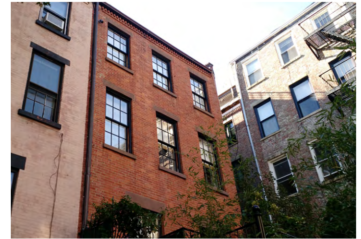
NEIGHBORS ADJACENT REAR FACADES (WEST)
