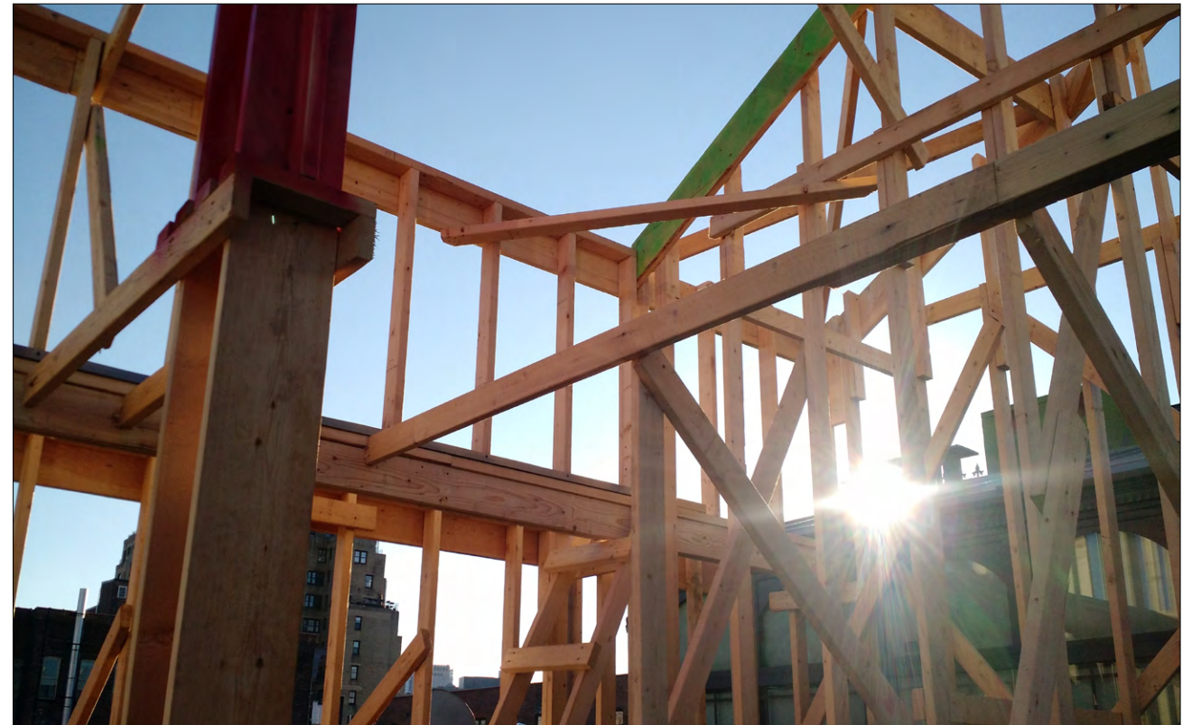
81 CHARLES ST - MOCK UP - ROOF VIEW 2 (LOOKING SOUTH @ STAIR BULKHEAD + RAILING)
