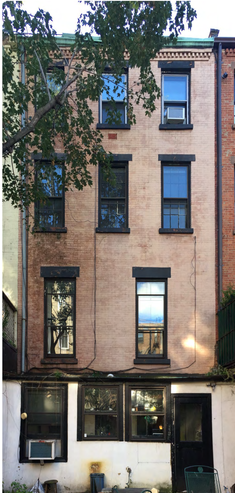
EXISTING REAR FACADE
